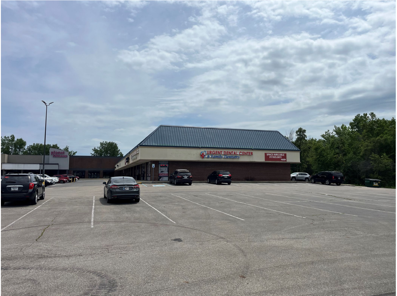
Photo 2: View of some of the tenant spaces on Lot A
