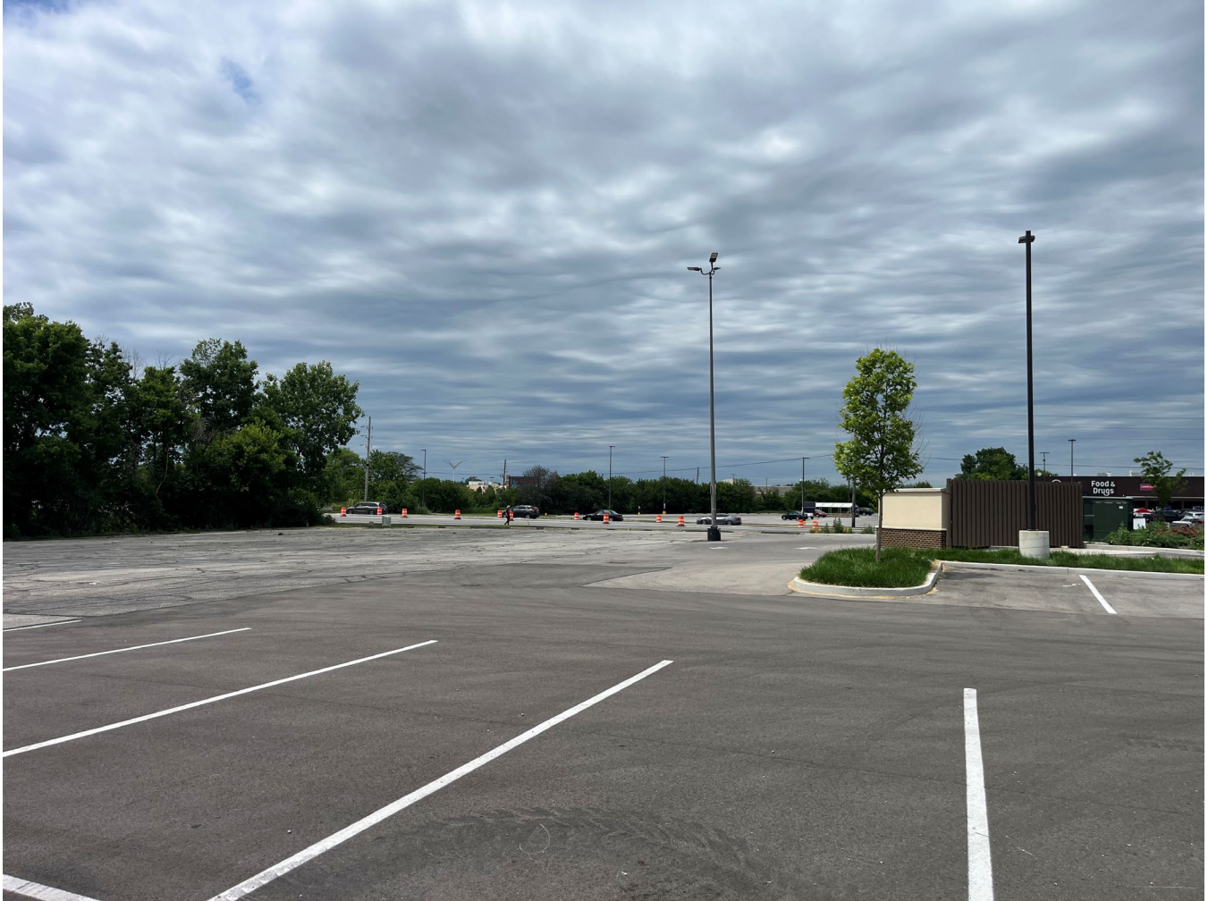
Photo 1: View of Lot 2 with Washington Street in background
