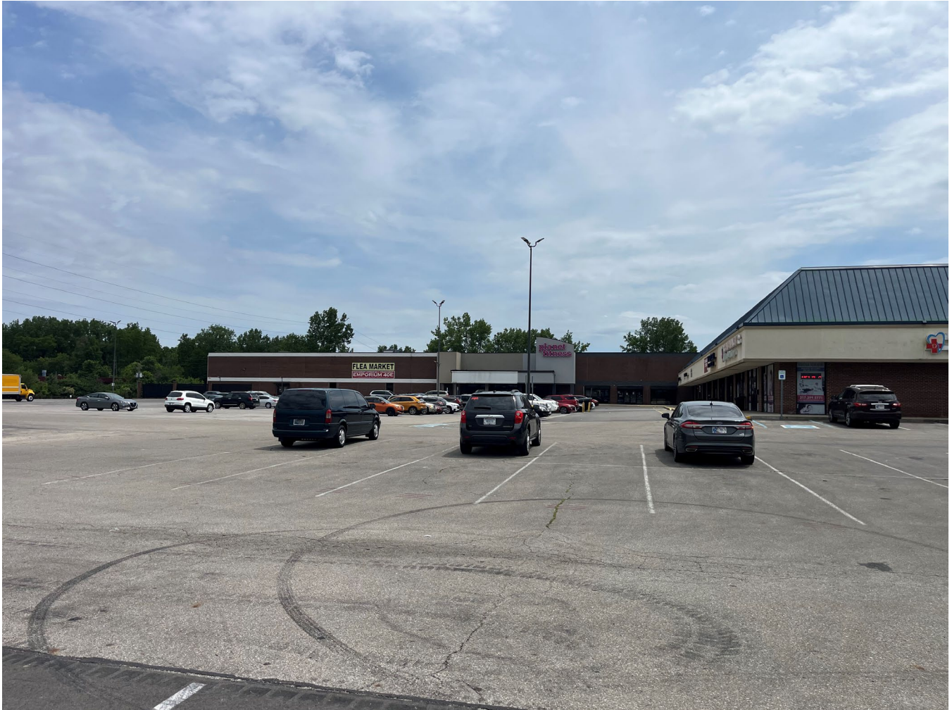
Photo 3: Another view of the tenant spaces on Lot A
