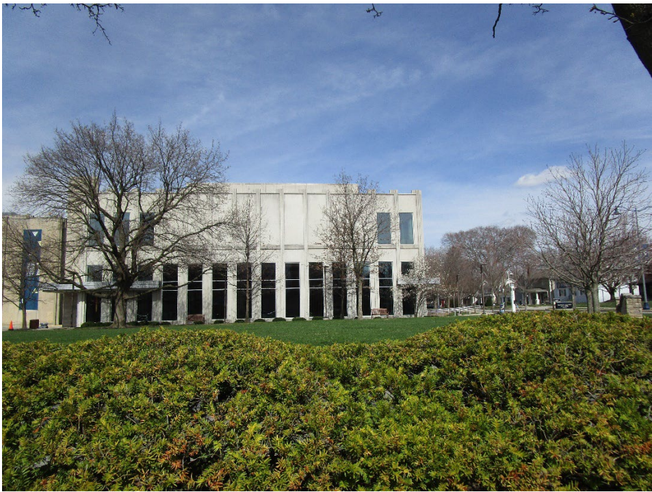
View of Schrott Center for the arts
