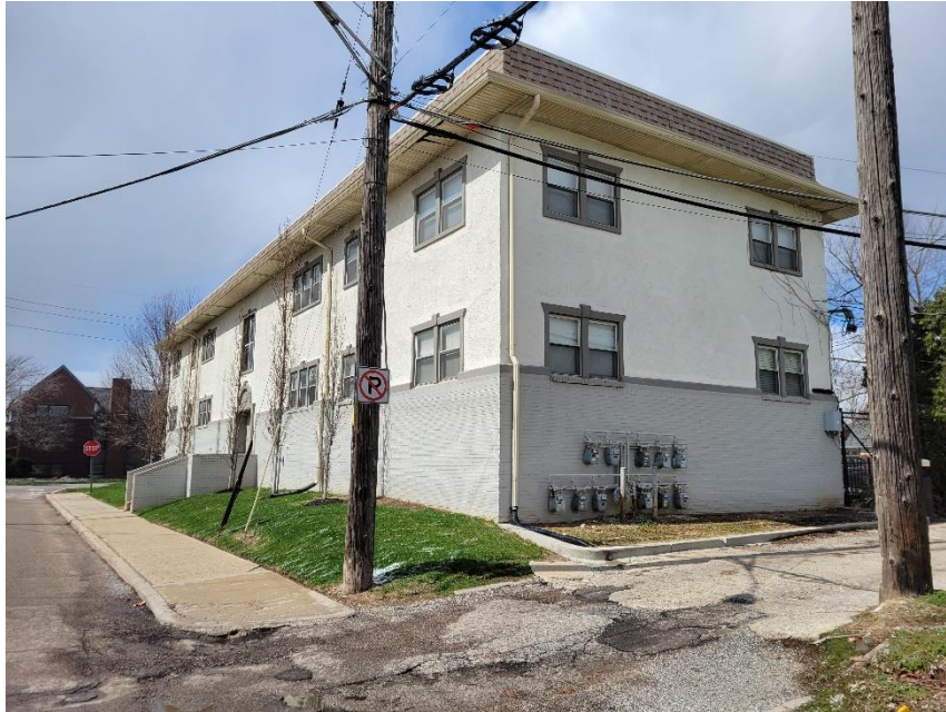
Photo 9: Adjacent Building to West
