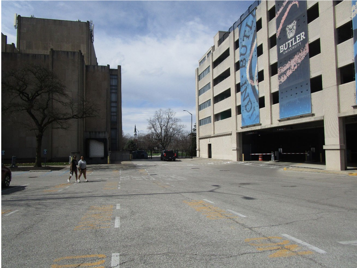
View looking west along the drive – site to the south
