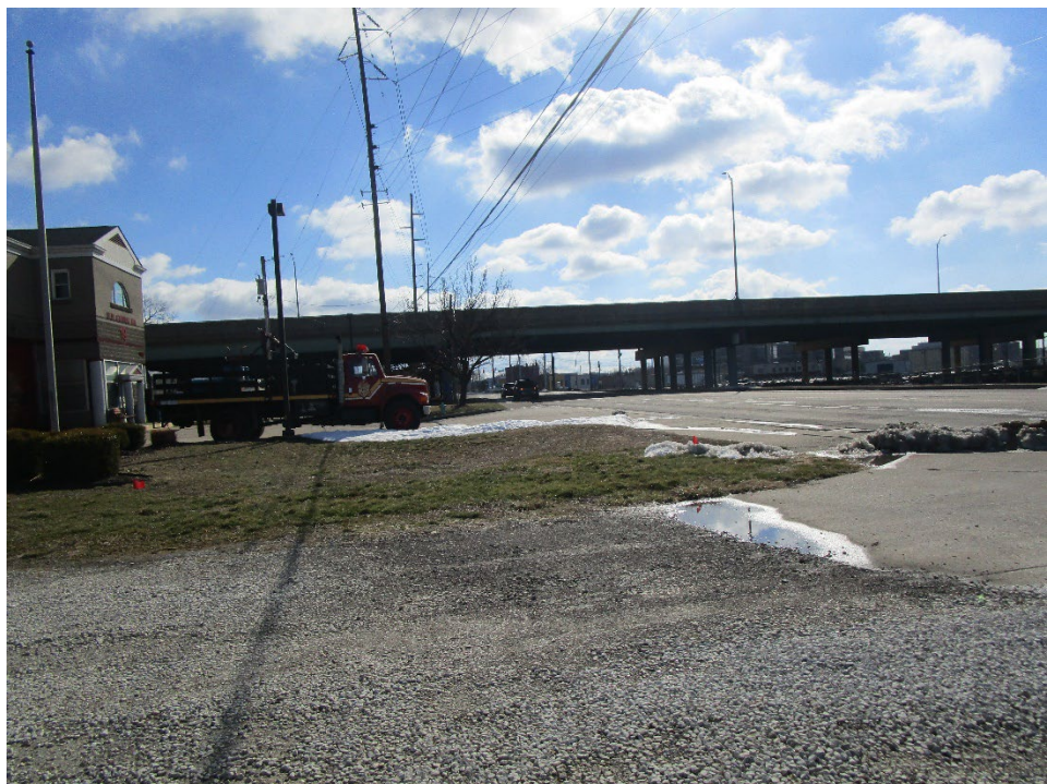
View looking south along South White River Parkway West Drive
