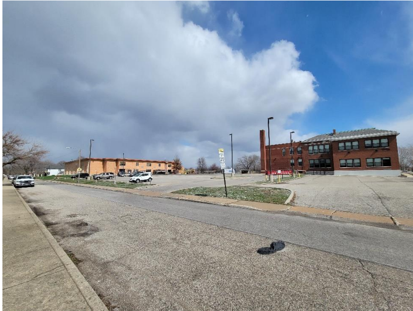
Photo 5: Adjacent Property to East
