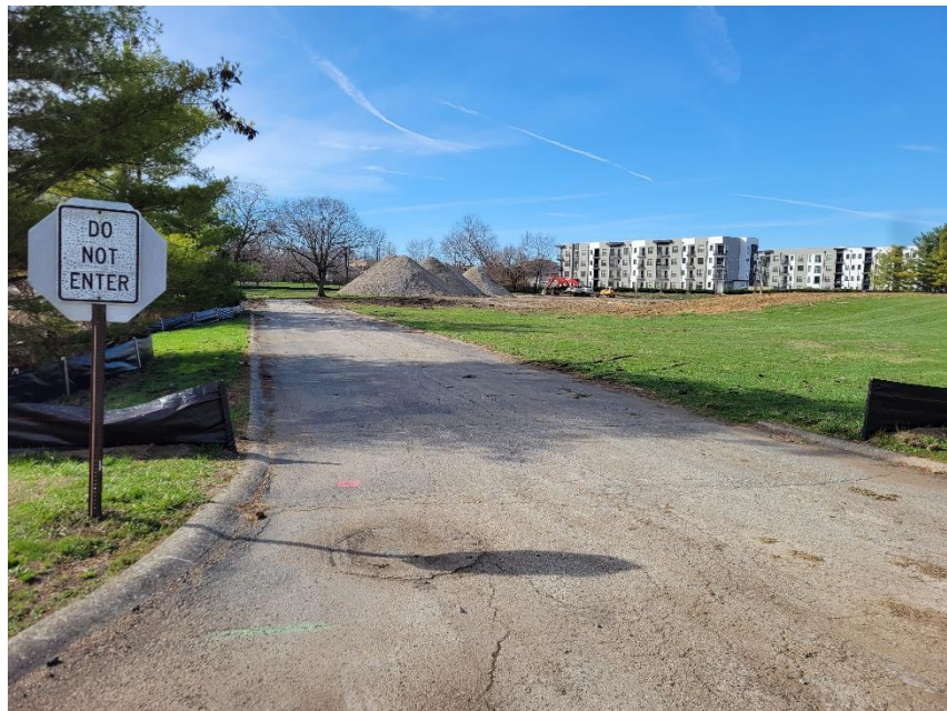
Photo 2: Subject Site Viewed from Southeast
