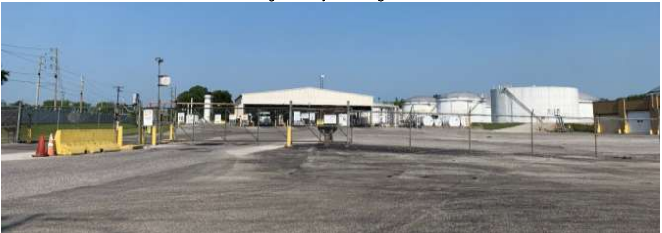
Photo of the gas company northwest of the site.
