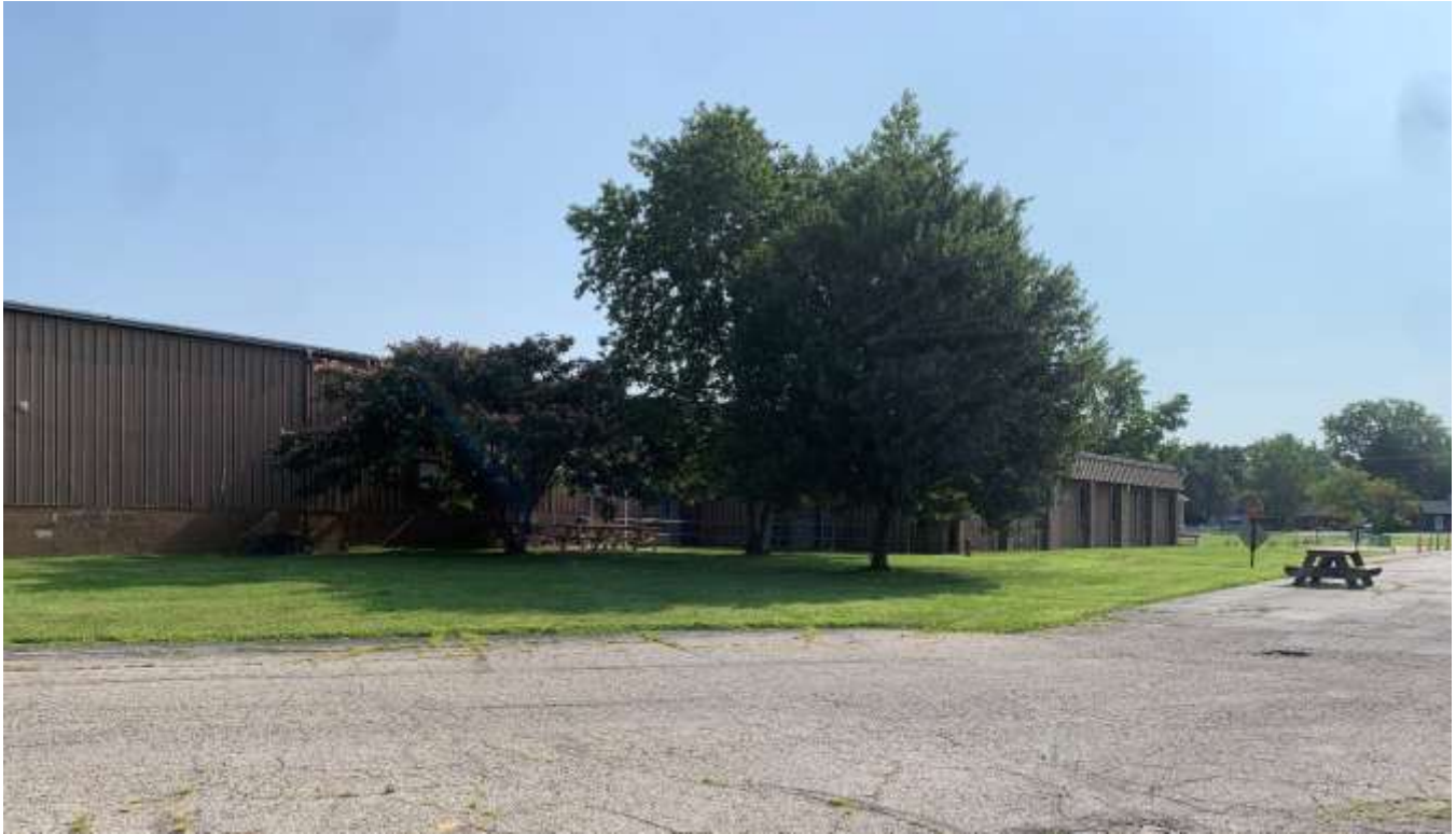
Photo of the existing building looking east.
