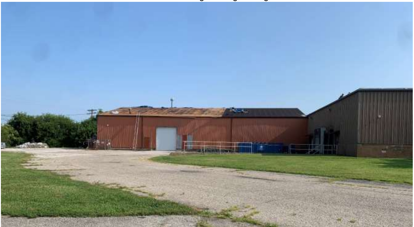
Photo of the existing building looking north.
