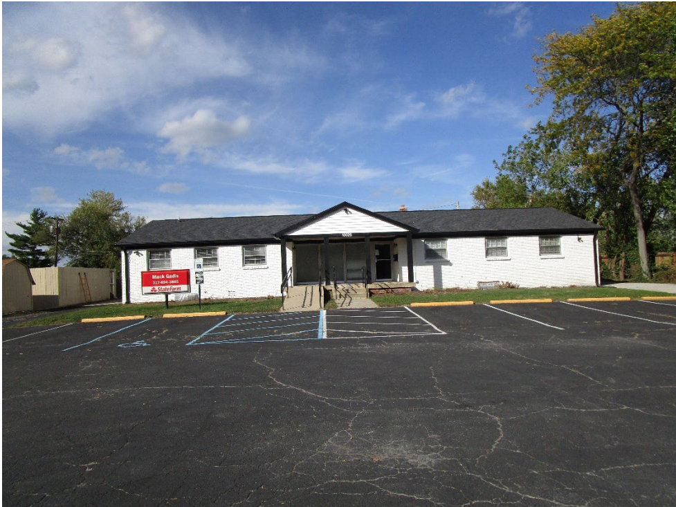
View of site looking north
