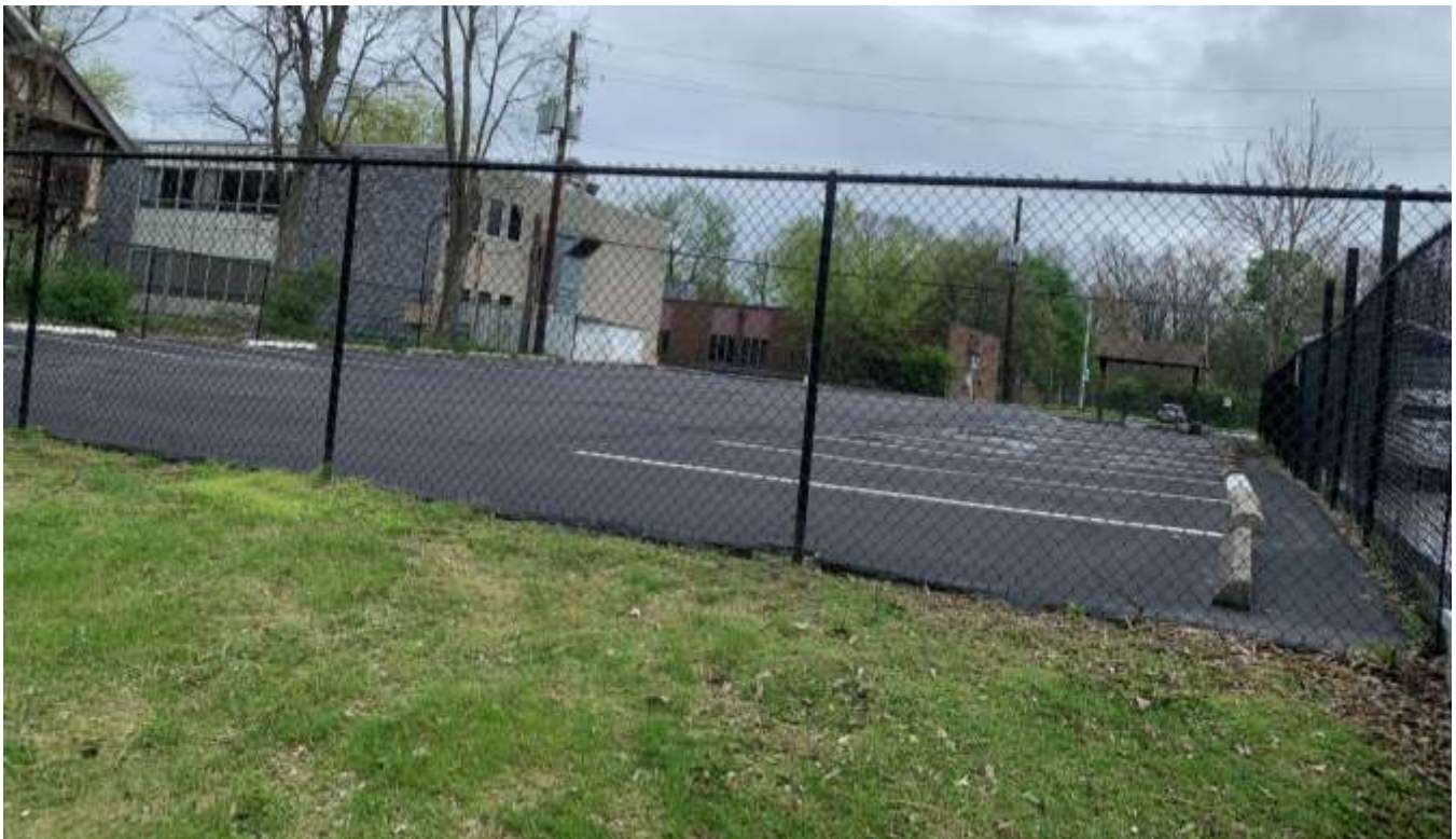
Photo of the rear parking lot on the subject site.
