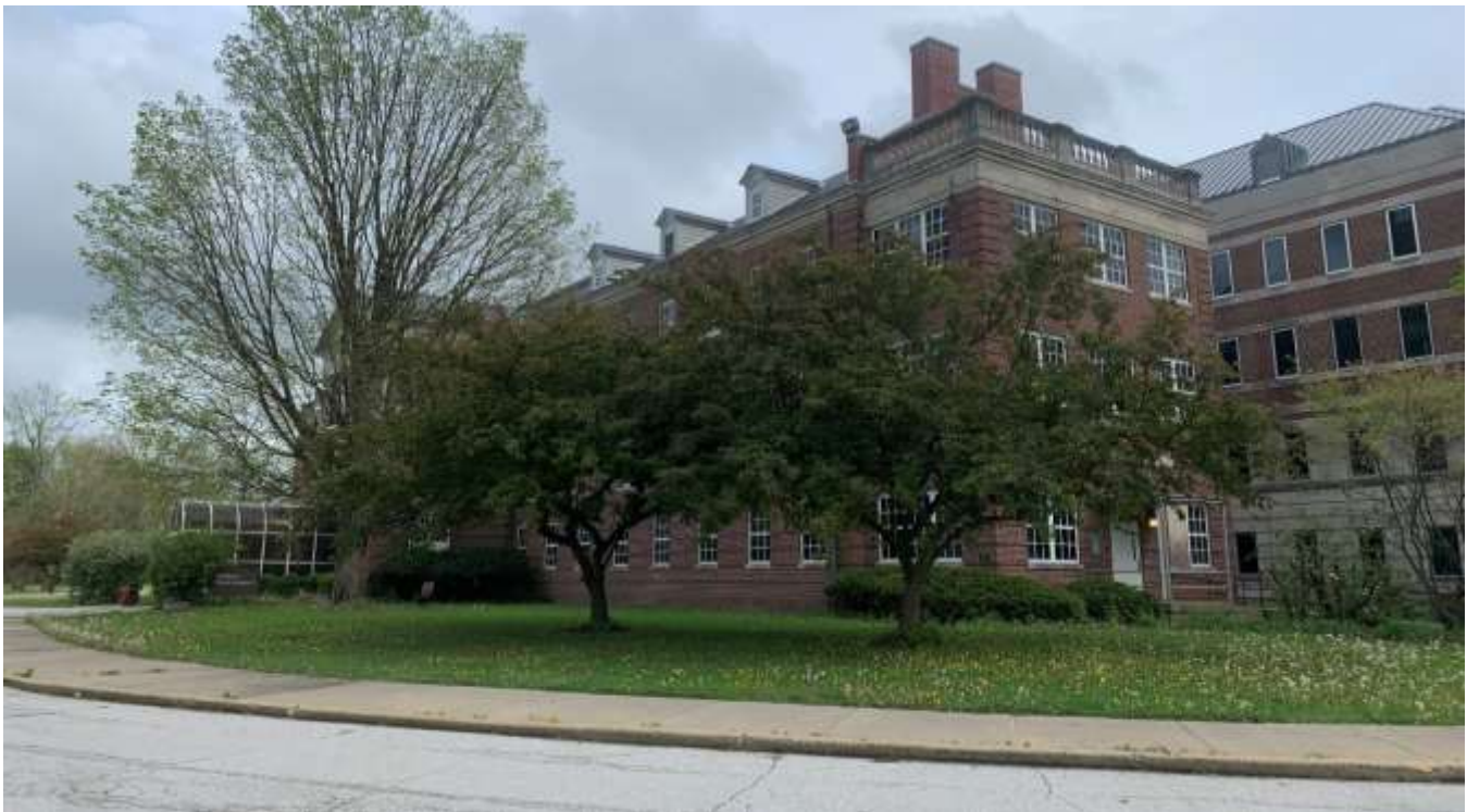
Photo of the northern portion of the building on site.
