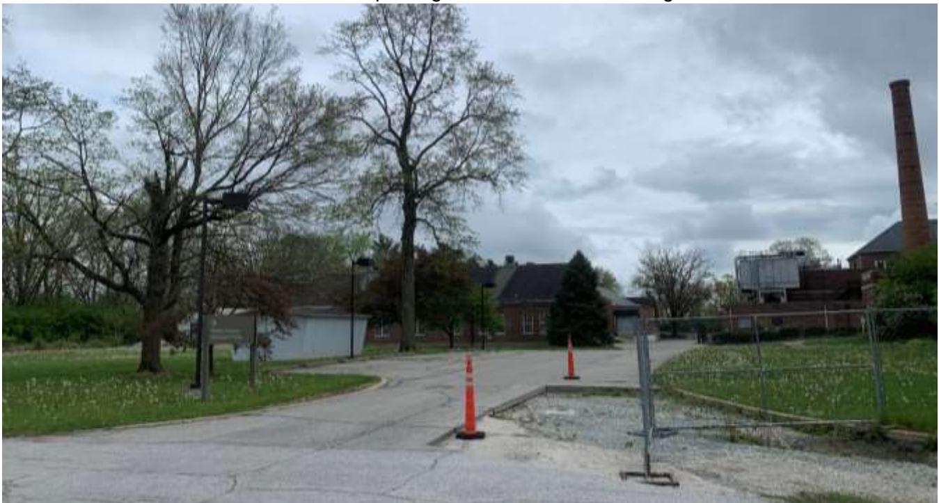
Photo of the rear portion of the property looking south at other buildings on site.
