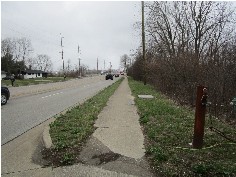
View looking west along East County Line Road
