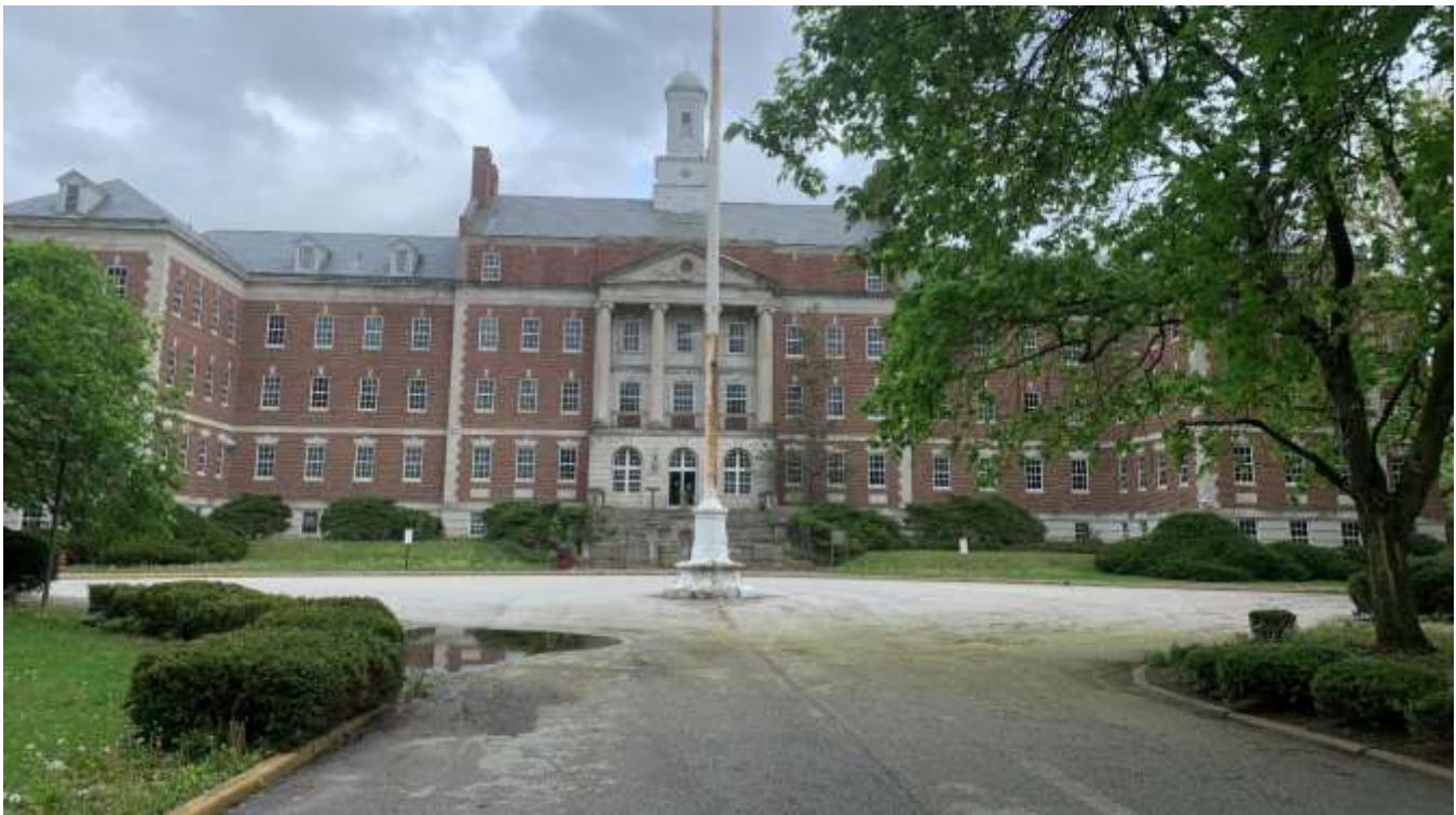
Photo of the building on site looking east.
