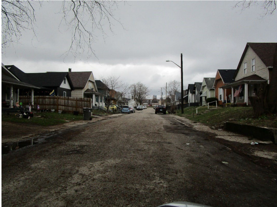
View looking north along South Illinois Street
