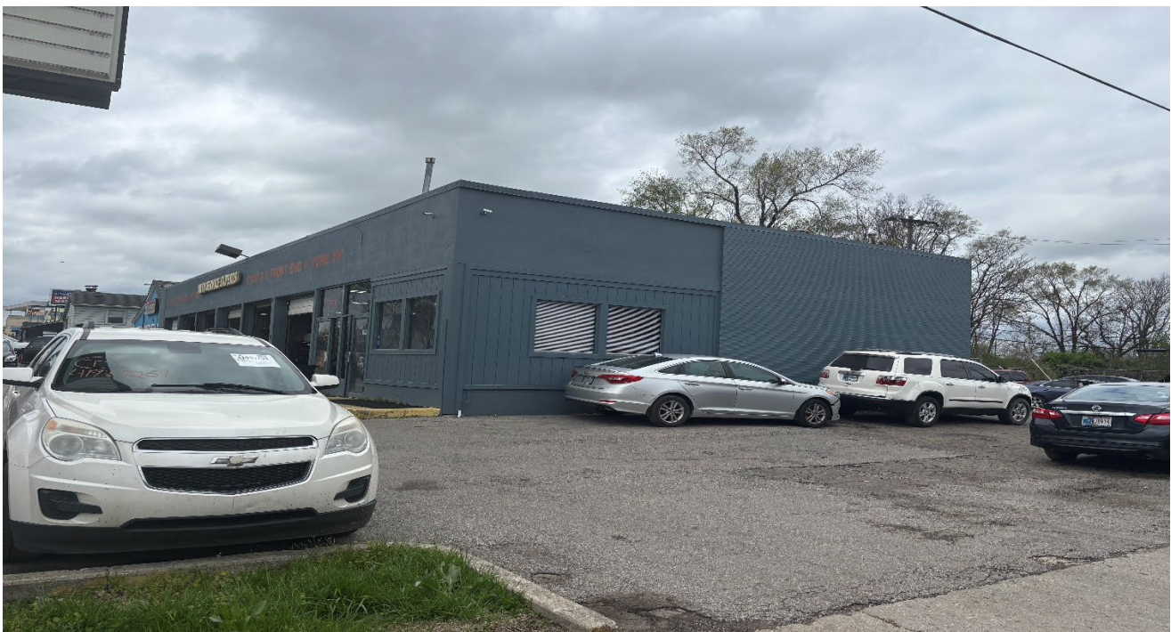
Photo: 5 Looking at the subject property
