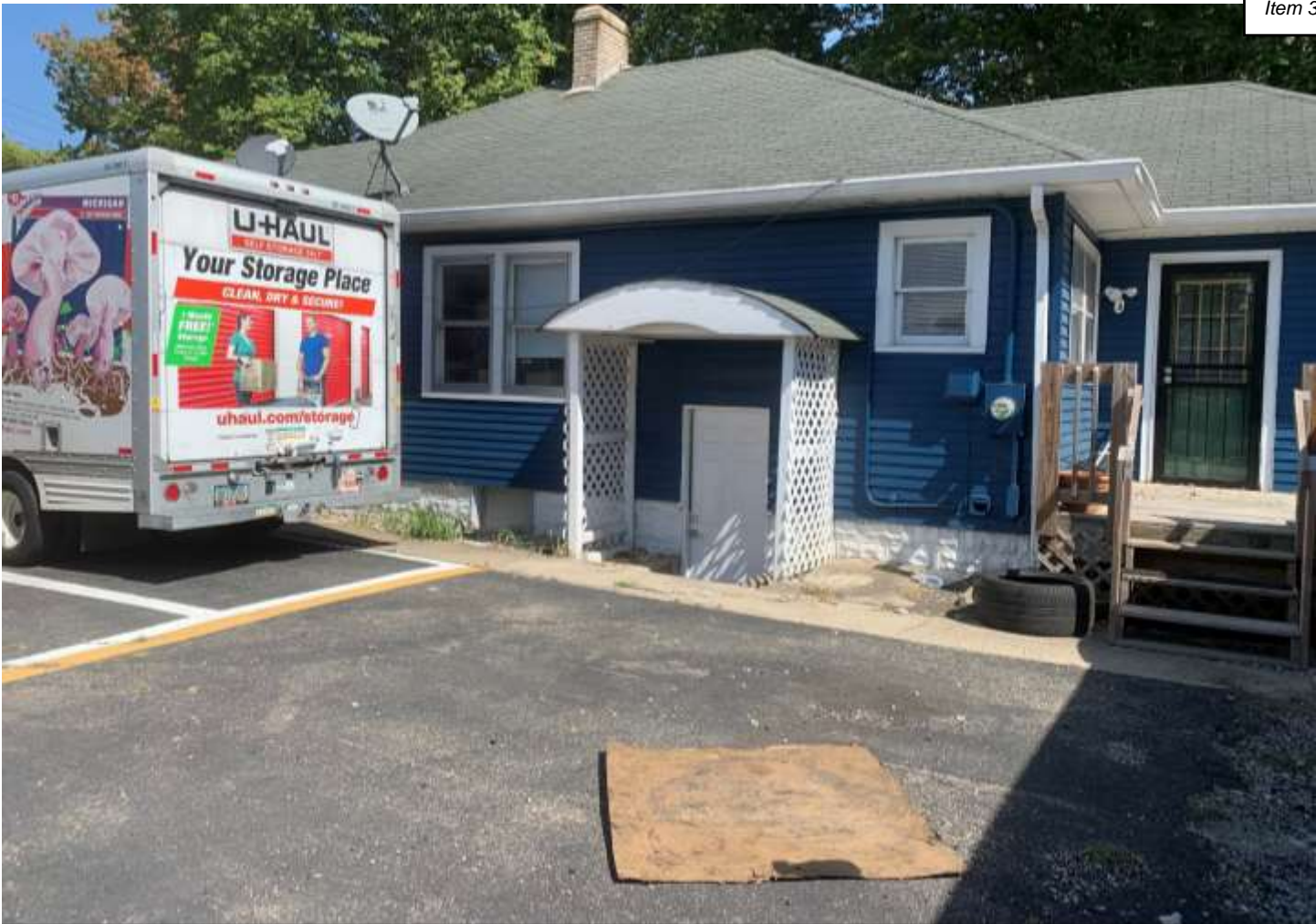
Photo of the western office façade.
