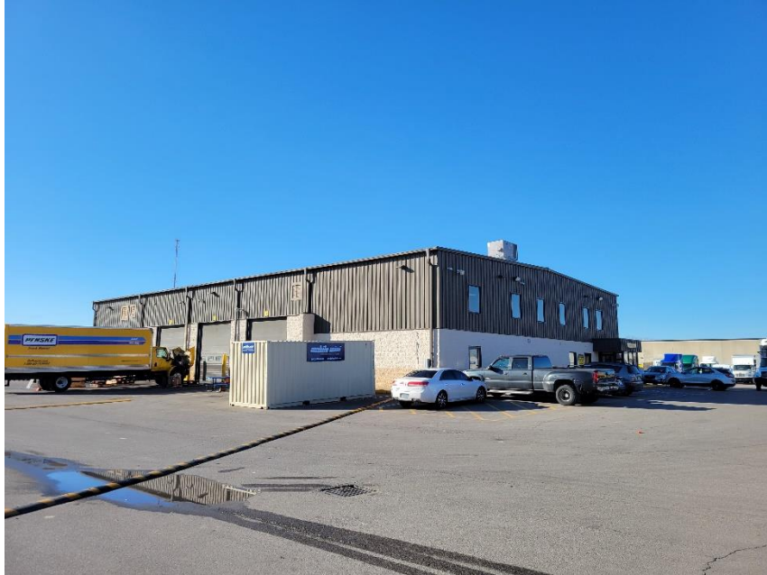
Photo 5: Primary Building Viewed from Northeast
