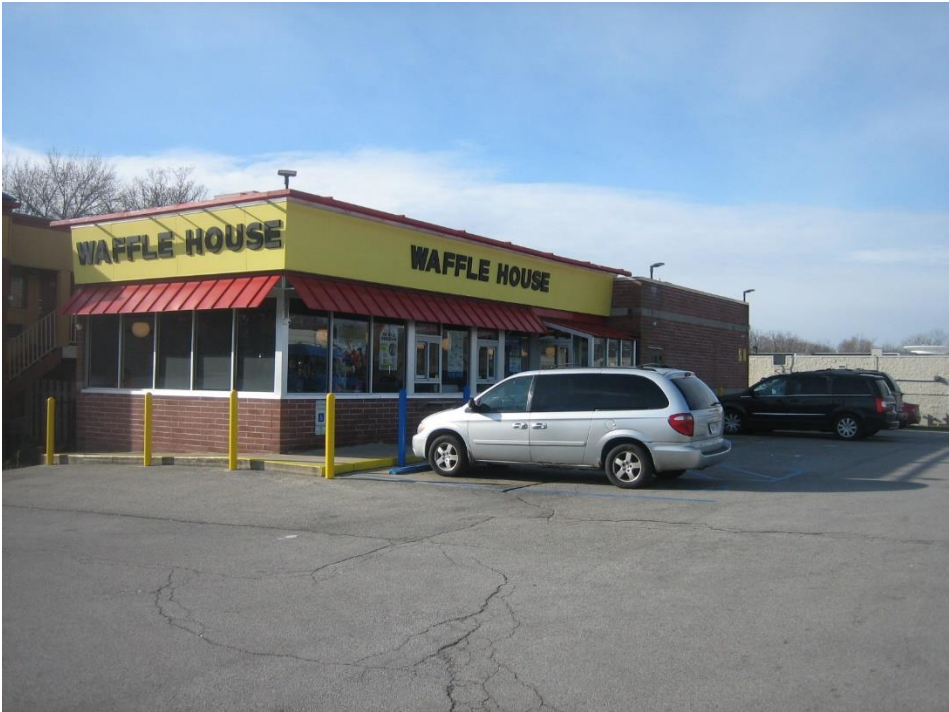
Adjacent Commercial restaurant to the north, looking west.
