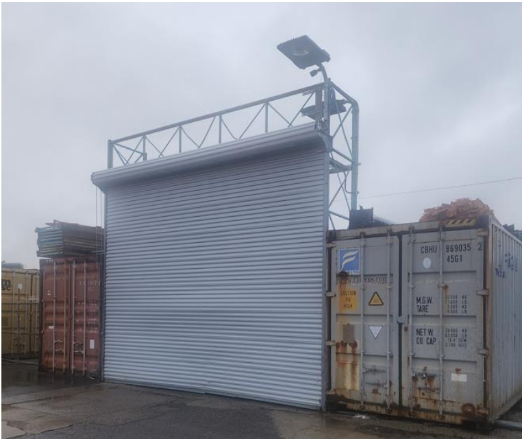
Photo 5: Overhead Garage Door along Southern Elevation (submitted by applicant)
