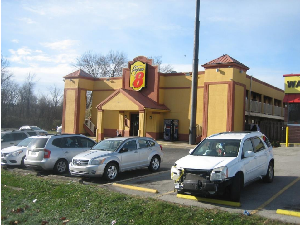
Subject site, east façade, looking west.
