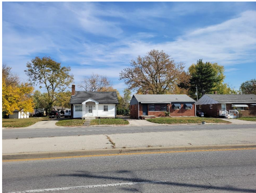
Photo 10: Adjacent Property to East
