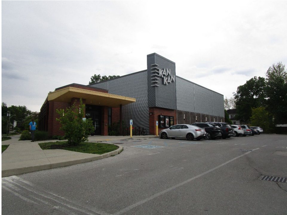
View of site looking southeast
