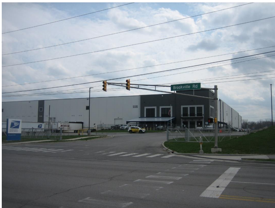
Light industrial warehouse distribution center to the south.
