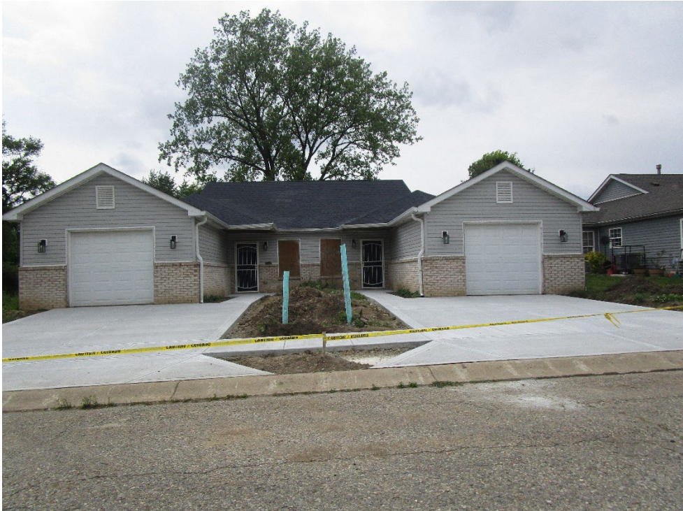
View of site looking west at new development
