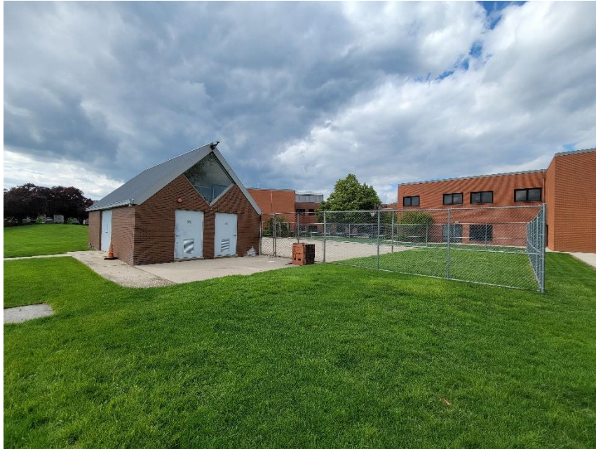
Photo 3: Subject Site Viewed from East
