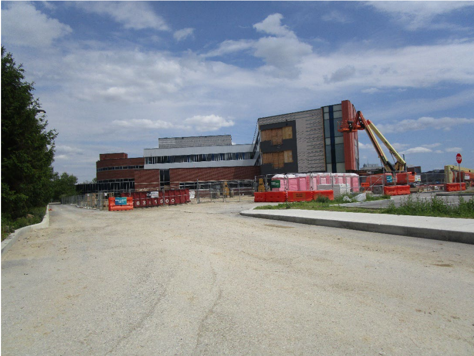
View of site looking east
