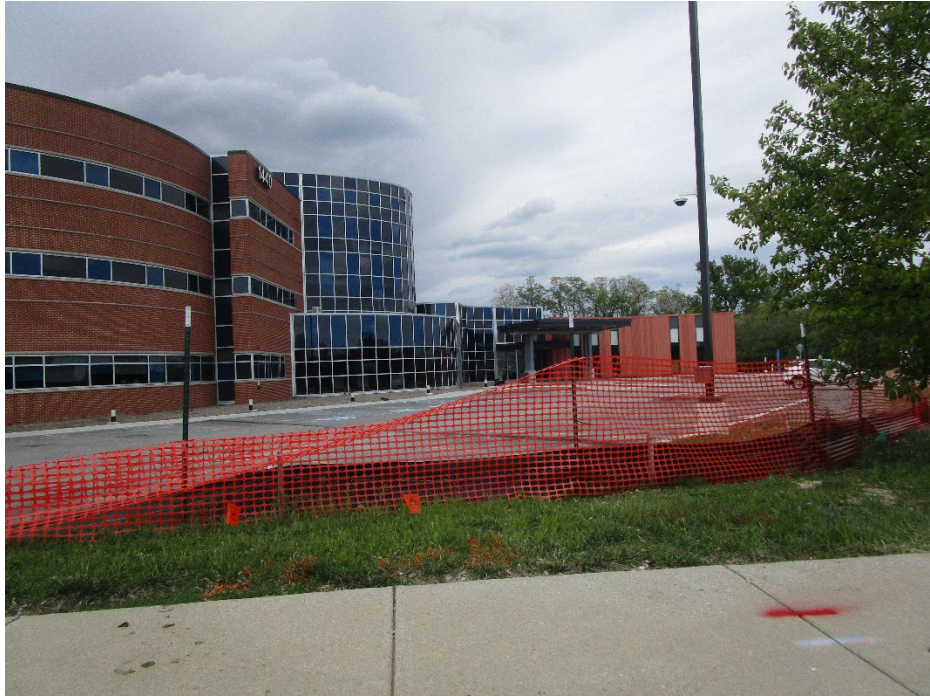
View of site looking east
