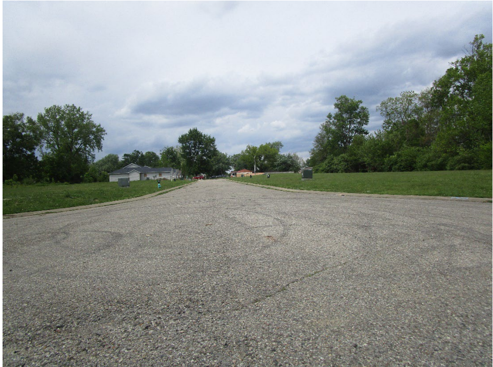
View looking north along Walker Place
