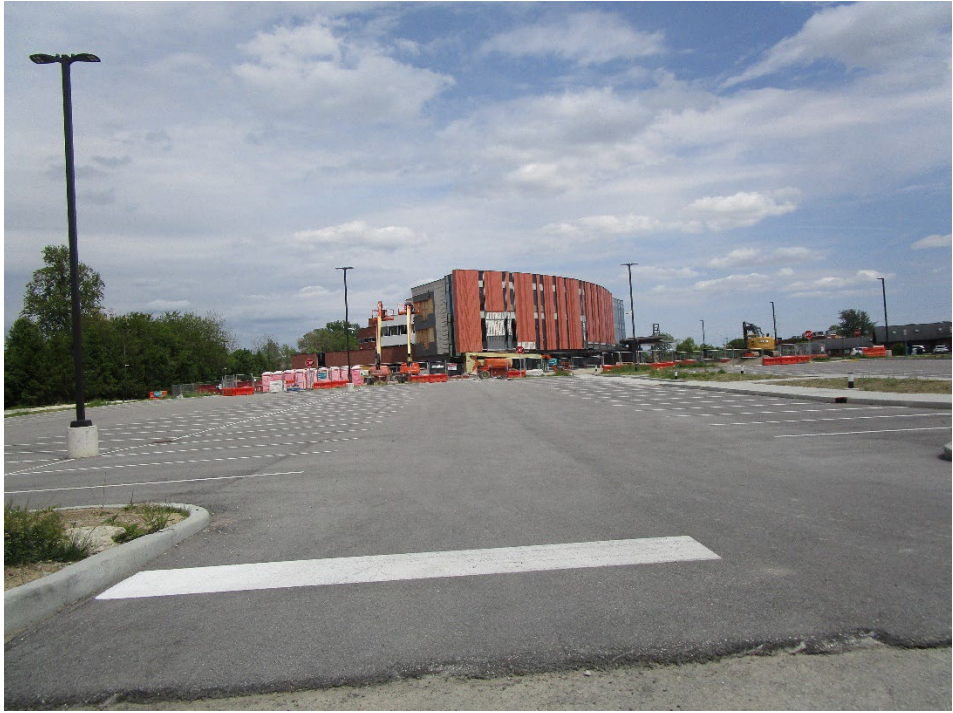
View of site looking northeast
