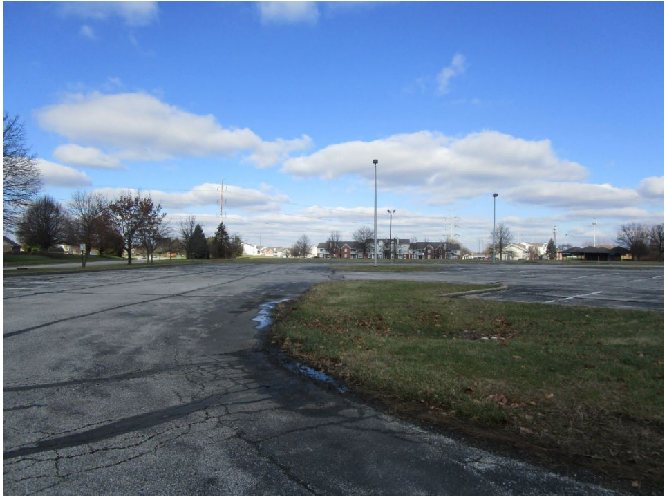
View of site looking north
