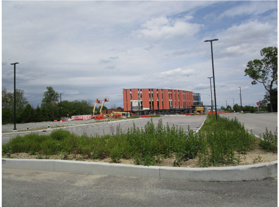
View of site looking east
