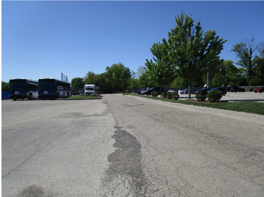
View looking south along recently vacated Evanston Avenue
