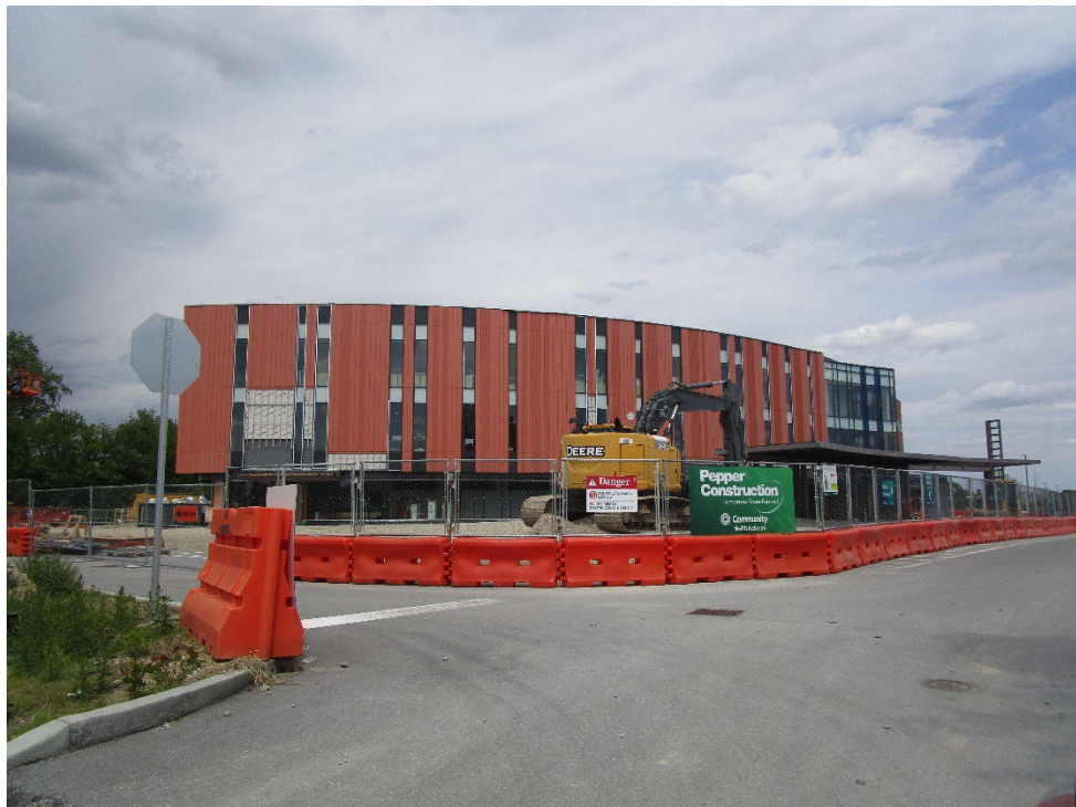
View of site looking northeast
