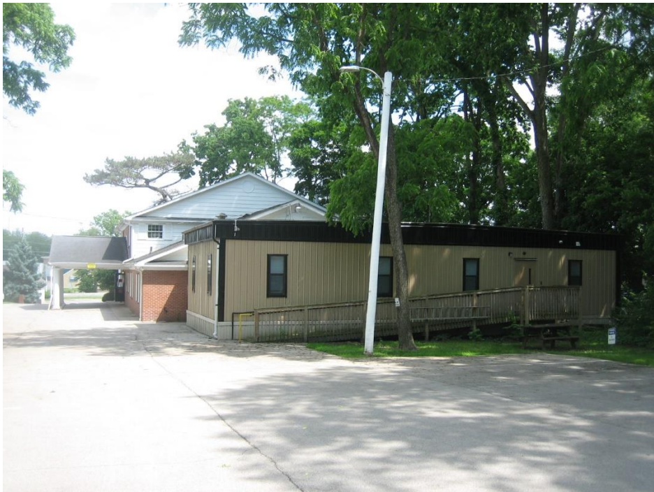
Subject site temporary modular building behind the primary building, looking east.
