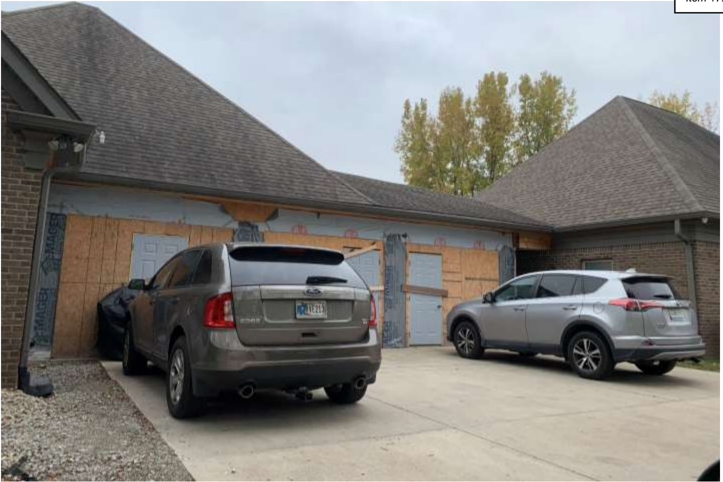
Photo of the northern buiding façade.
