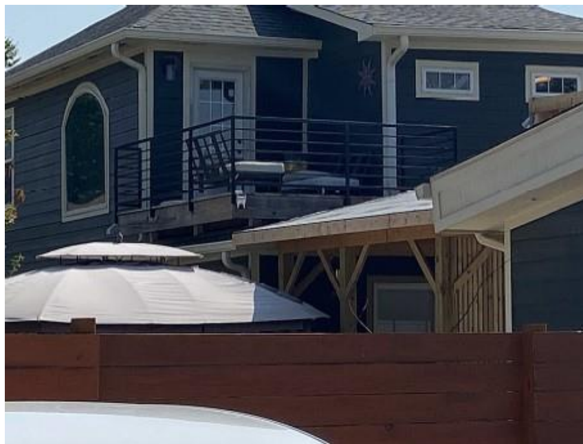
Photo 10: Building Addition Viewed from West
