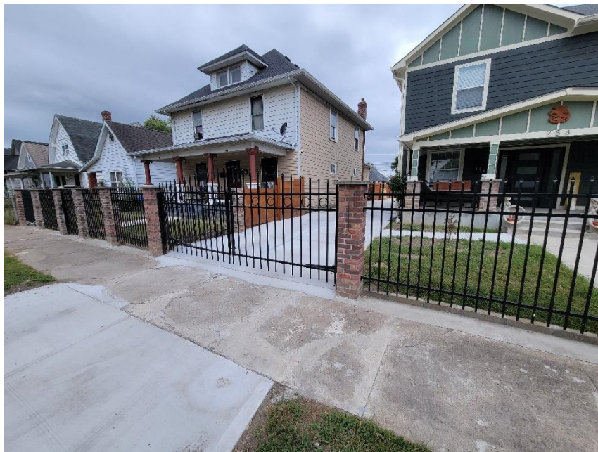
Photo 4: New Driveway on Subject Site Viewed from East
