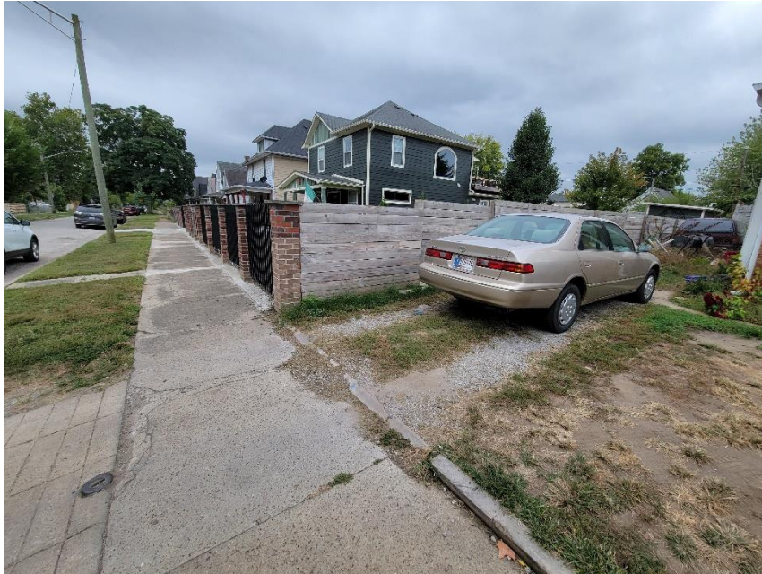
Photo 3: Subject Site and Neighboring Driveway Viewed from East
