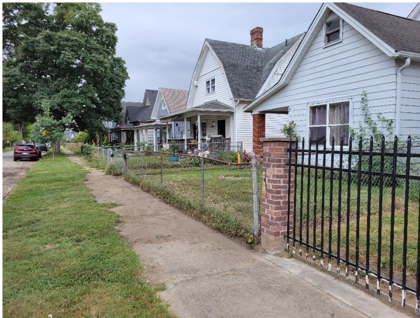
Photo 6: Adjacent Property to South
