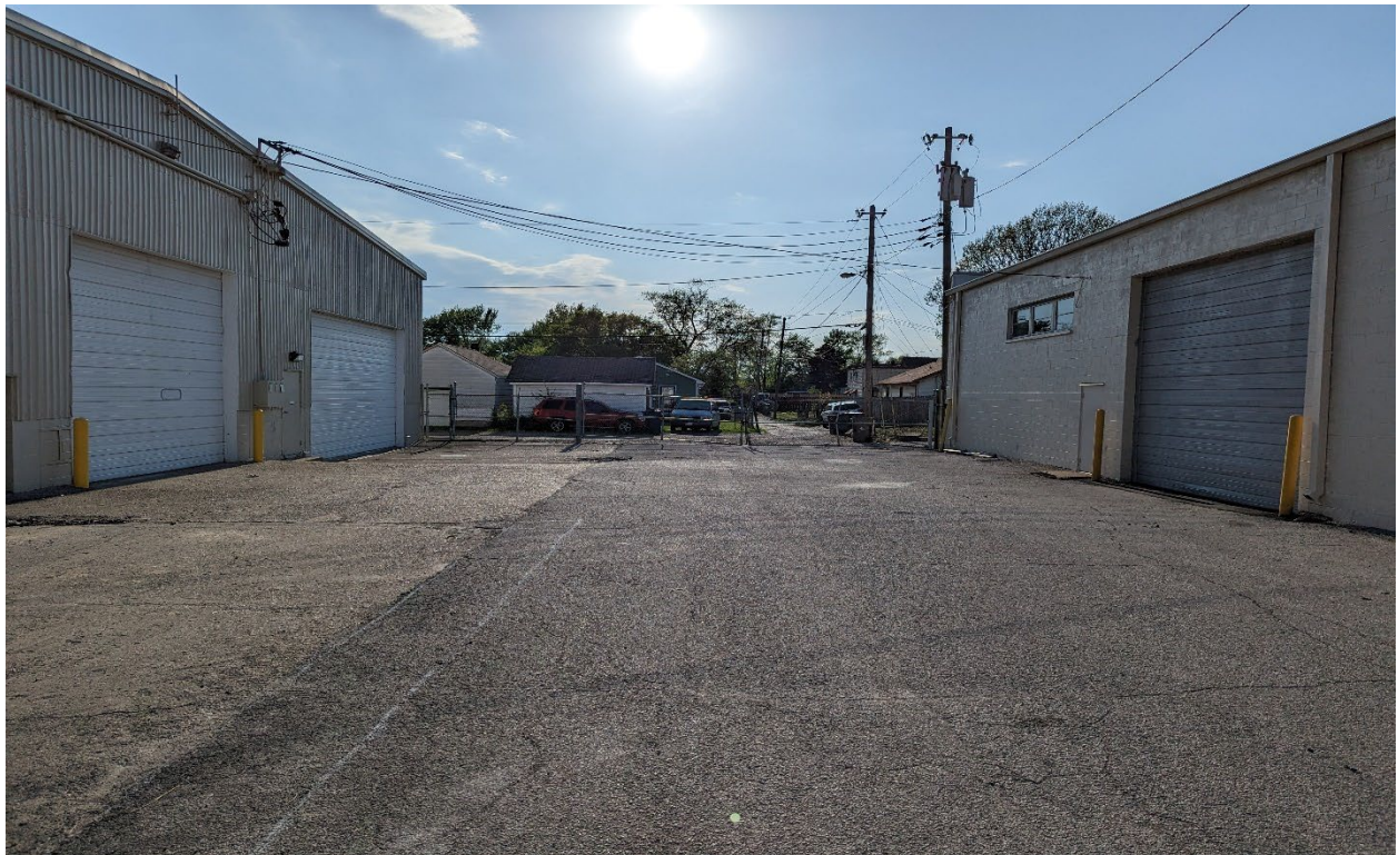
Photo Four: Internal to site. Subject building and overhead door on the right
