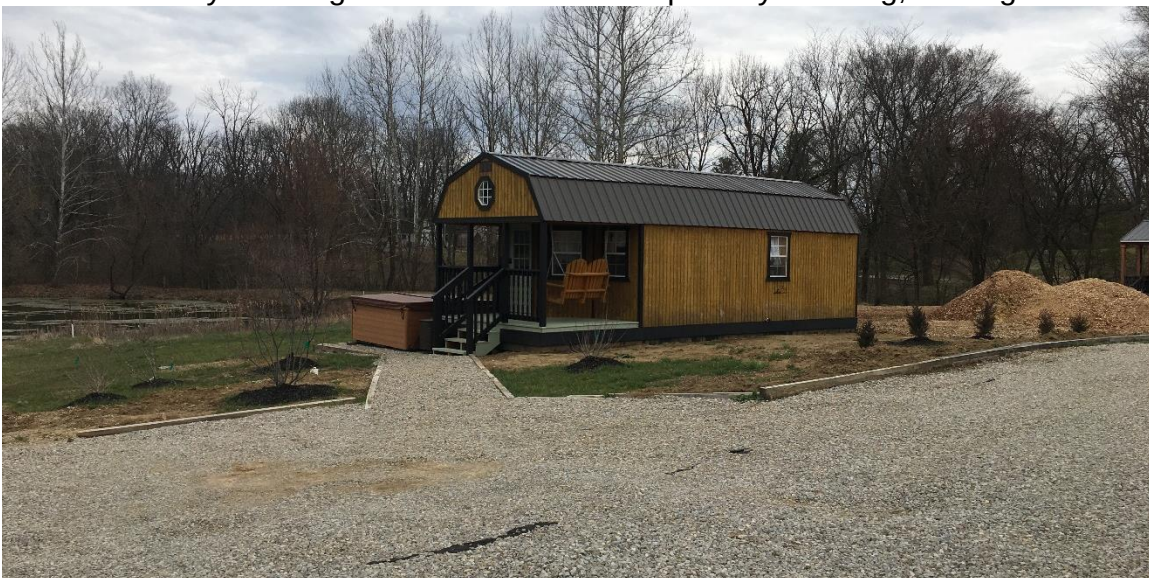
Secondary dwelling cabin, looking east
