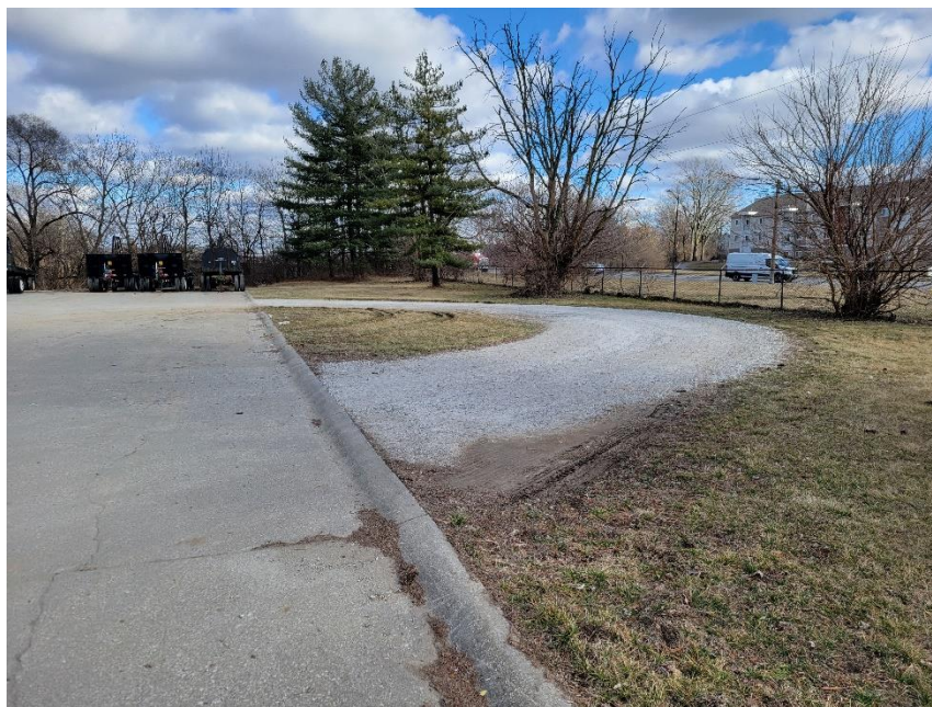
Photo 2: Horseshoe Gravel Area For Truck Maneuvering (Installed 2021)
