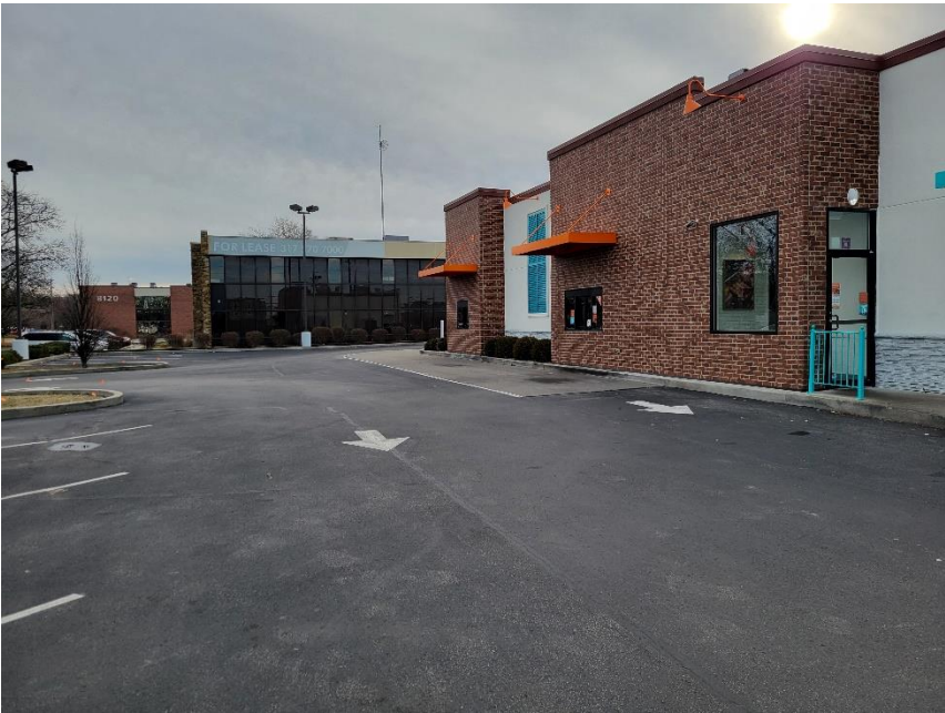
Photo 2: Drive-Thru in Front Yard Viewed from North
