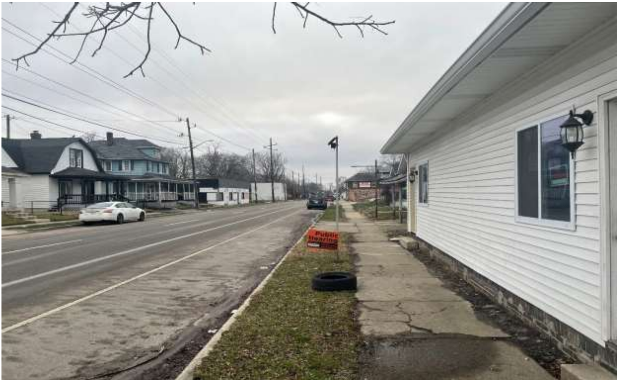
Photo Two: Looking West Along Michigan Street – Subject Site On Right
