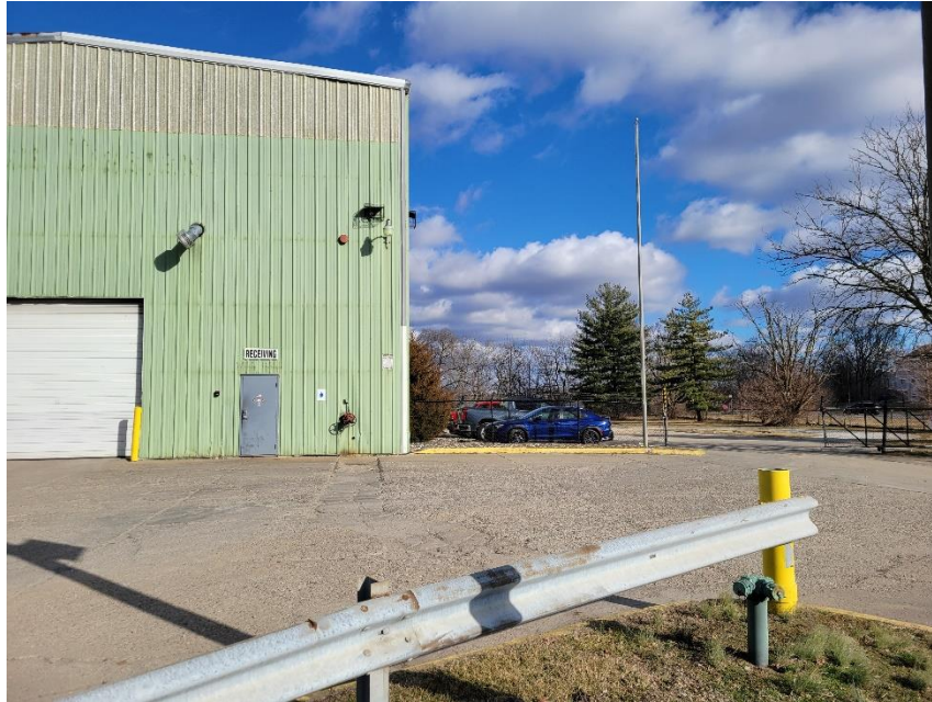
Photo 5: Truck Entrance Area & Partial Western Elevation
