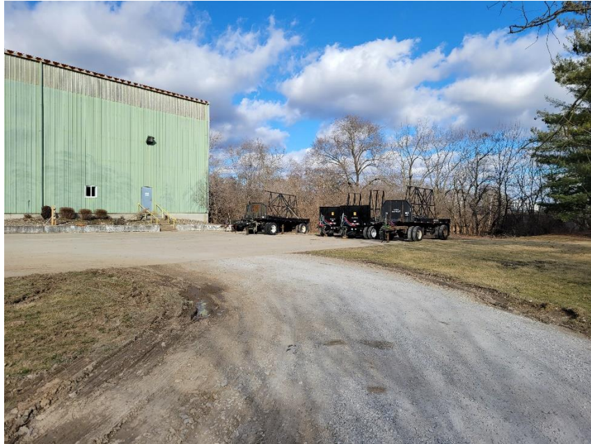
Photo 3: Partial Southern Elevation & Loading/Storage Area
