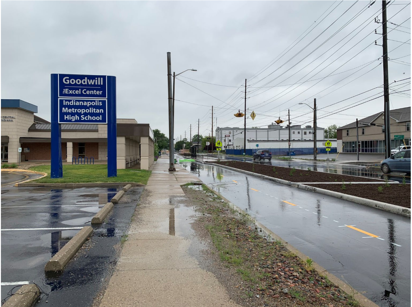
View of the existing pylon sign, bus stop, bike lane, landscape buffer zone and the two travel lanes of Michigan Street, looking west
