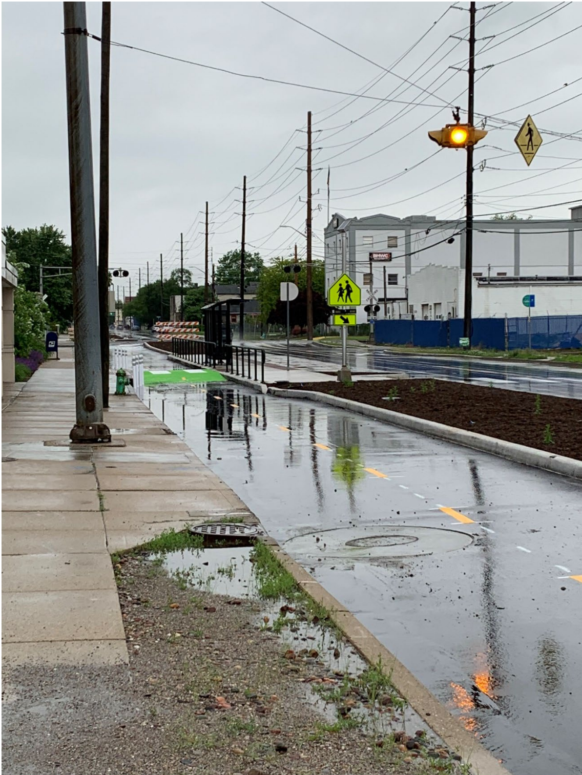
Close-up view of bus stop, bike lane, landscape buffer zone and the two travel lanes of Michigan Street, looking west
