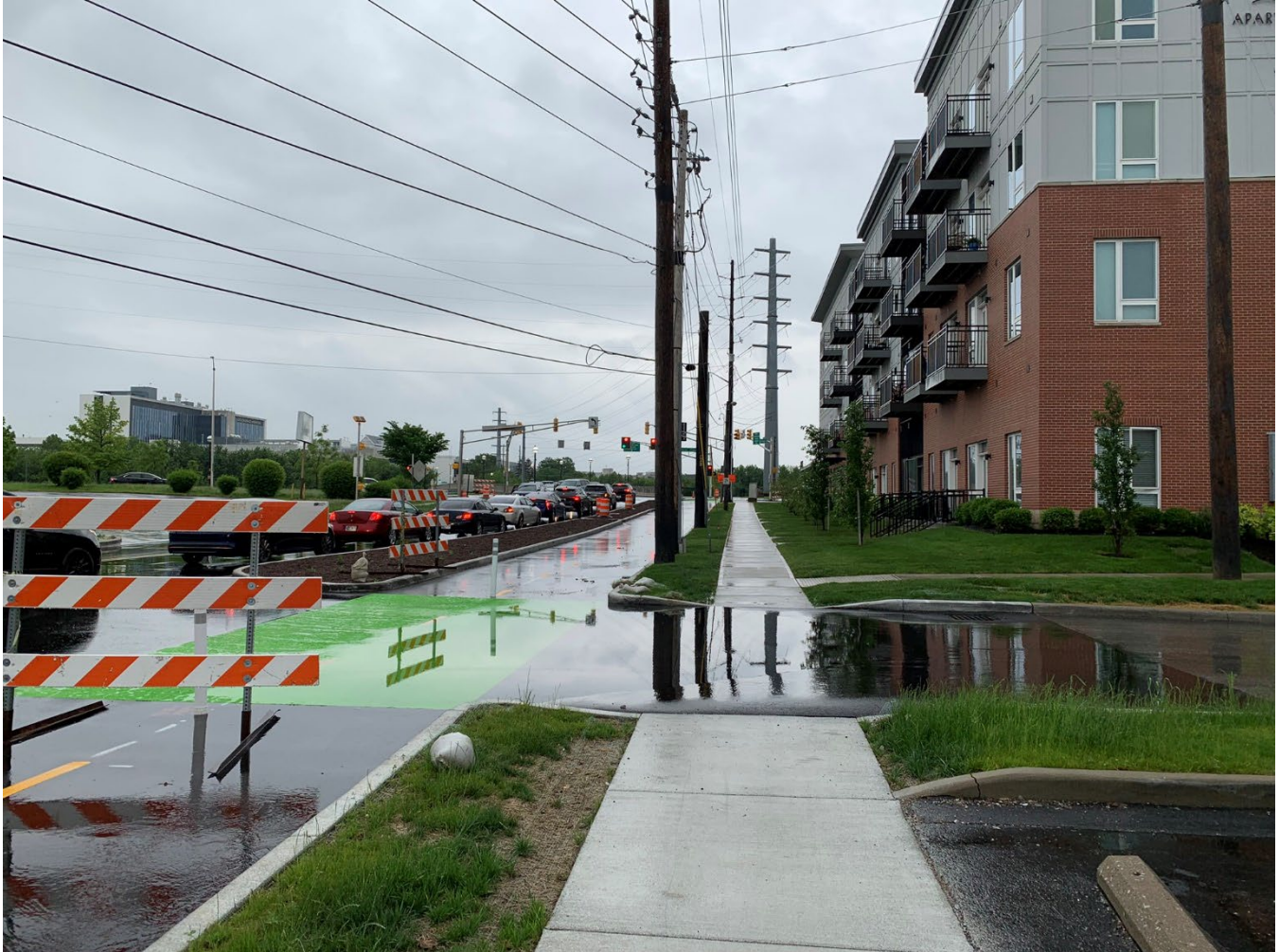
View of Michigan Street bike lane and landscape buffer zone (newly installed) and multi-family dwellings east of subject site, looking east
