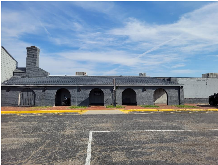
Photo 2: Subject Site from West (southern portion)
