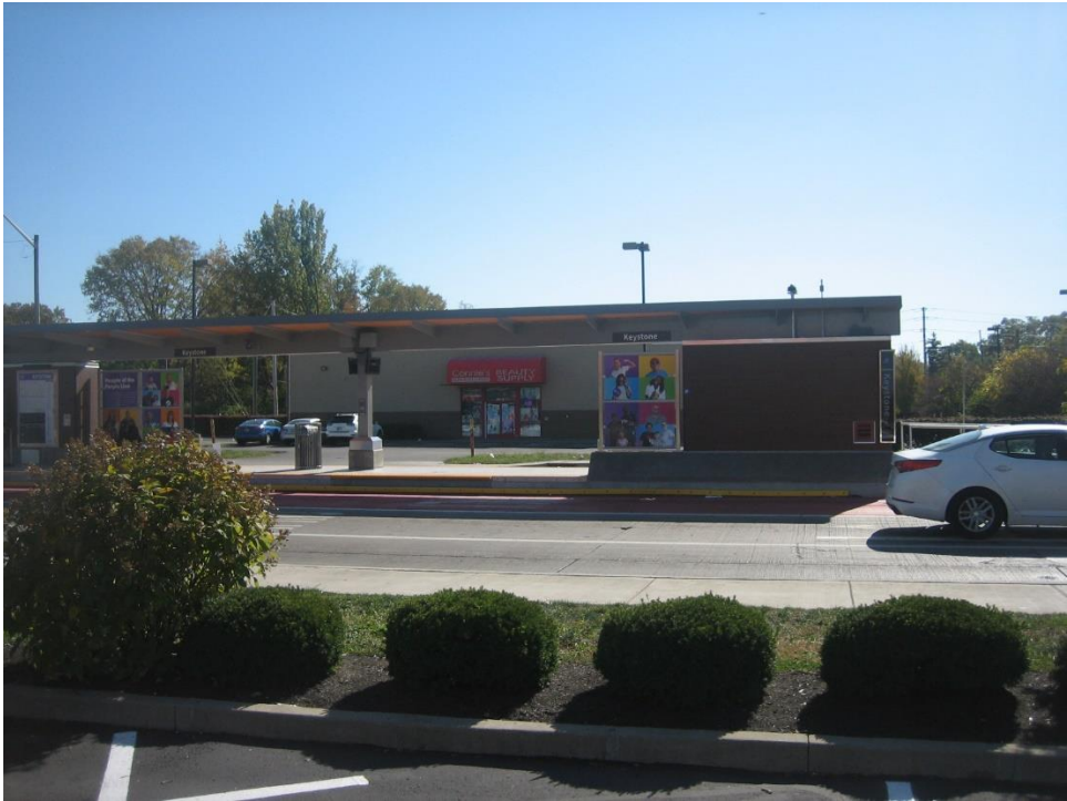
Adjacent Purple line transit stop, to the south
