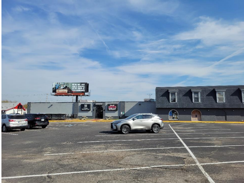
Photo 1: Subject Site from West (northern portion)
