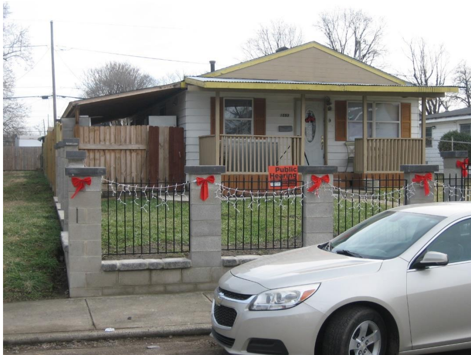
Photo 2- Subject property attached covered porch with zero-foot north side yard setback, looking east.
