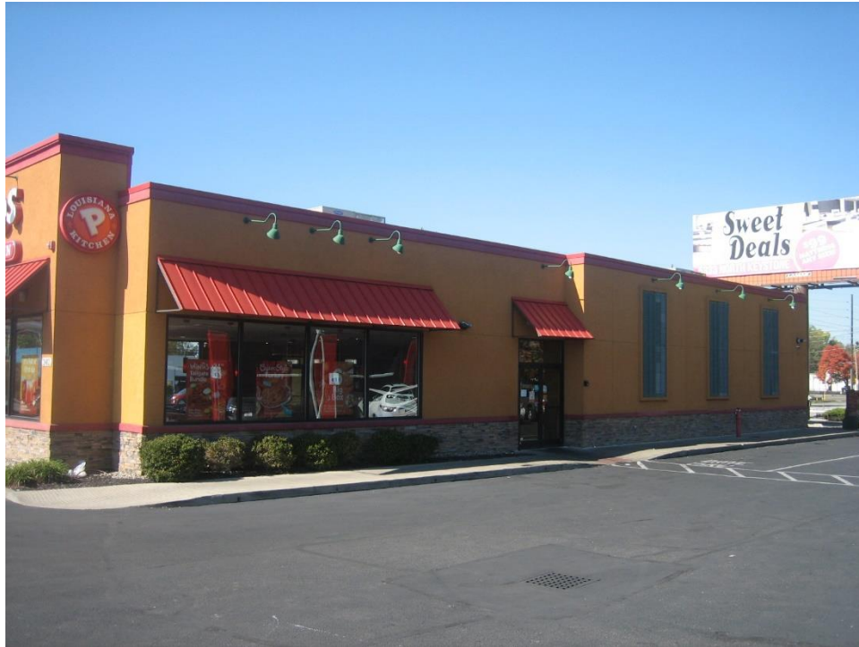
Subject site, east façade, looking northwest.
