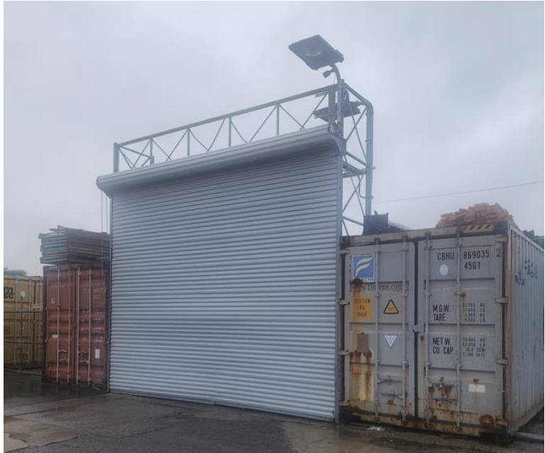
Photo 5: Overhead Garage Door along Southern Elevation (submitted by applicant)
