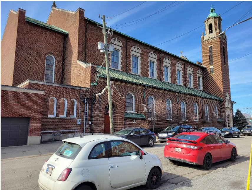
Photo 10: Adjacent Property to South
