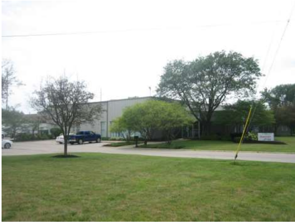
Adjacent industrial property to the west.
