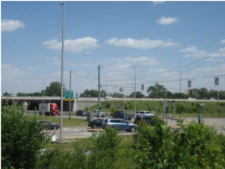
Adjacent I-465 interstate interchange, looking east.
