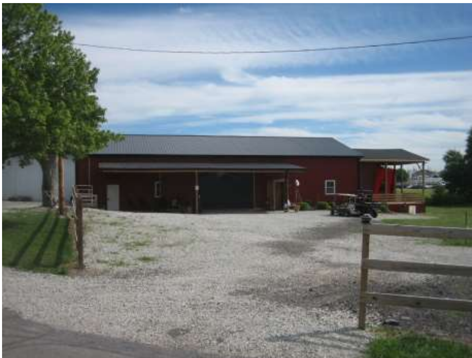
Subject site event center, looking south
