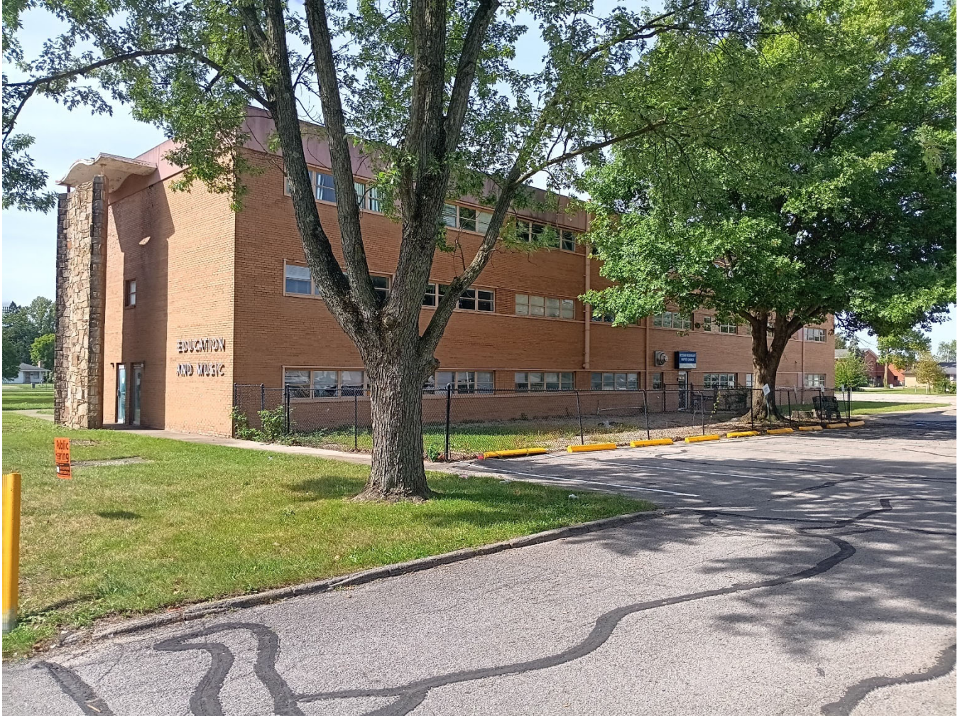
Exhibit 5: North right-side where vocational beauty school and dedicated parking spots will be located, facing southwest.
