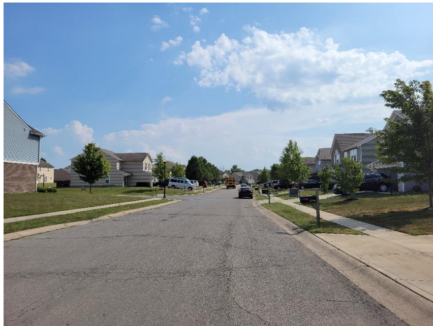
Photo 4: Adjacent Property to South
