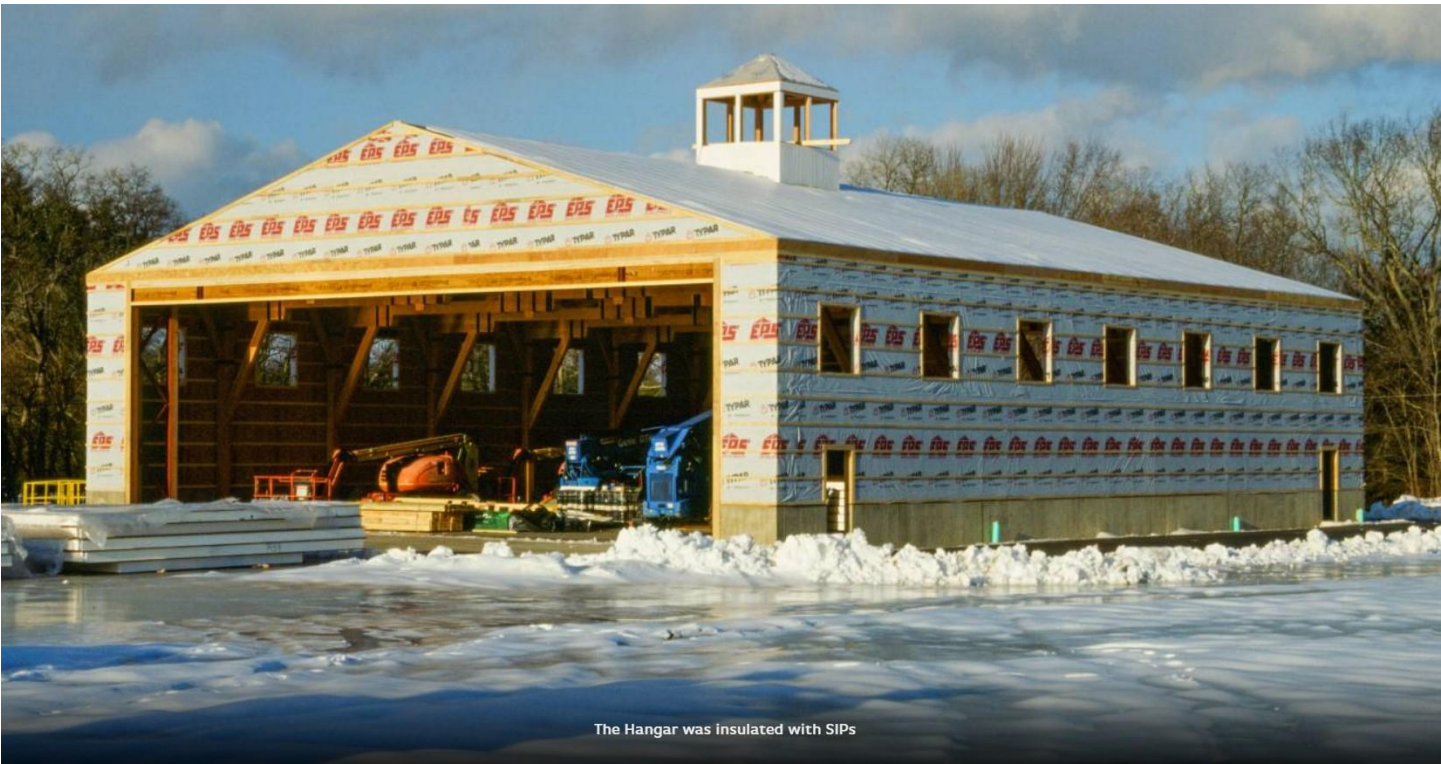
The finished frame with roof decking
