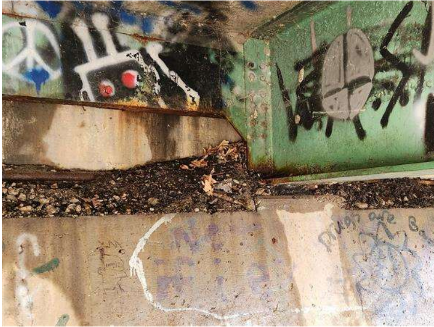
Photo Number: 15 Photo Taken: 12/29/2023 Heavy buildup of road debris around abutment beam bearings (typical of both sides)
