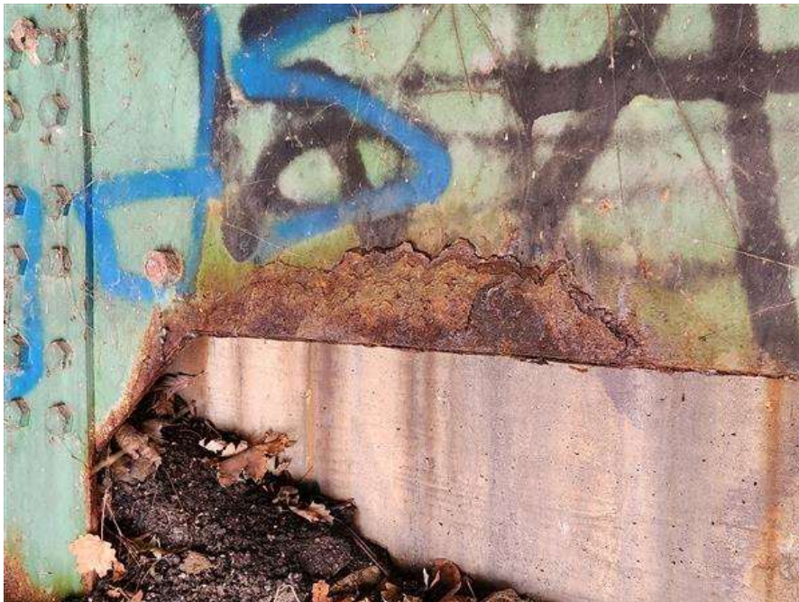
Photo Number: 16 Photo Taken: 12/29/2023 Steel corrosion with delaminations on West abutment diaphragms
