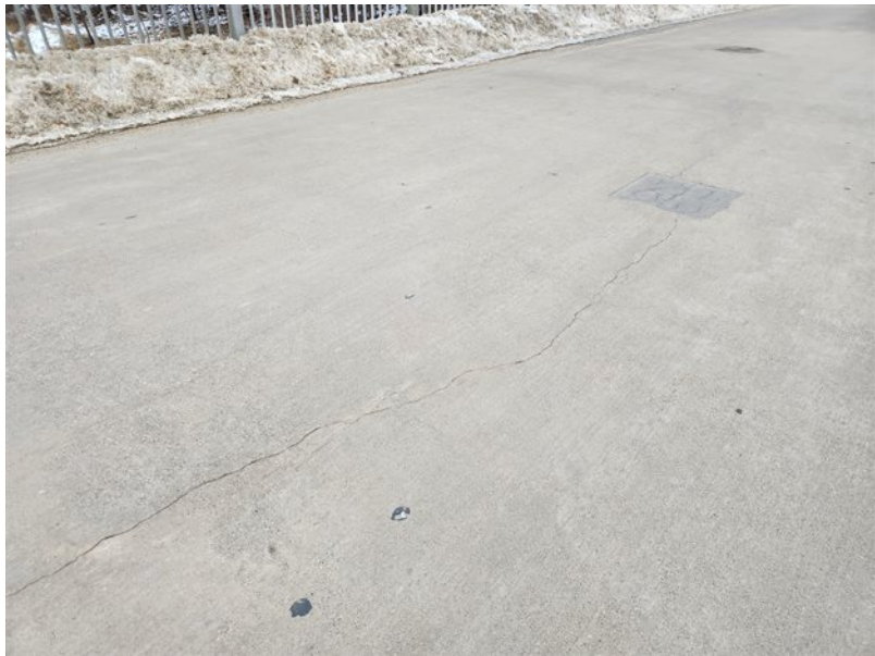
File Description Longitudinal centerline crack on surface of deck
