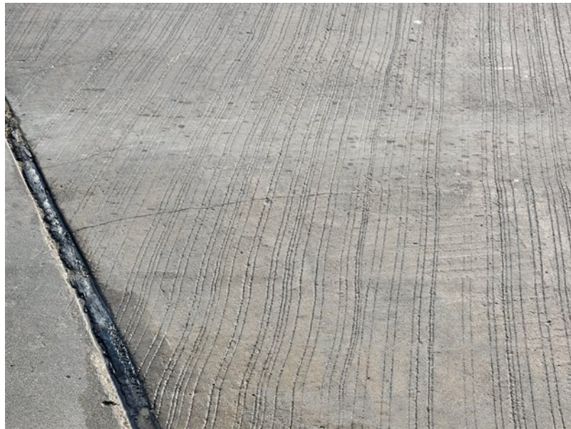
File Description Cracking at ends of deck (typical of both sides)
