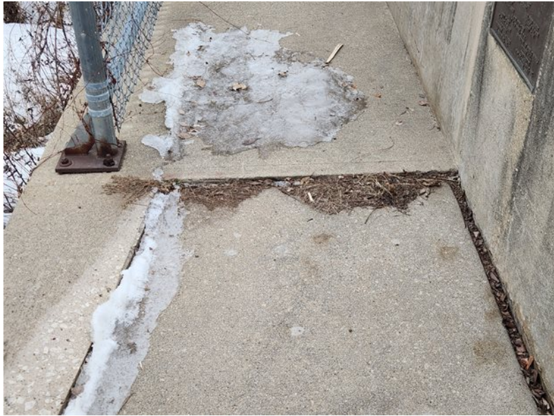
File Description Sidewalk approaches settling
