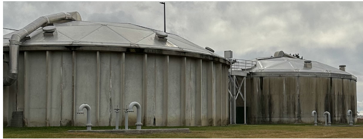
Existing Trickling Filters
