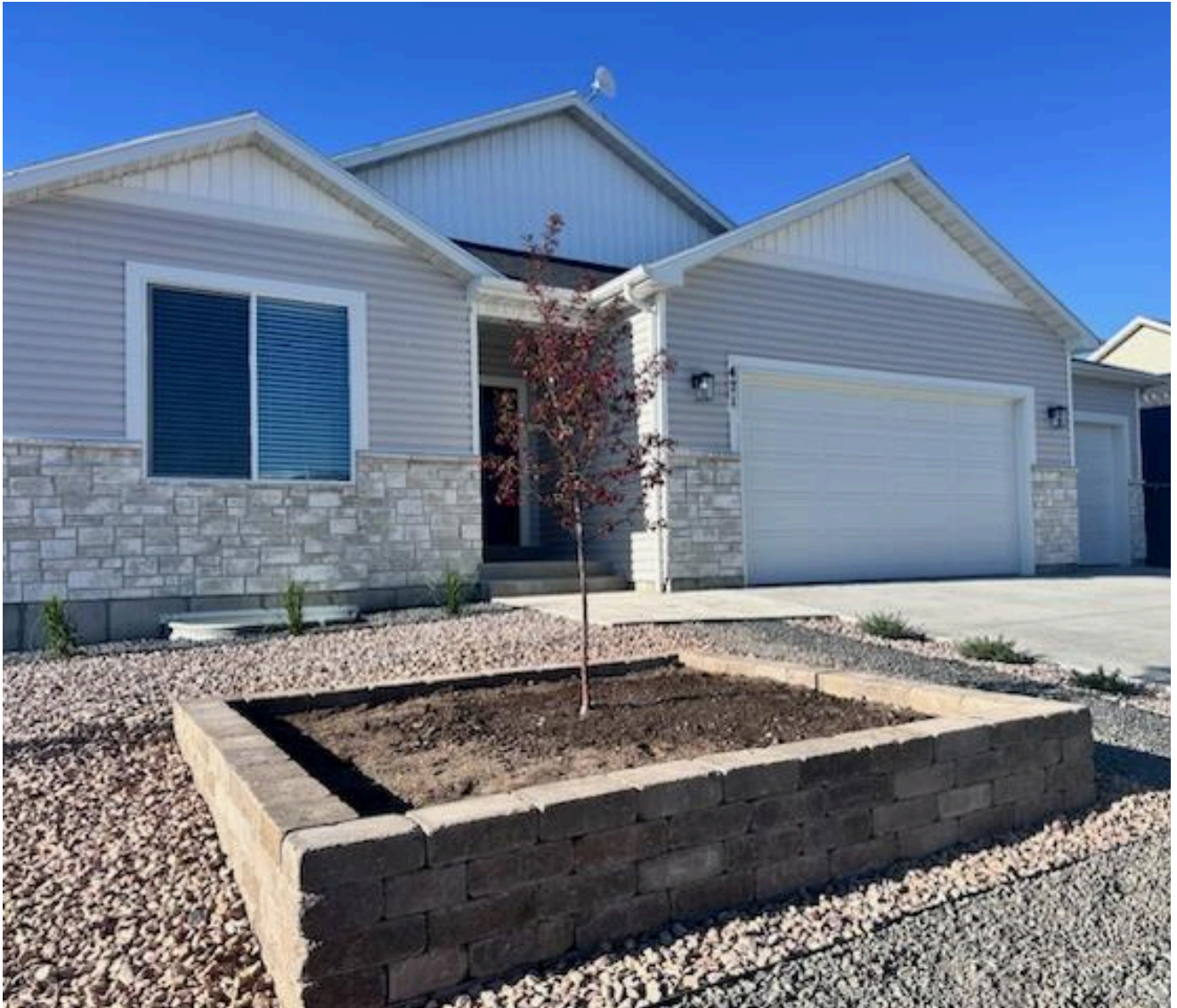
Image D: Front View of House
