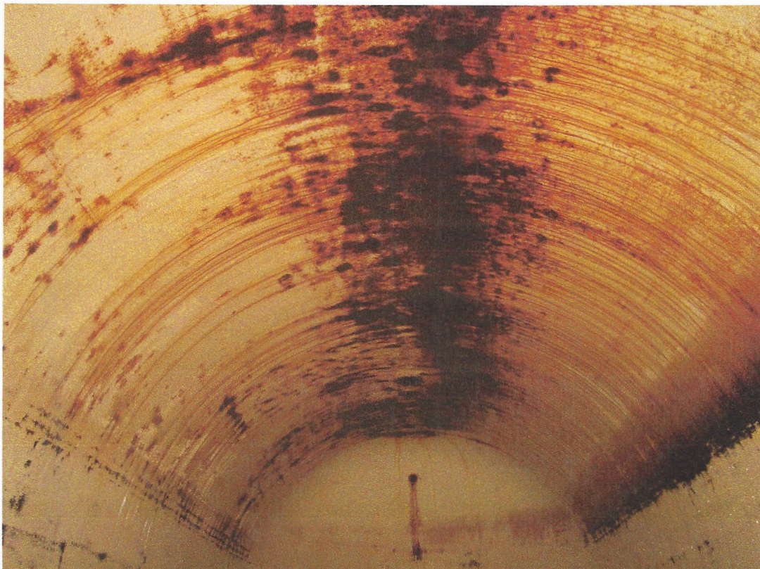
Protective coating failure and corrosion on the weld seams and steel plate above the normal water line.
