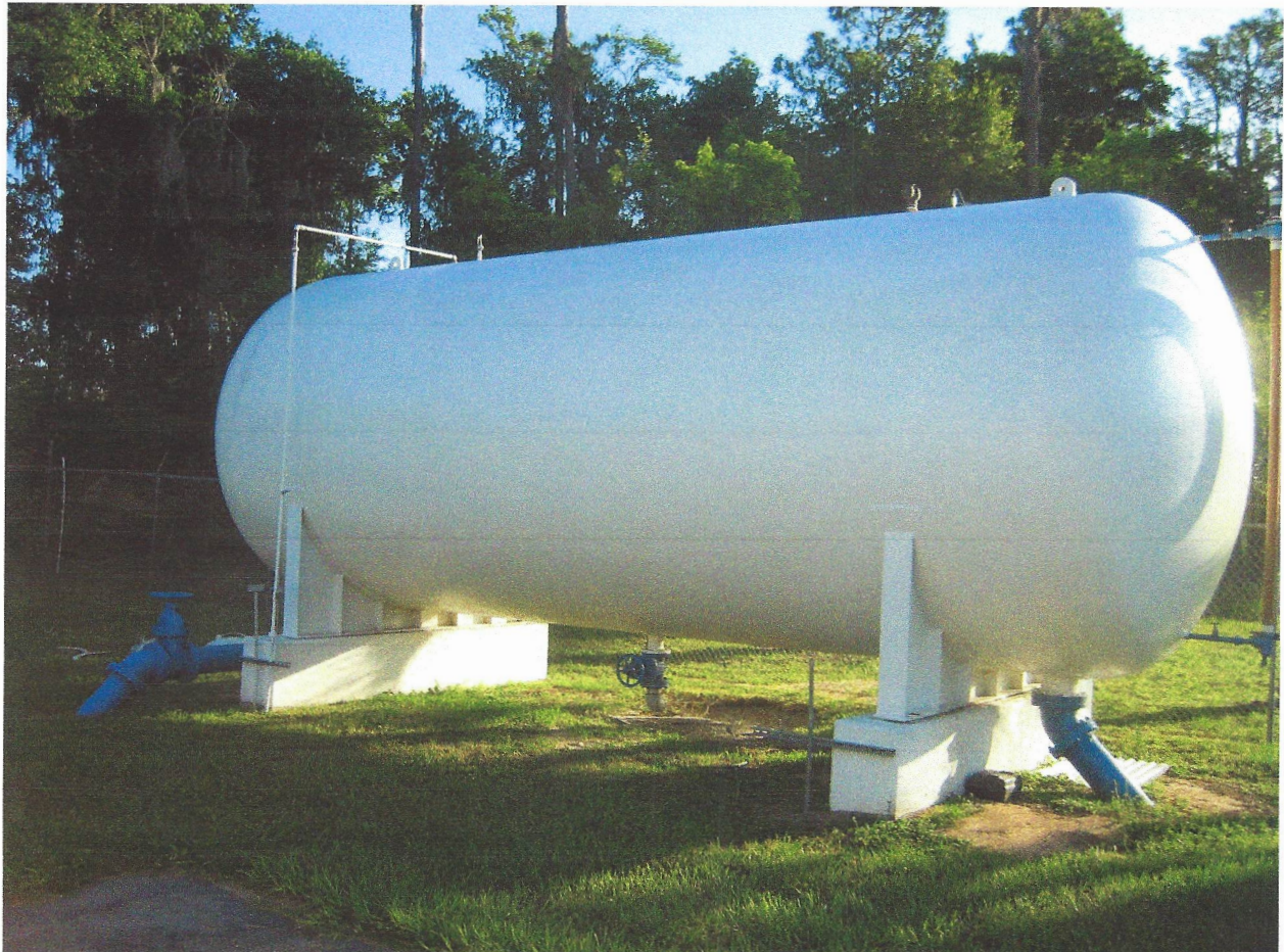
The hydropneumatic tank at Howey-in-the-Hills Well #3.
