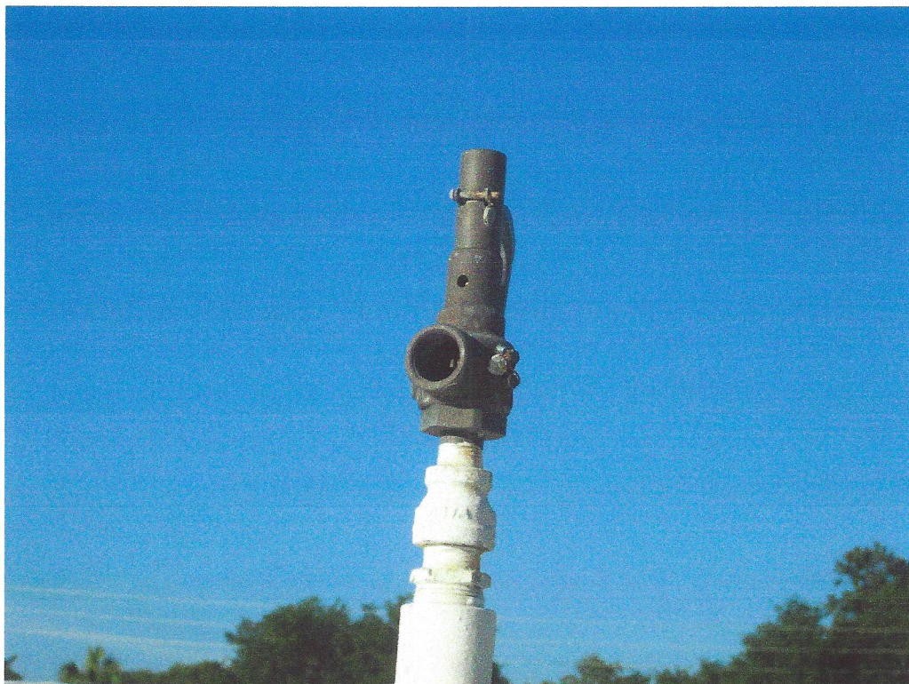
The PRV is not screened.
