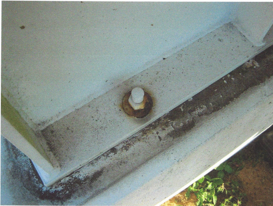
Corrosion on the washers securing the saddle supports to the foundations.
