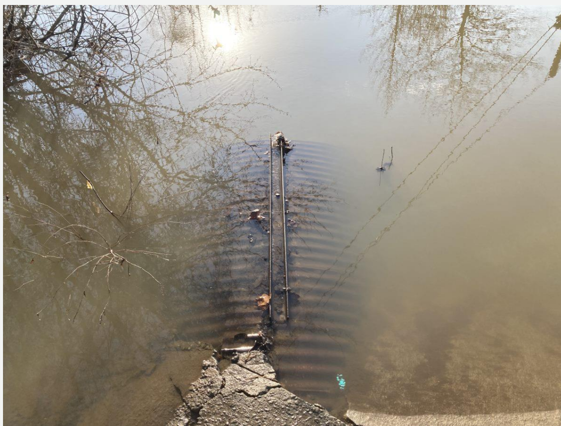
Wash Creek culvert at site – debris collected after heavy rain
