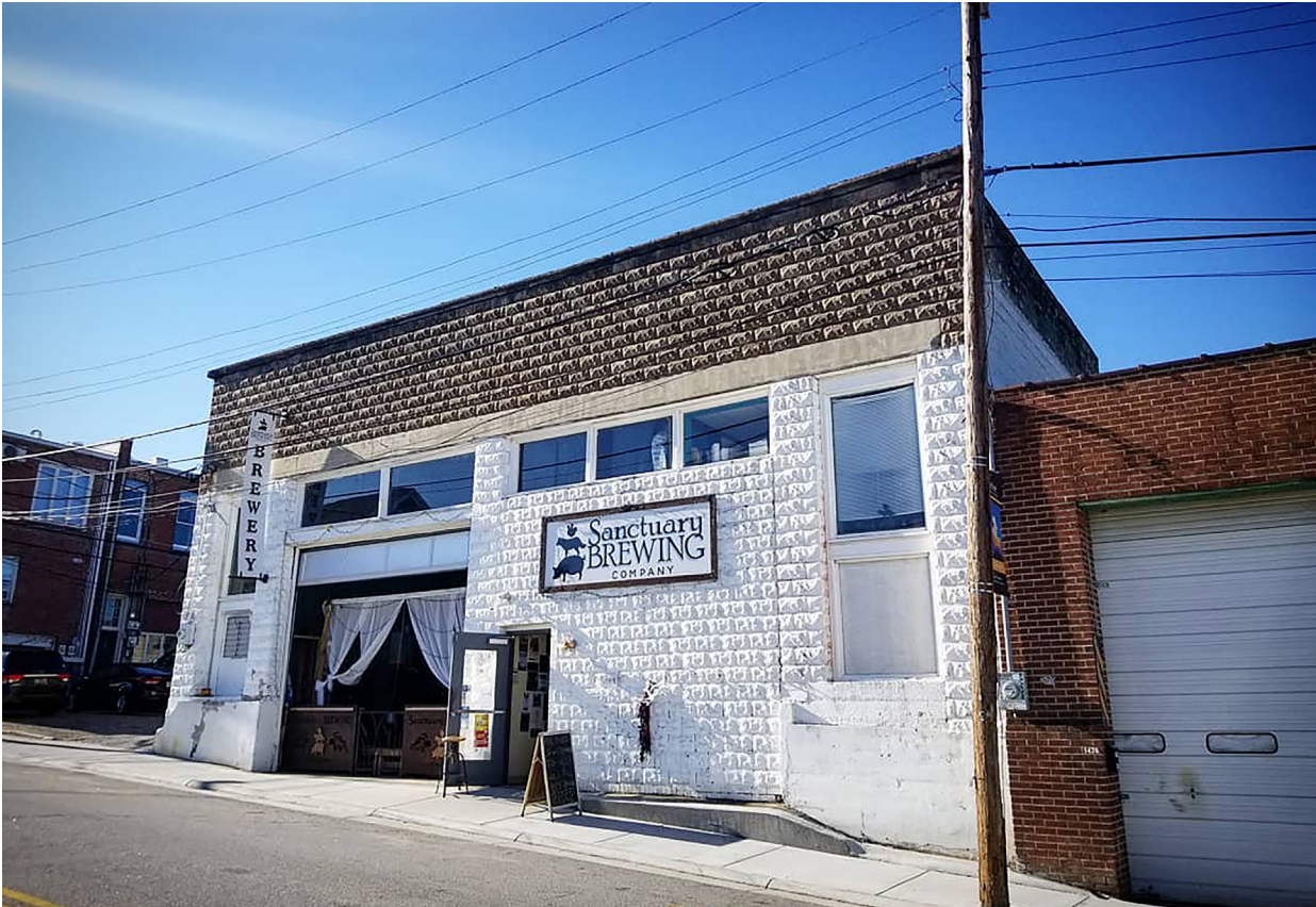
Building Facing South
