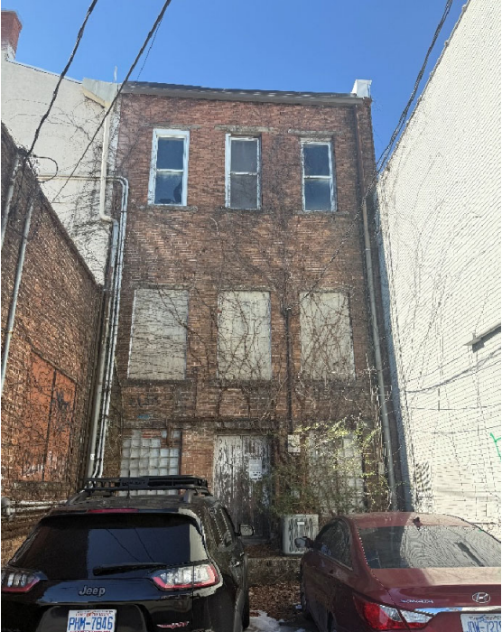
Current rear façade
