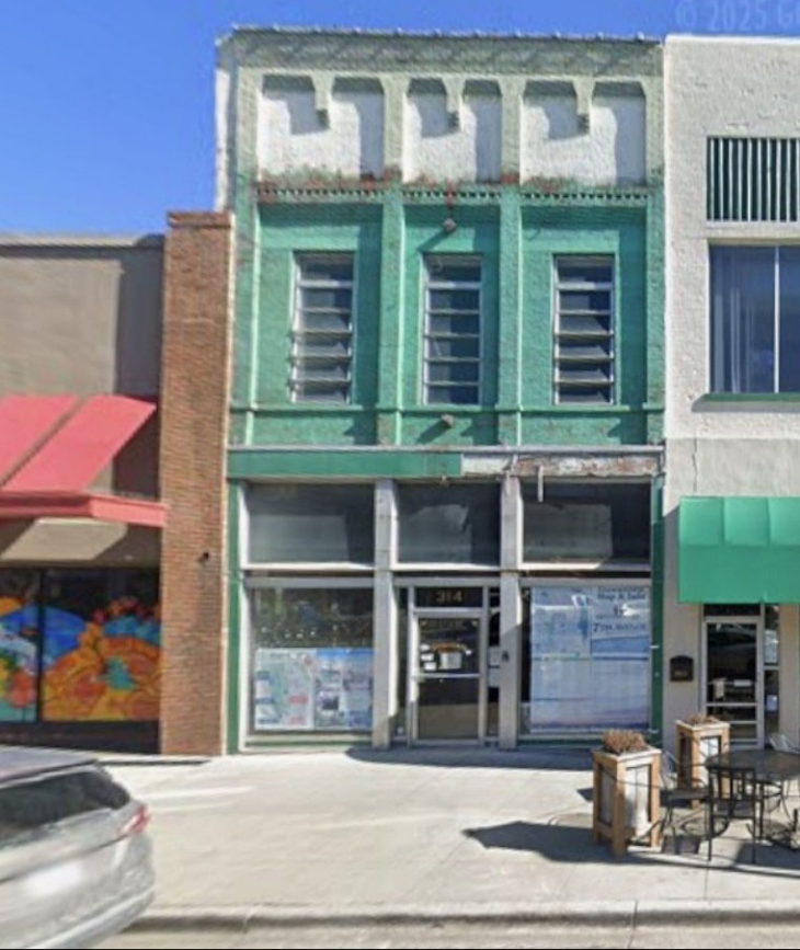
Existing front façade of 314 N Main Street.
