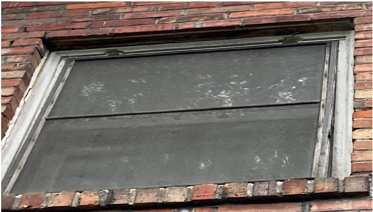
Figure 14 - Rotting Wood Window Frame
