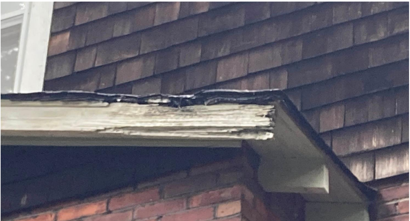
Figure 17 - Damaged/Rotten Eaves and Shingles
