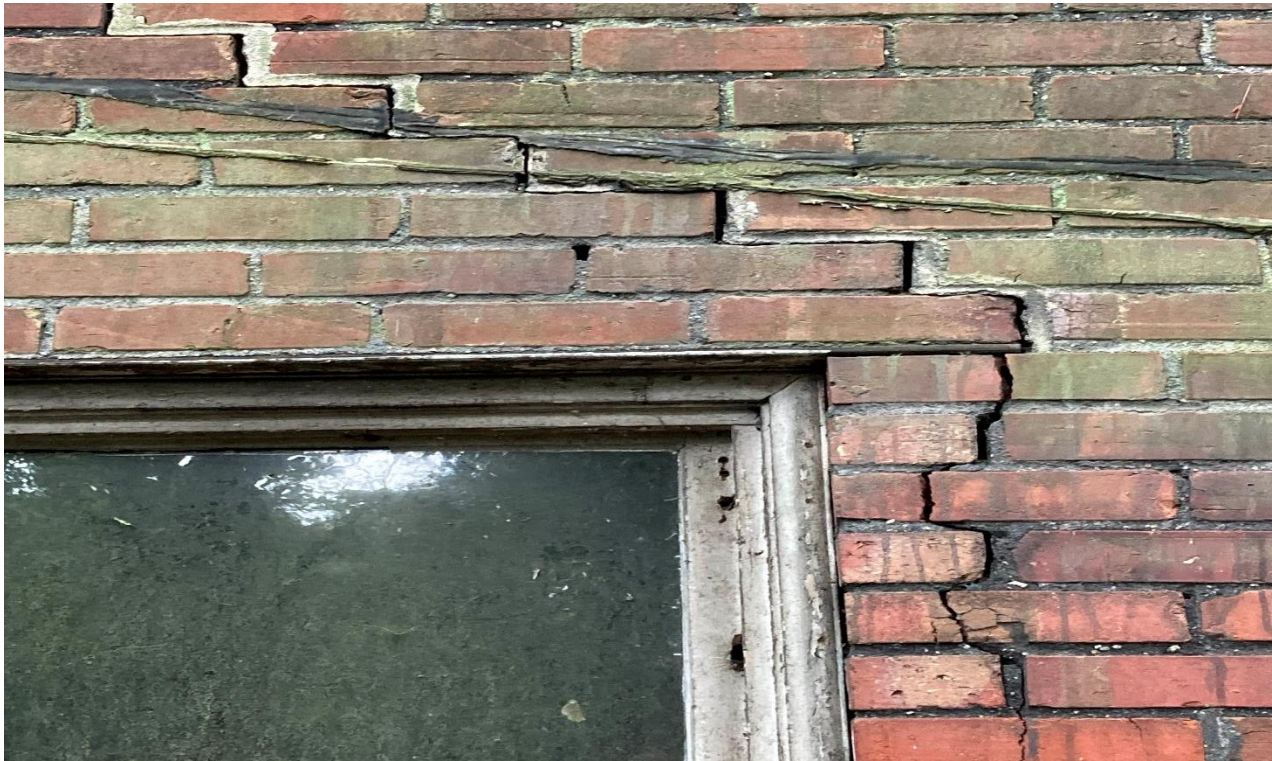
Figure 6 - Missing mortar and crack above window; rotting window frame
