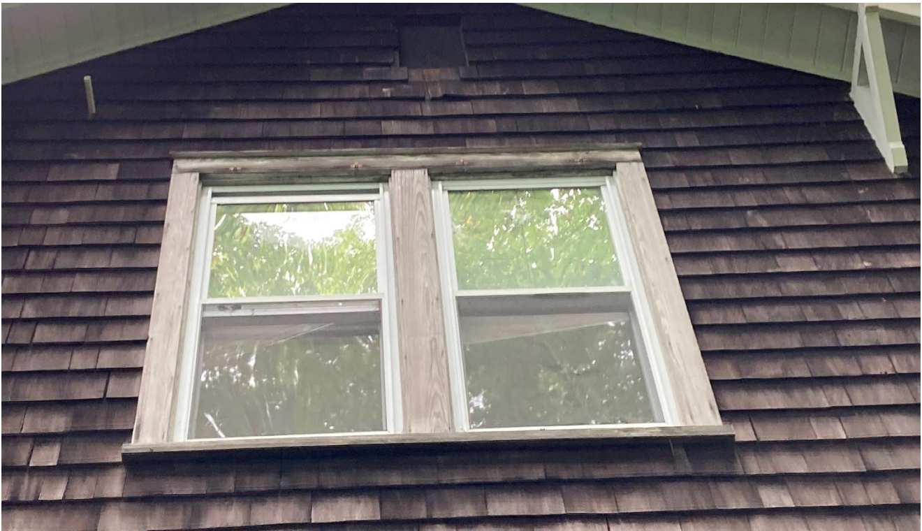
Figure 10 - Exposed/Unpainted Wood Window Trim
