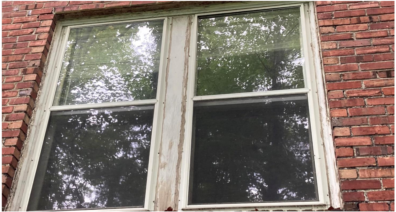
Figure 13 – Rotting/Exposed/Unpainted Wood Window Frame
