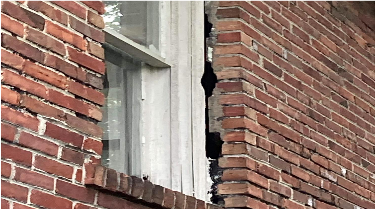
Figure 7 - Gaps between window and frame
