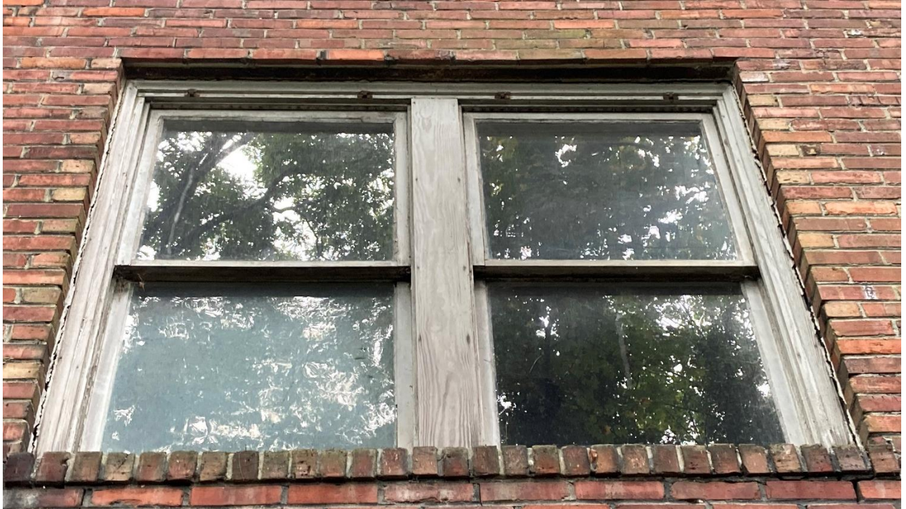
Figure 9 - Exposed/Unpainted Wood Window Trim
