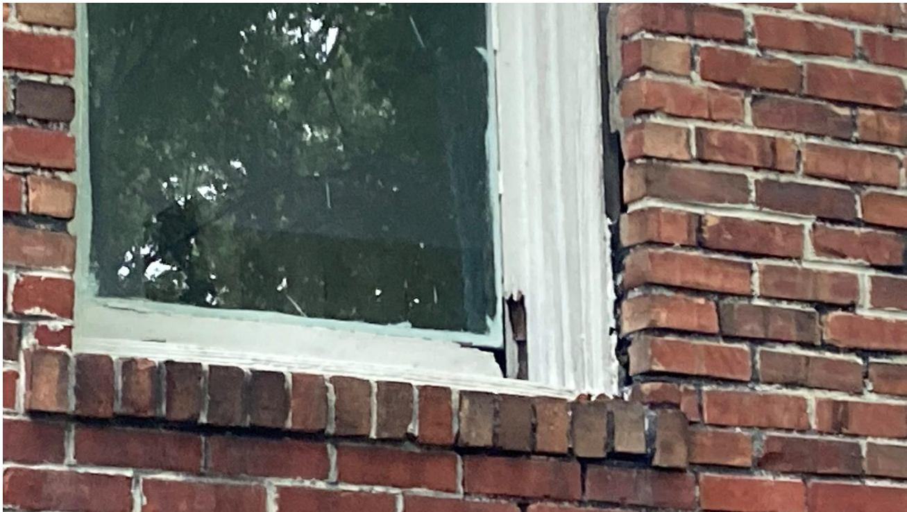
Figure 8 - Rotten/Damaged Window Frame
