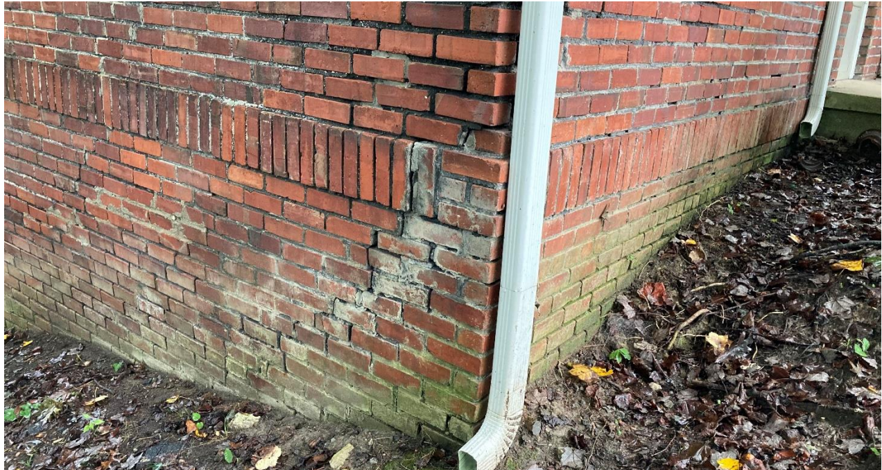
Figure 5 - Cracks in Foundation Masonry
