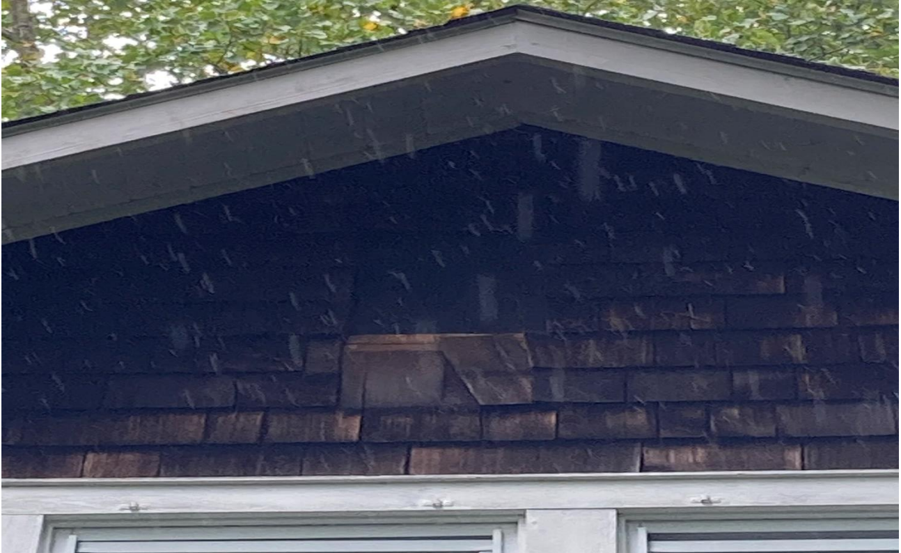
Figure 16 - Damaged Shingle
