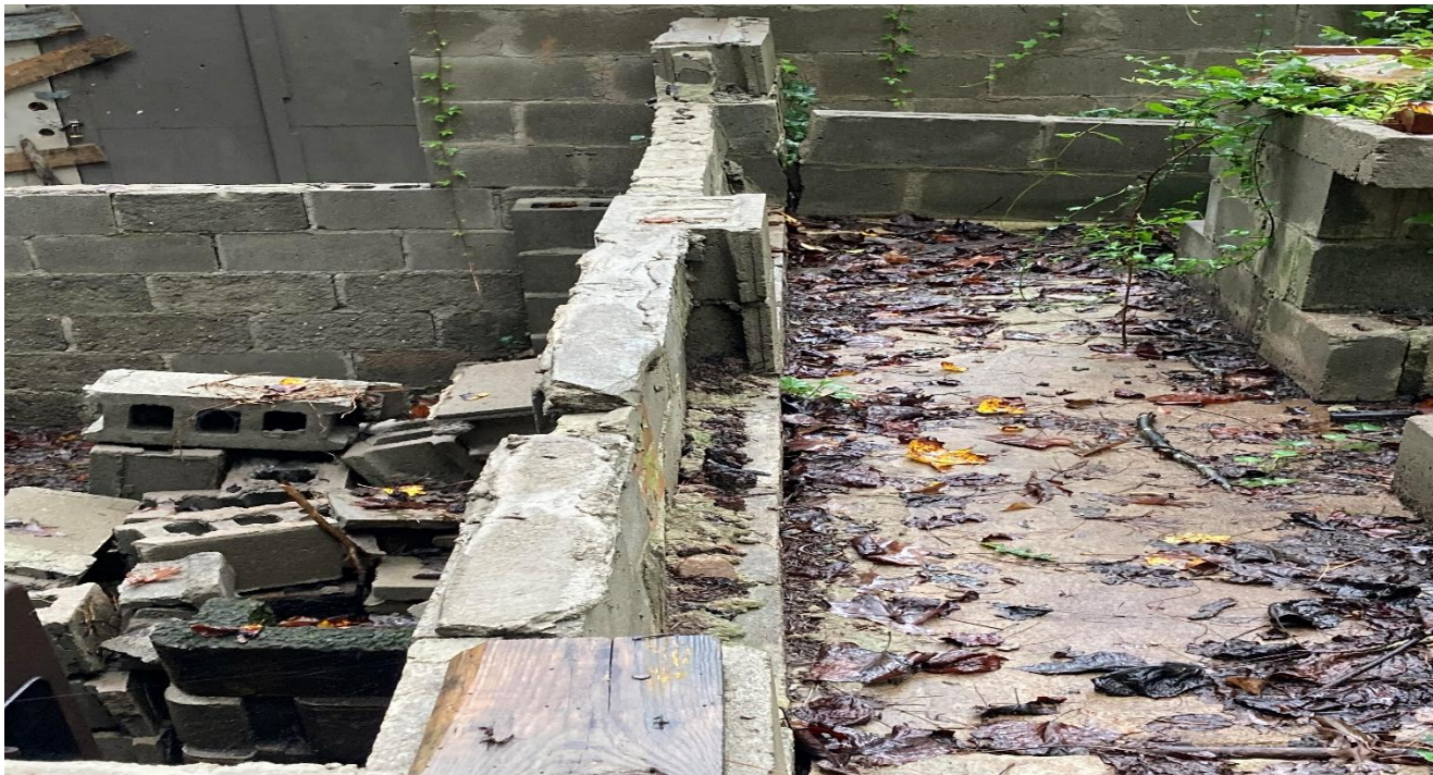
Figure 12 – Leaning Foundation/Wall for Former Boiler Room /Greenhouse
