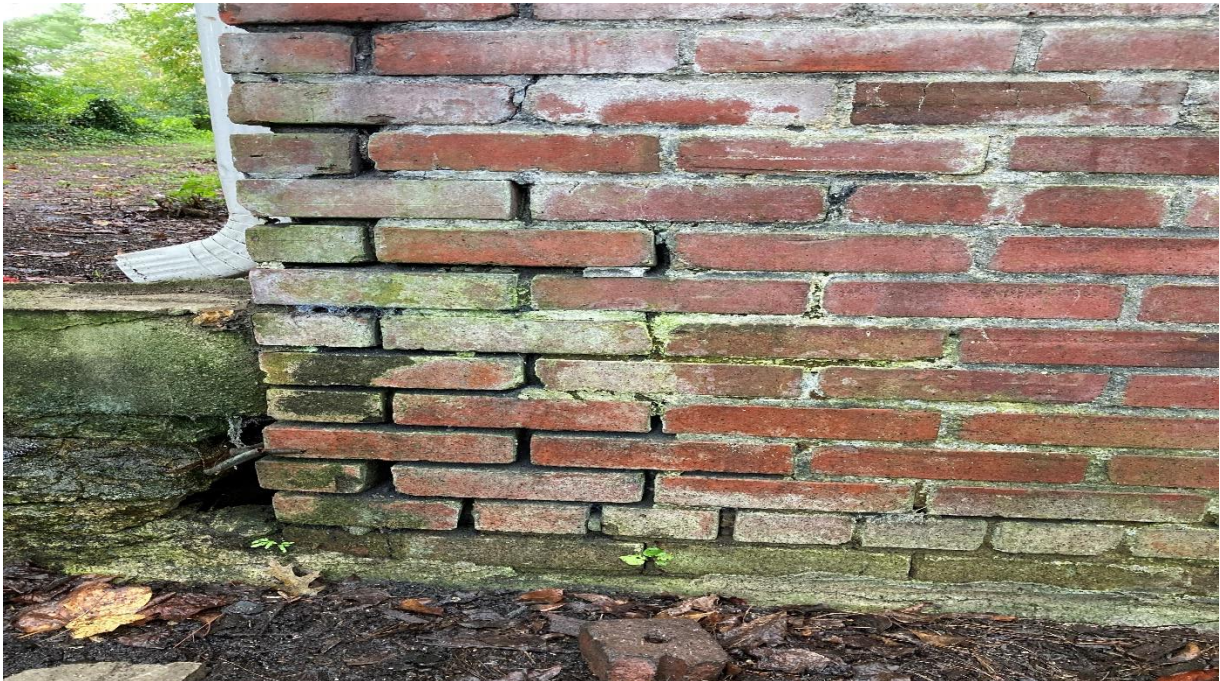
Figure 1 - Missing Mortar
