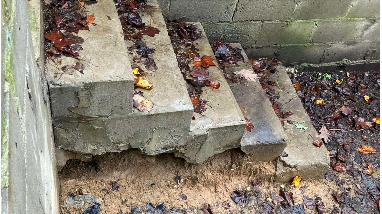
Figure 11 - Erosion Underneath Exterior Concrete Stairs
