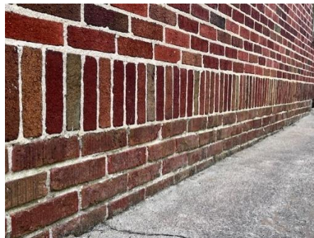
Appendix A: 41 Solider Course between foundation and facade
