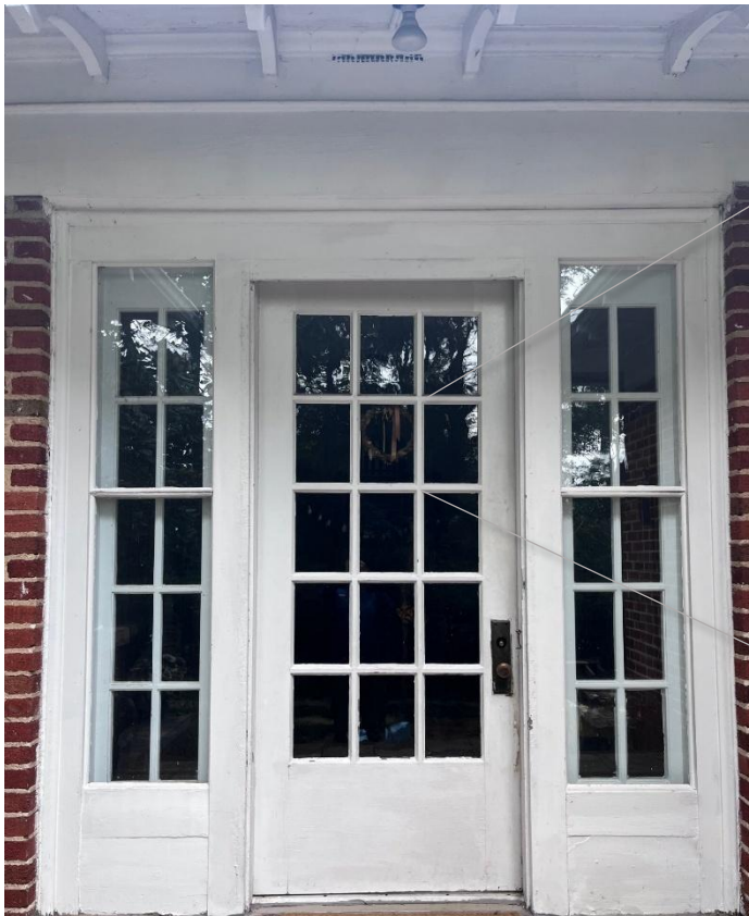
Appendix A 14: 15-Lite Side Stoop Door featuring 2 - 10-Pane Sidelites
