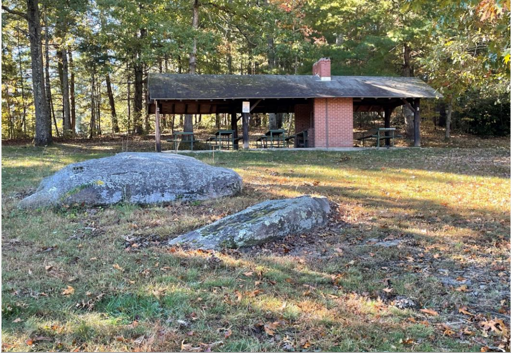
View of the existing shelter facilities (to be removed)
