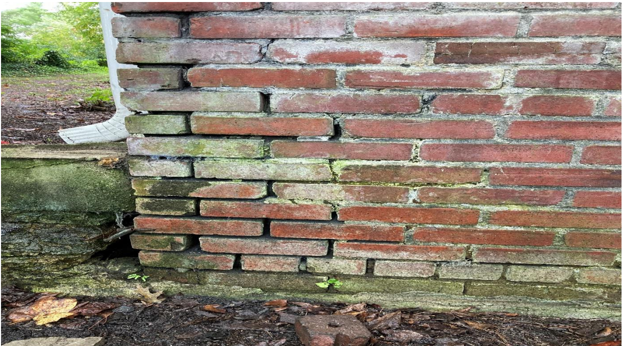
Figure 1 - Missing Mortar
