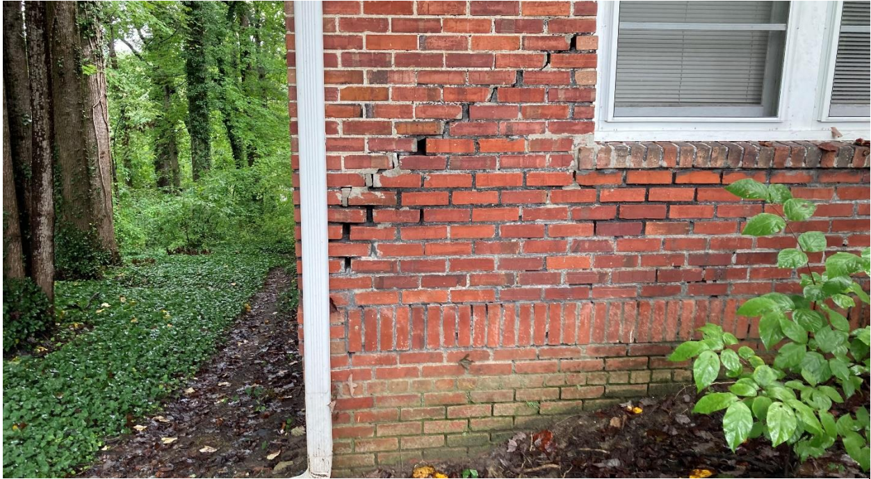
Figure 3 - Missing/Damaged Mortar
