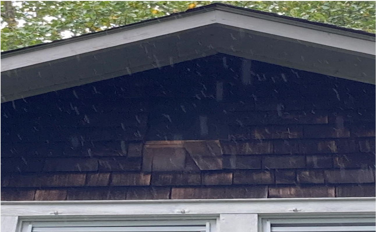
Figure 16 - Damaged Shingle
