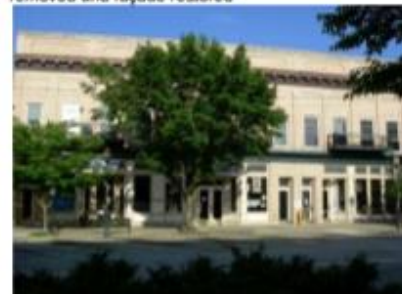
Houston Furniture building after metal cladding removed and façade restored
