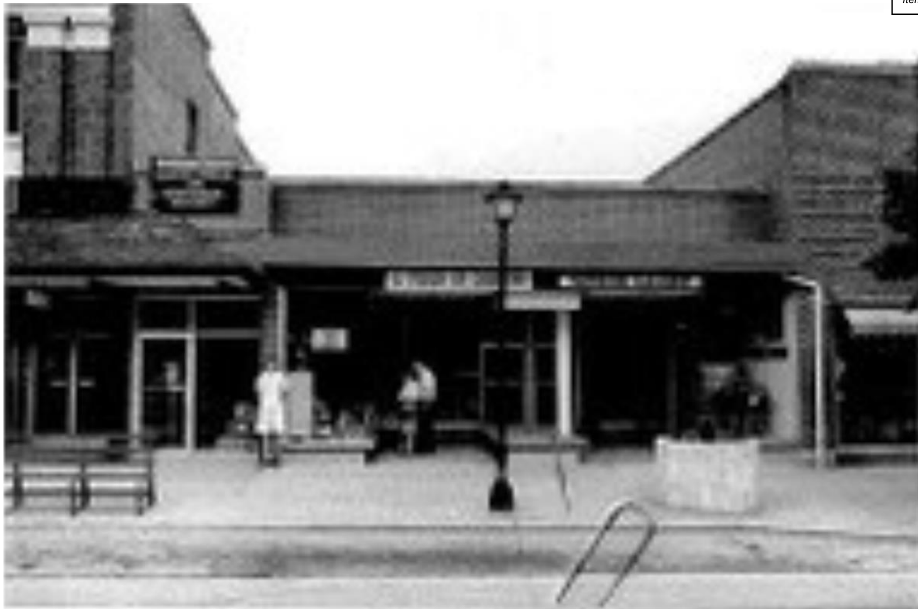
Photo of Subject Property – Dated 1987 | Quality of photo lacks sufficient detail of storefront design and materials.
