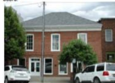
Retain and preserve original windows and doors.
