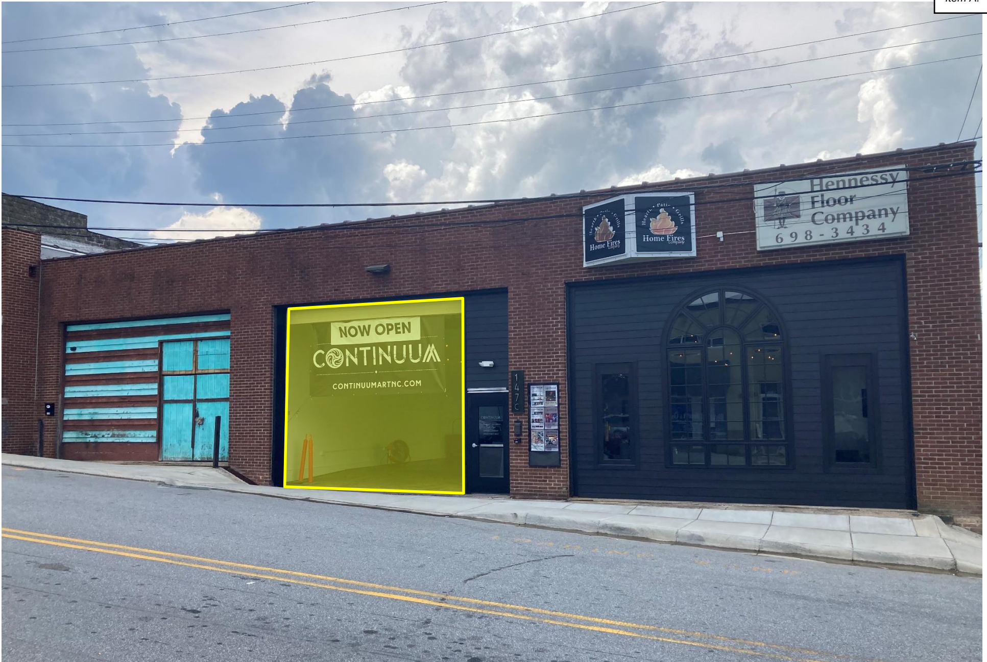
Photo of Subject Property – Current – Door Opening Highlighted
