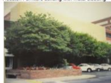
Houston Furniture building with metal cladding
