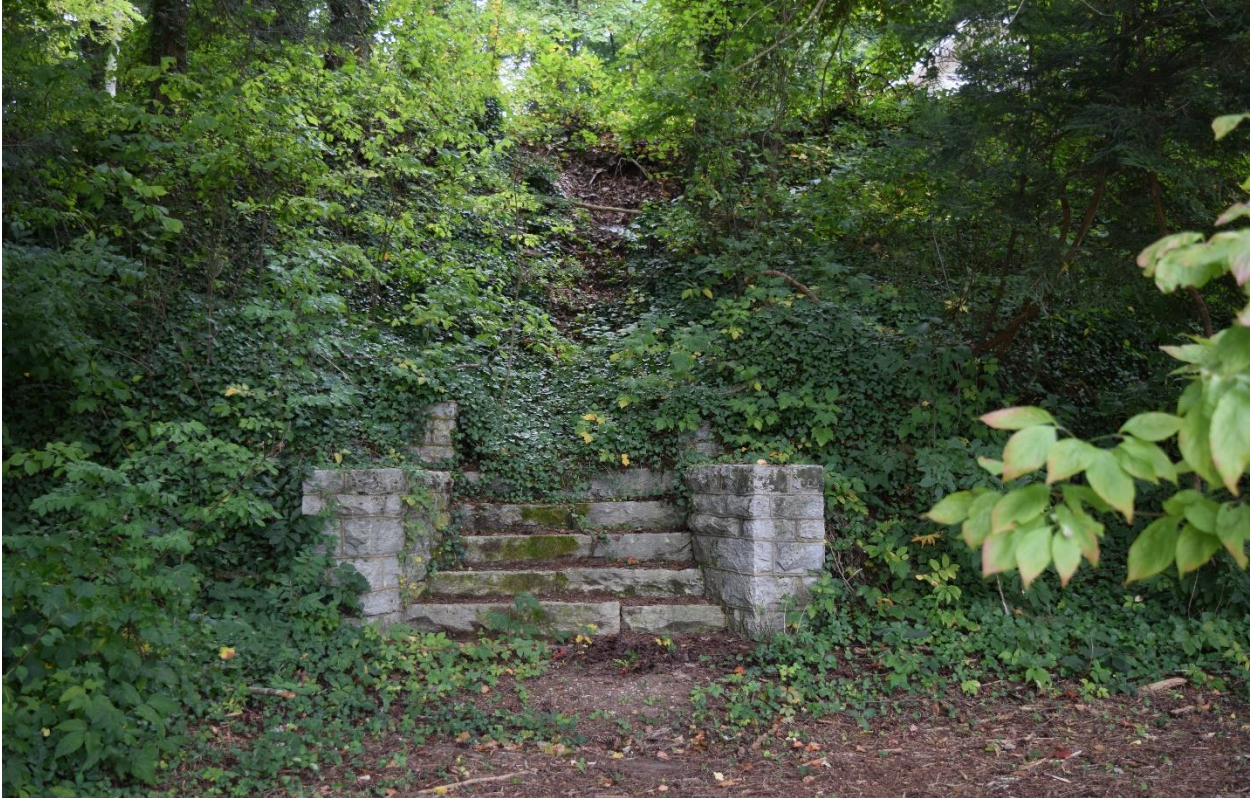
10. Stone staircase at southwest edge of property, view southwest
