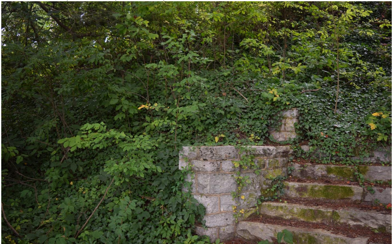
13. Staircase at rear of spring, view southeast
