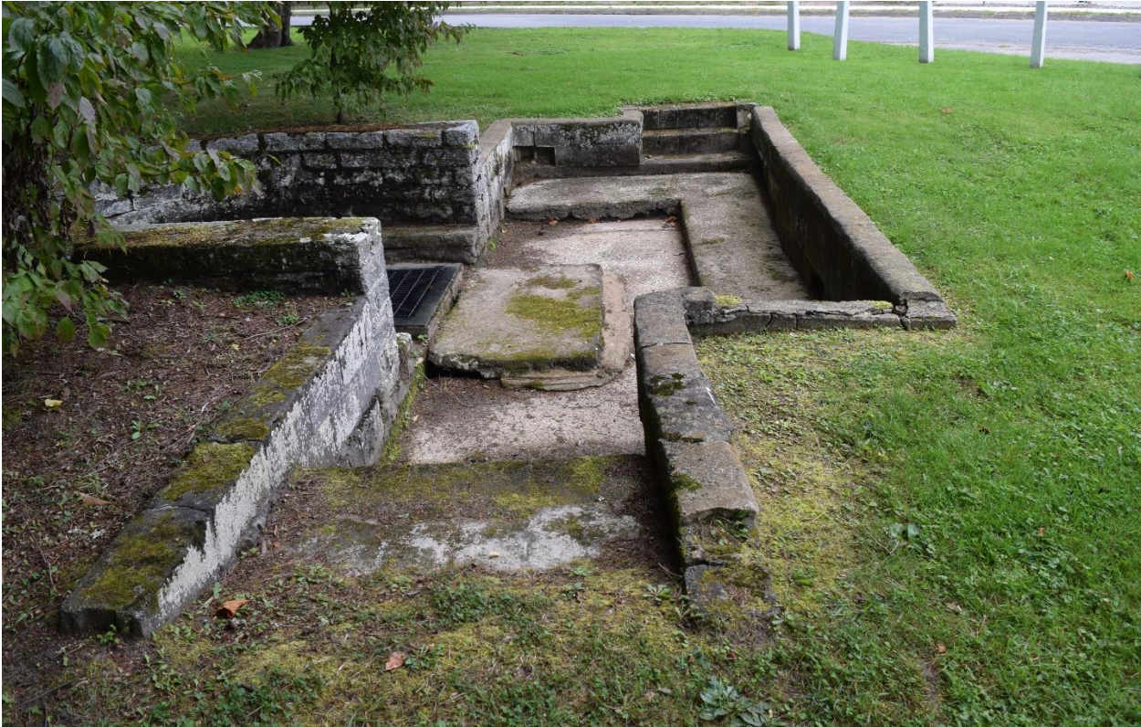
9. Lenox Spring stonework, view northwest
