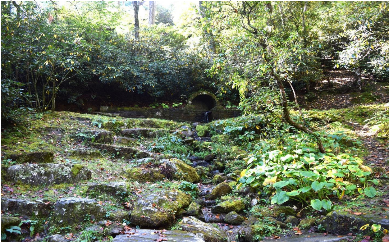
Crystal Spring and stonework, view southwest
