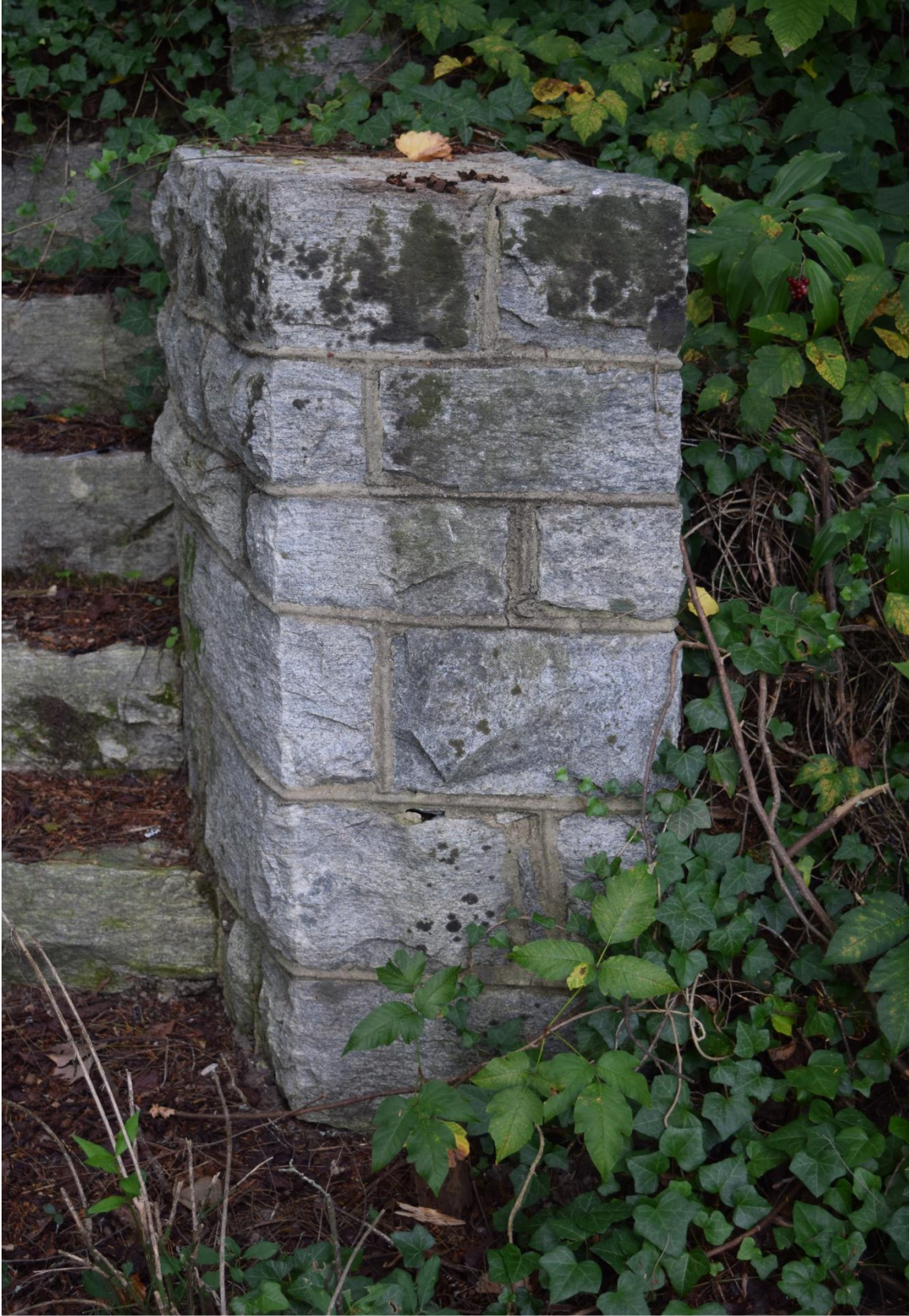
11. Close-up view of stonework on staircase, granite with beaded mortar joints
