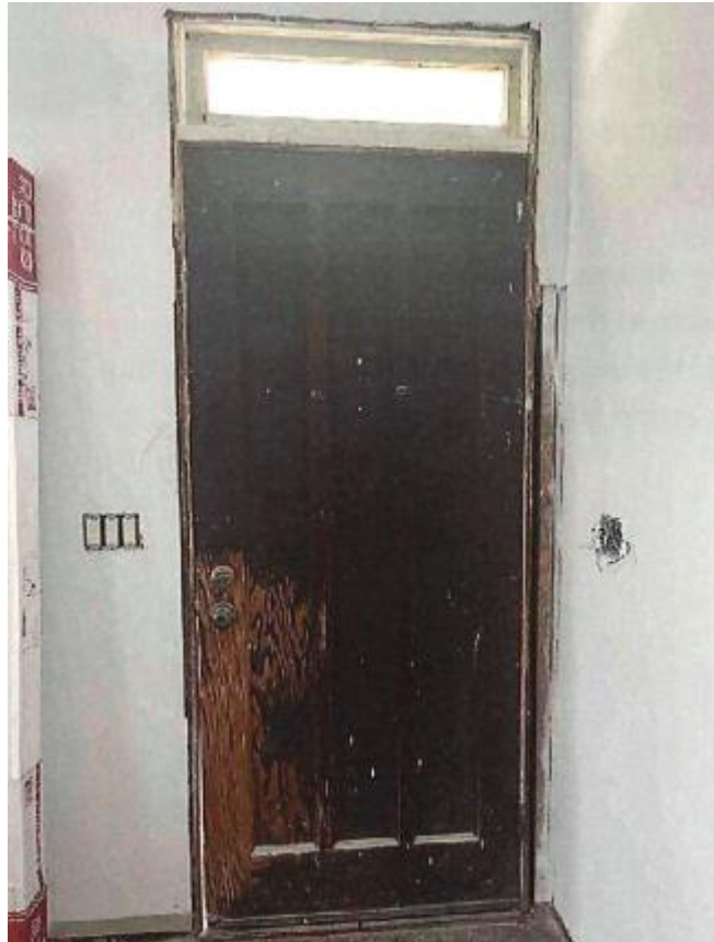
Damage to interior of front door.
