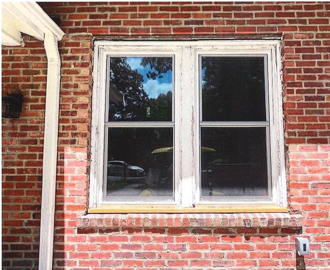
NEW WINDOWS WITH OLD FRAMES: FRONT RIGHT
