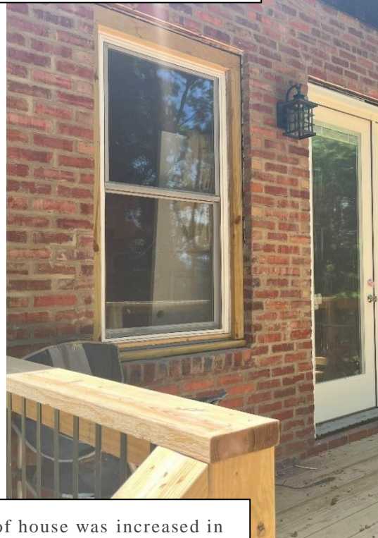
The original back door was removed and replaced with a window. Brick was used to fill in underneath the window.
