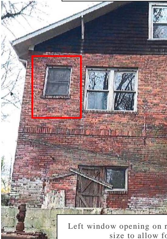
The original back door was removed and replaced with a window. Brick was used to fill in underneath the window.
