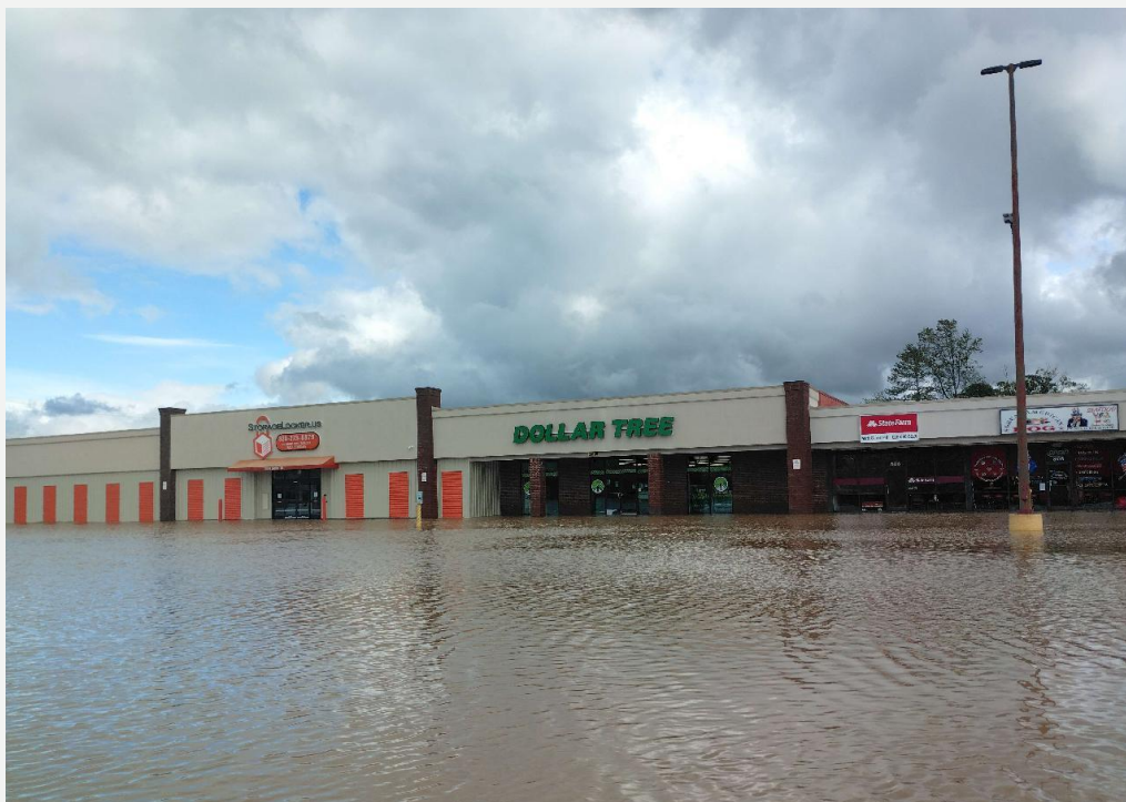
View of the plaza across the street from subject property during Hurricane Helene (9-27-2024)
