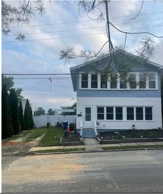
Front view of house and view of side yard where proposed addition would be constructed.
