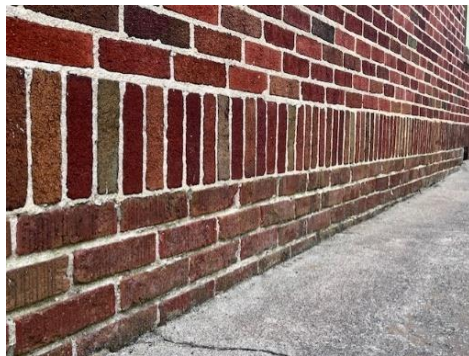
Baler Appendix A: 41 Solider Course between foundation and facade
