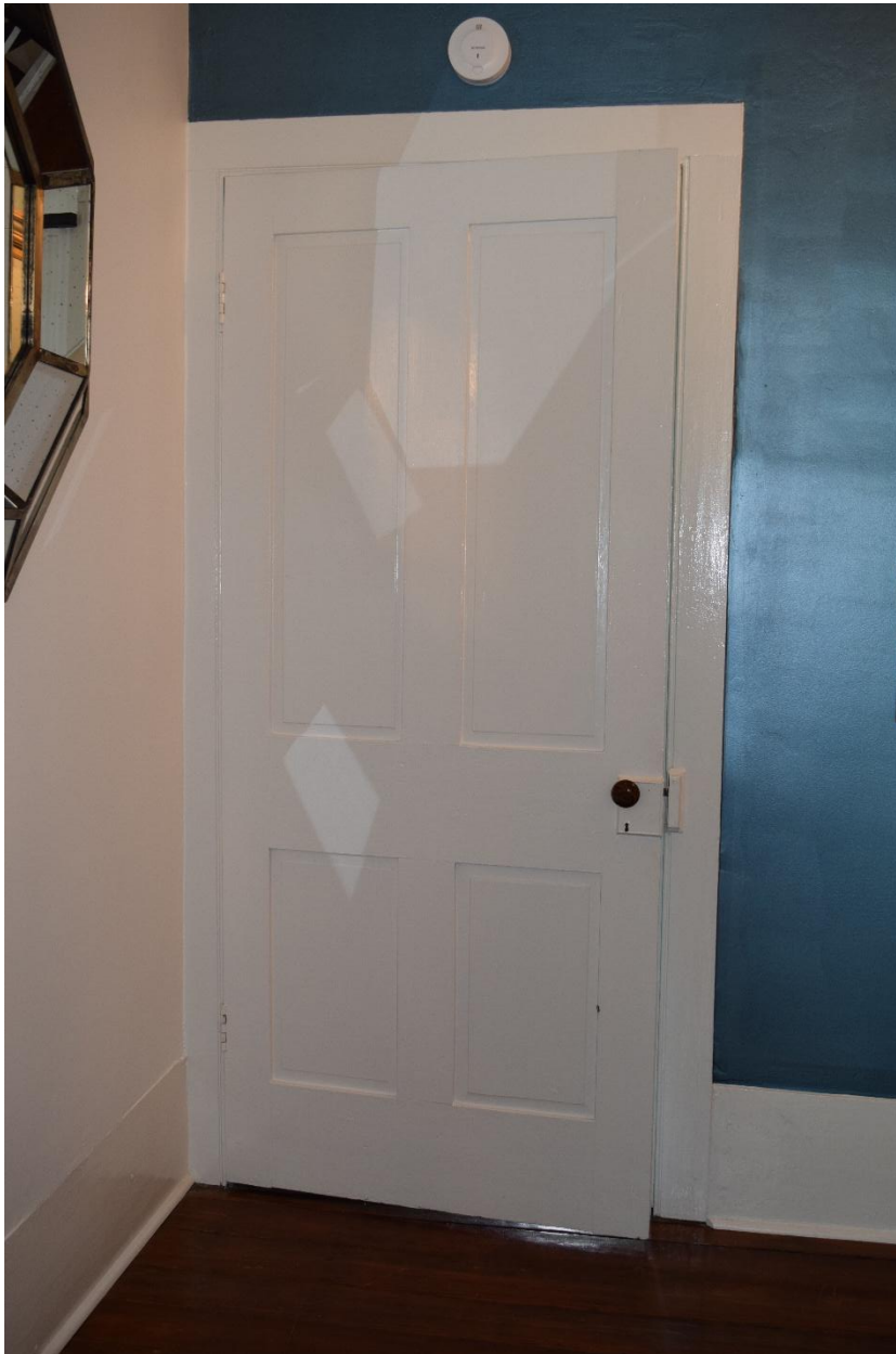
51. Typical four-panel door throughout house
