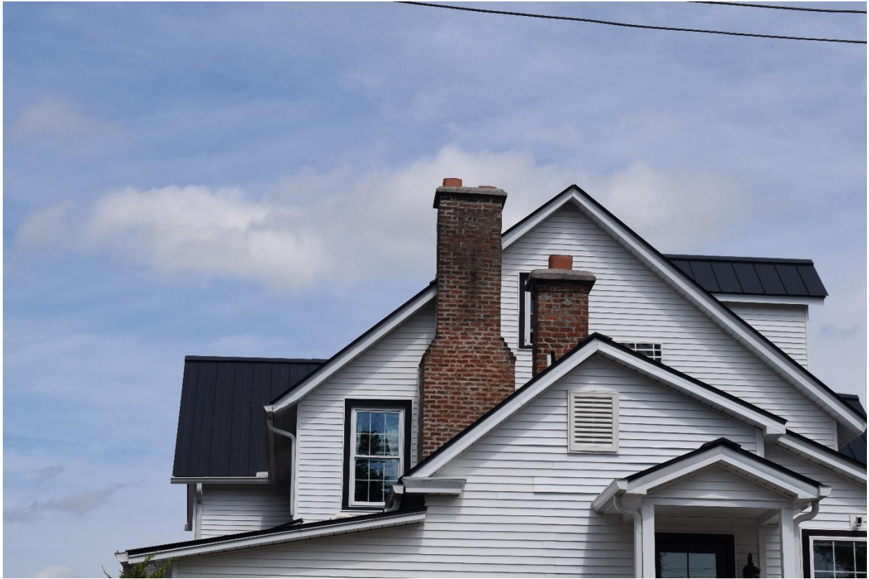
13. West elevation rooflines, view east
