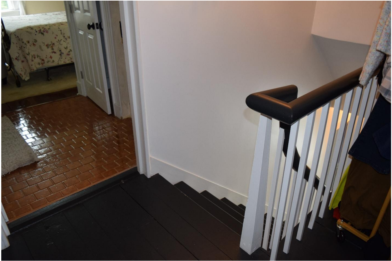
69. Attic stair detail
