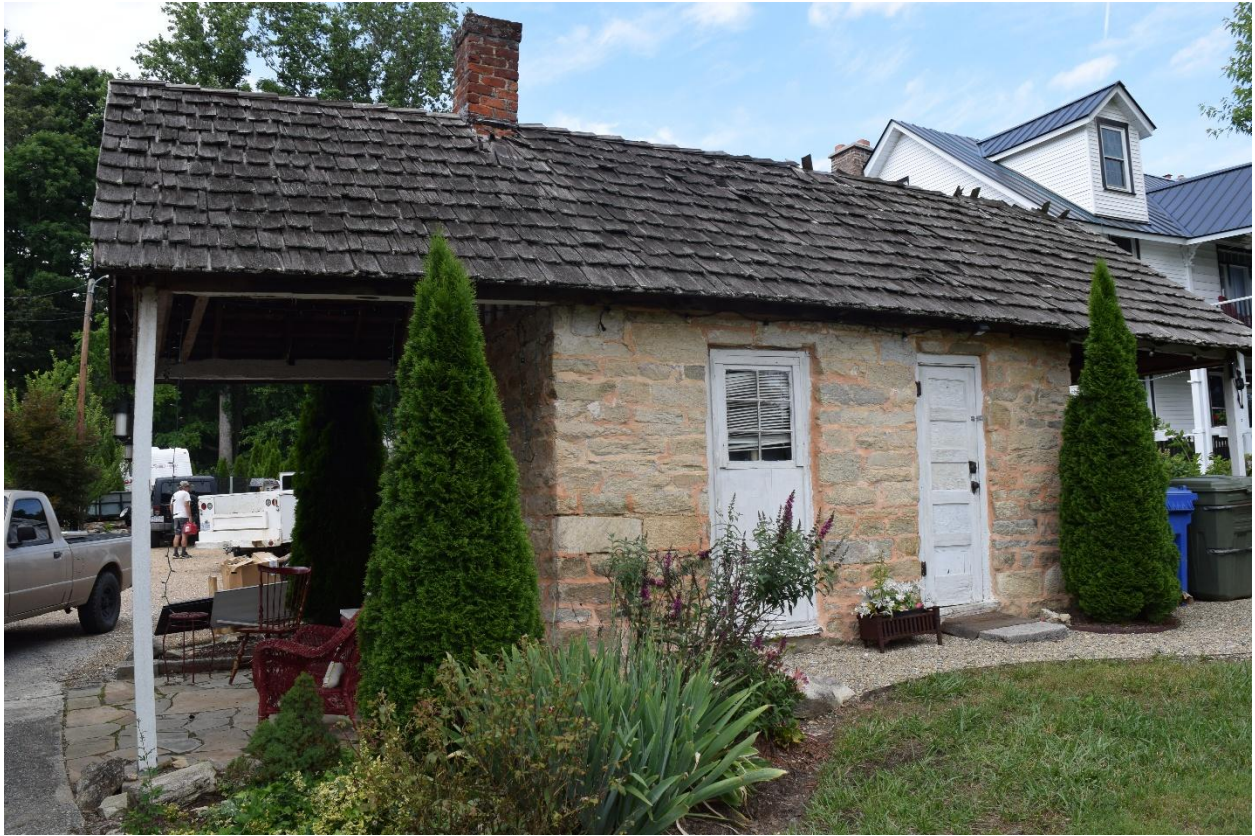
16. South elevation carriage repair stone outbuilding, view north
