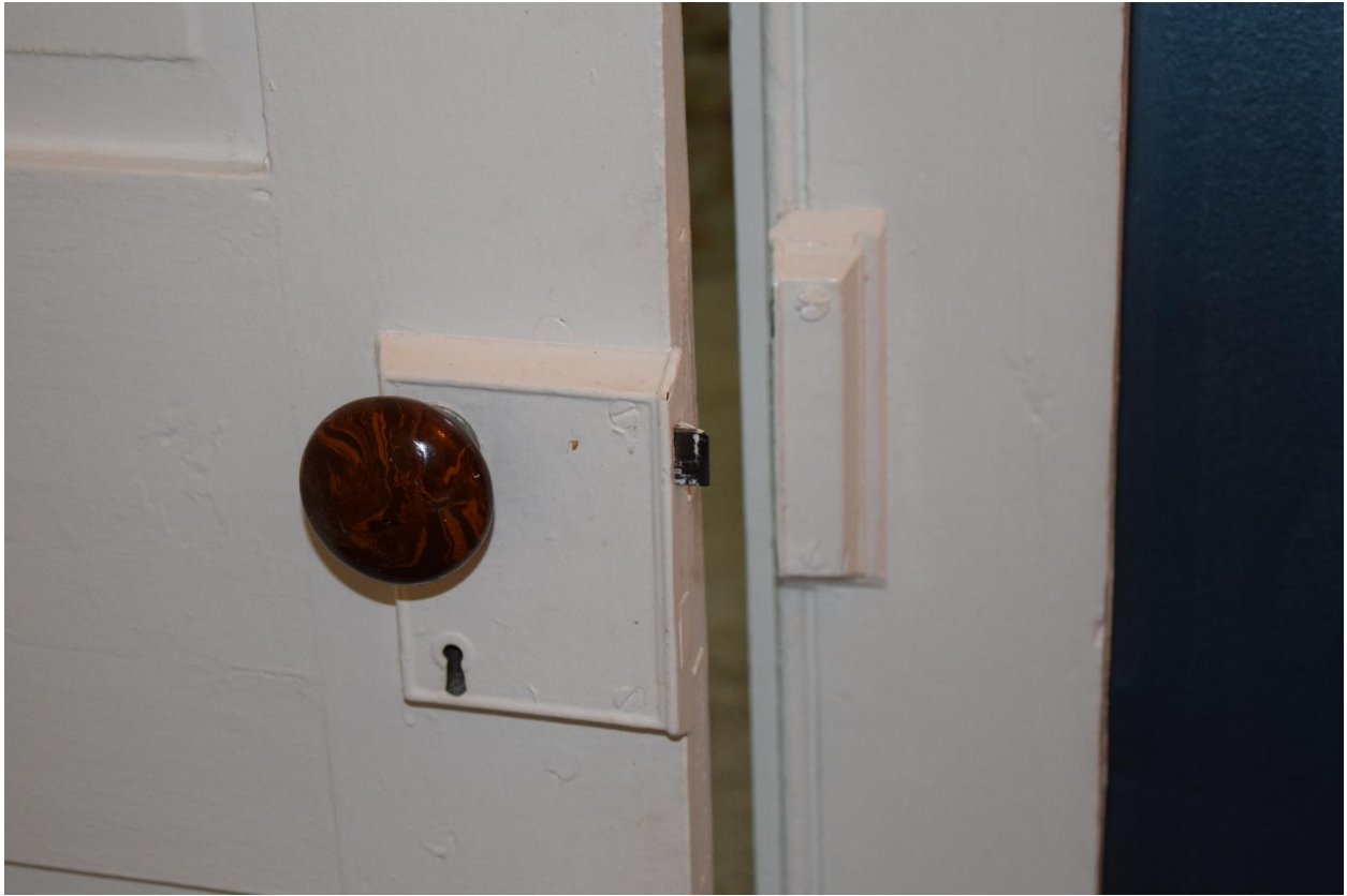
52. Typical hardware throughout house
