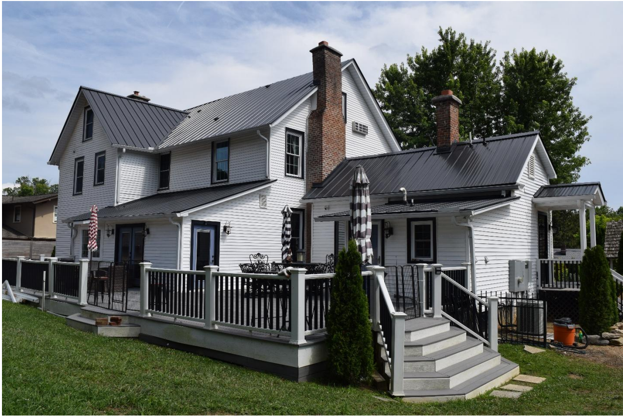
11. West elevation, view southeast
