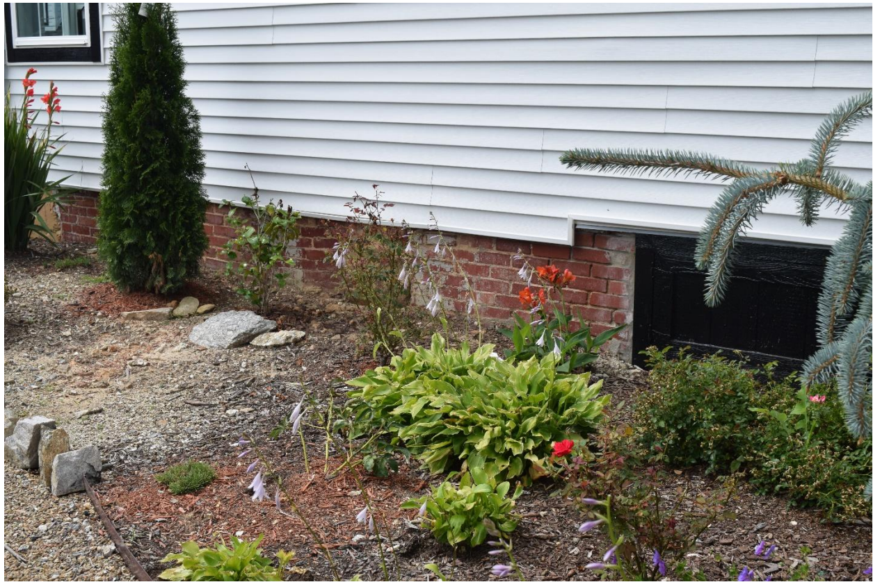
9. Brick foundation beneath kitchen wing, view northwest
