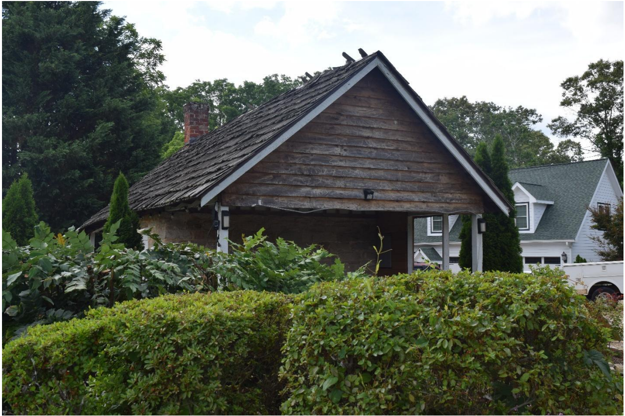
17. East elevation, carriage repair stone outbuilding, view west
