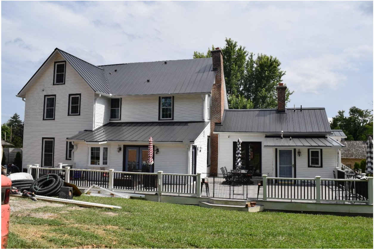
12. North elevation, view south
