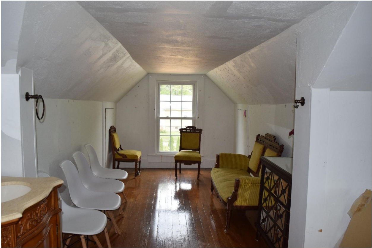
72. Attic bedroom, view north
