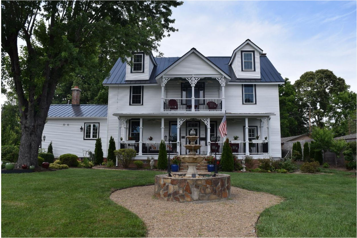
4. Front of house, view north
