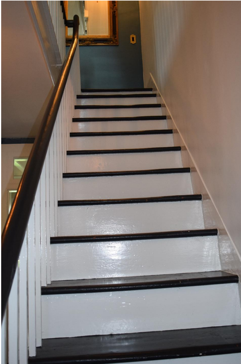
39. Staircase to second floor
