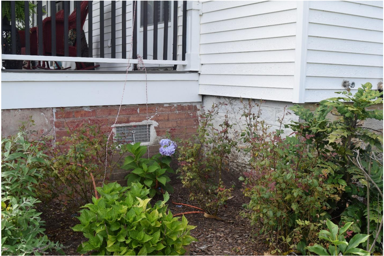
8. House and porch foundation, southeast corner of house
