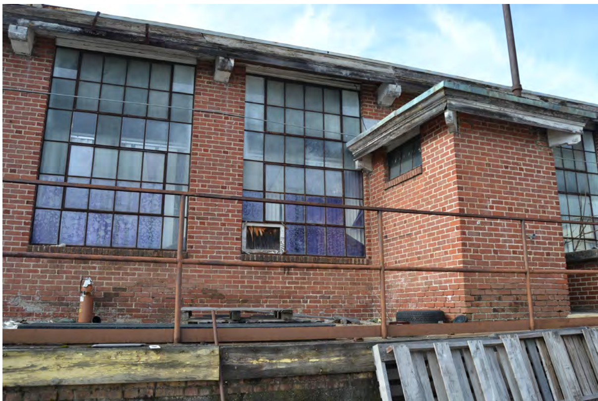
21. Grey Mill, 1919 Building, East Elevation, Window Detail
