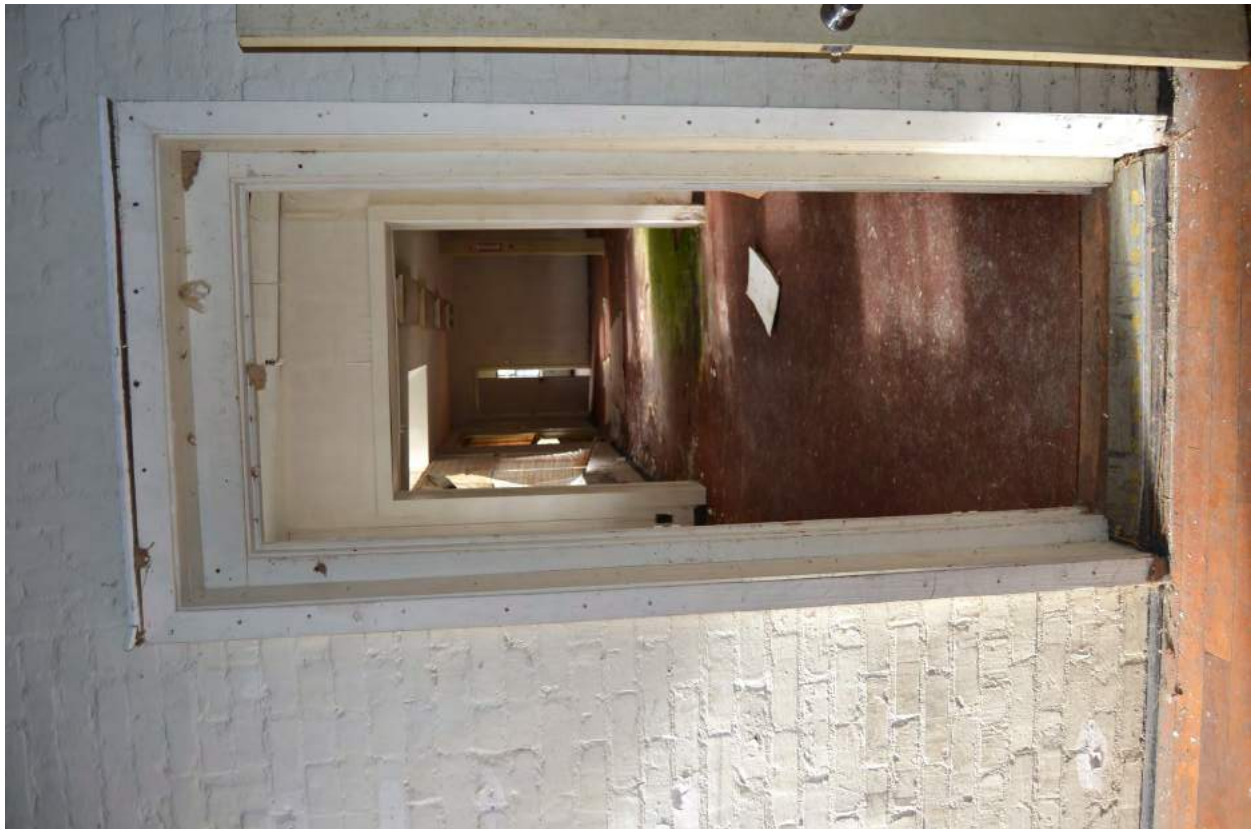
27. Grey Mill, 1919 Building to Office, Looking West
