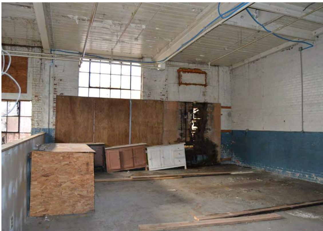
80. Grey Mill, 1926 Addition, Looking West
