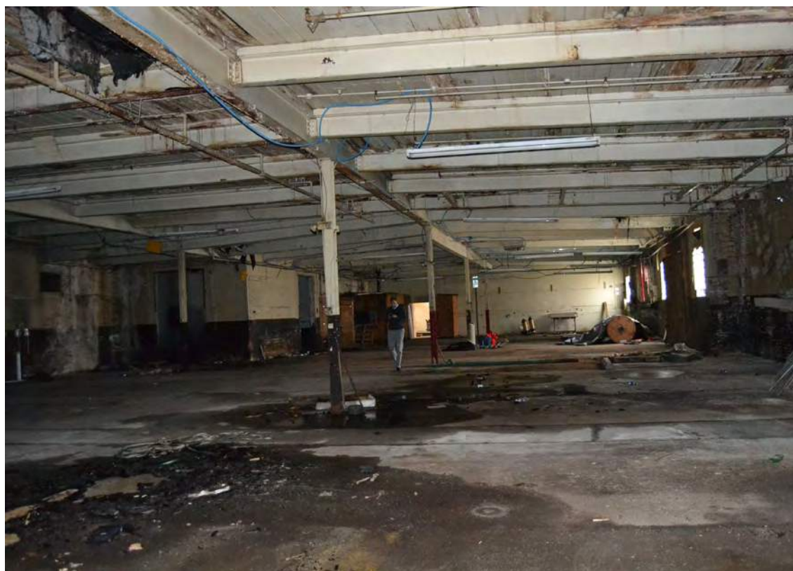
48. Grey Mill, 1947 Addition, Looking South
