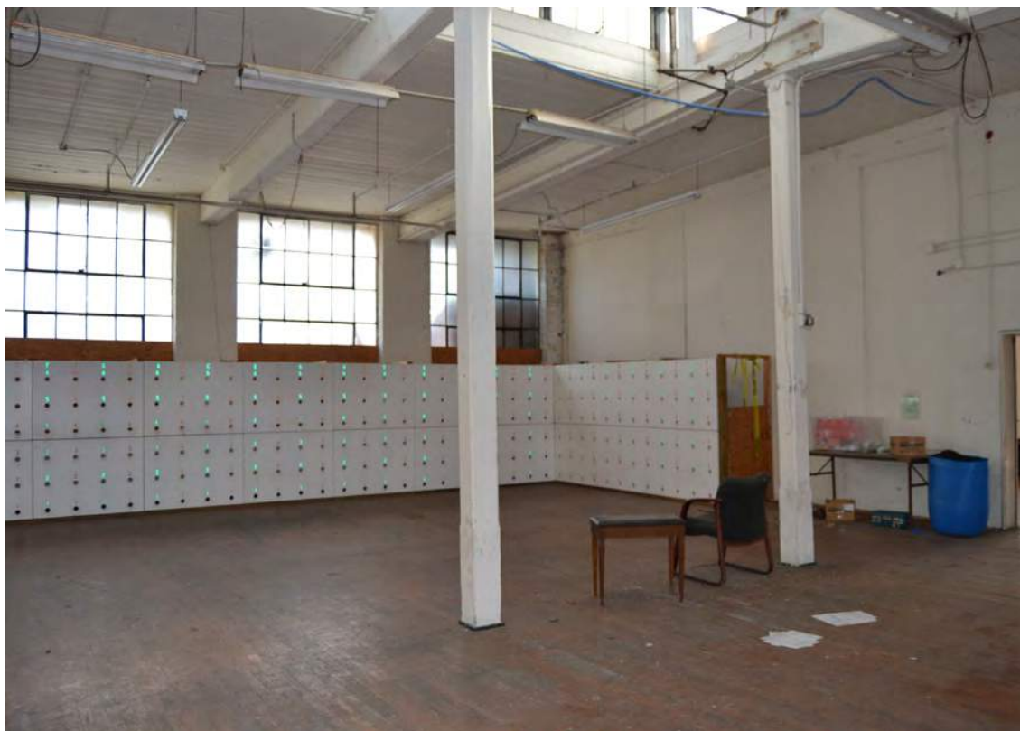
69. Grey Mill, 1926 Addition, Finishing Room, Looking Southeast
