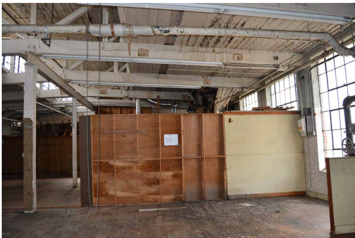
42. Grey Mill, 1915 Building, Looking South
