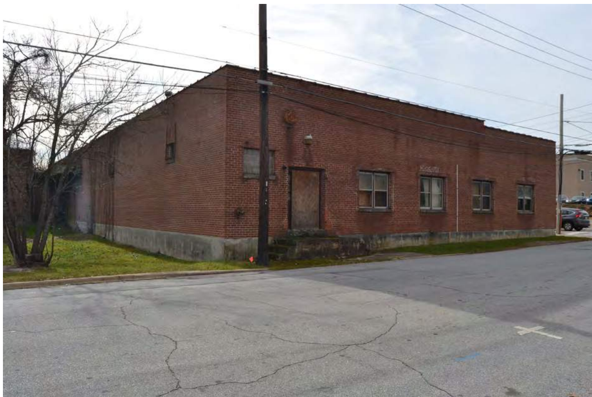
13. Grey Mill, 1947 Addition, North Elevation, Looking Southwest
