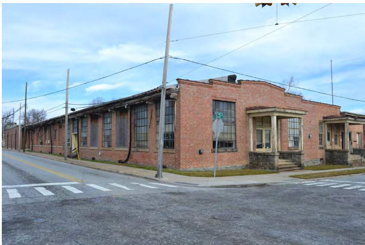
2. Grey Mill, 1915 Building, Southwest Corner, Looking Northeast
