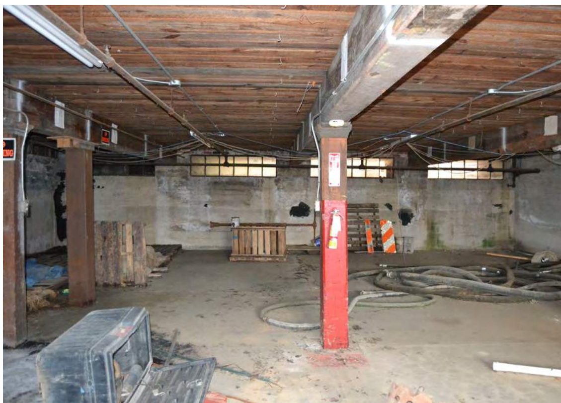
117. Grey Mill, Dye House Basement, Looking West
