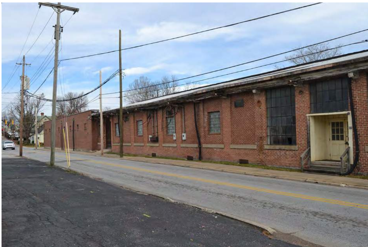
9. Grey Mill, 1915 Building, West Elevation, Looking Northeast
