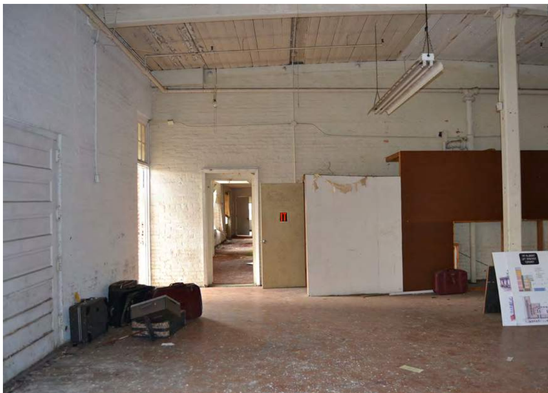
64. Grey Mill, 1919 Building, Looking West
