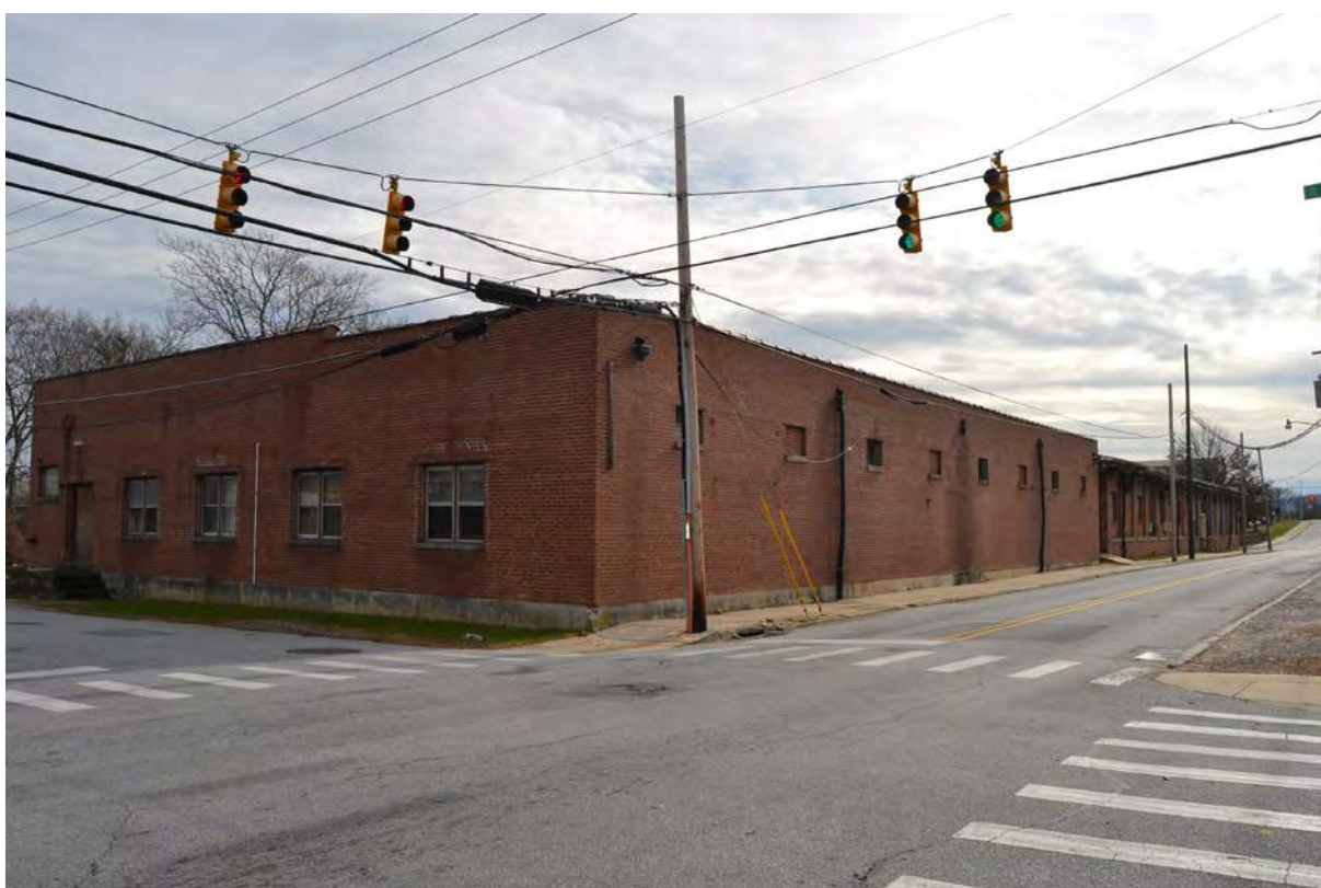
12. Grey Mill, 1947 Addition, Northwest Corner, Looking Southeast
