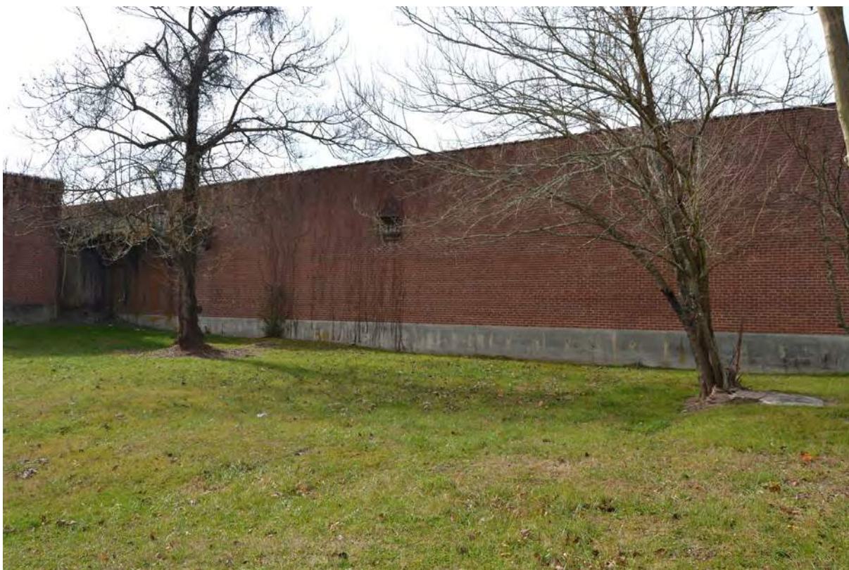
14. Grey Mill, 1947 Addition, North Elevation, Inside Wall, Looking Southwest
