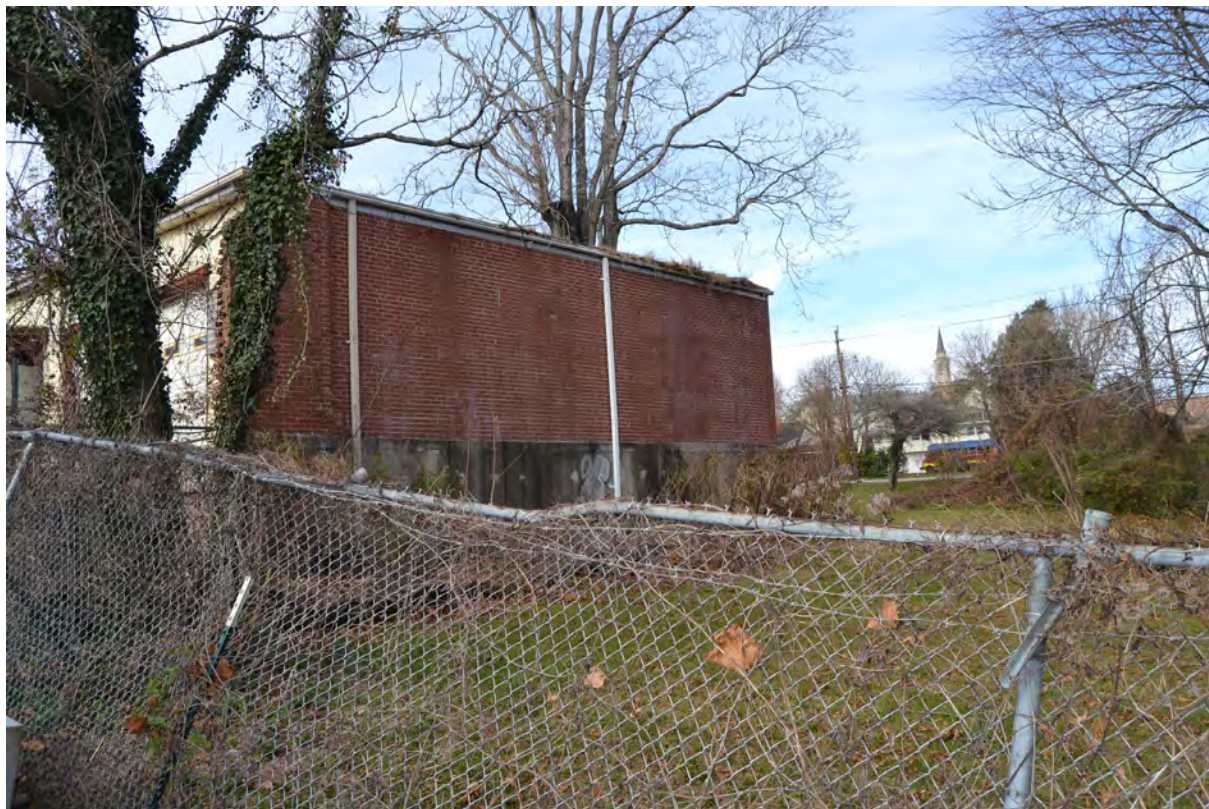
23. Grey Mill, 1970s Warehouse, Looking Northwest
