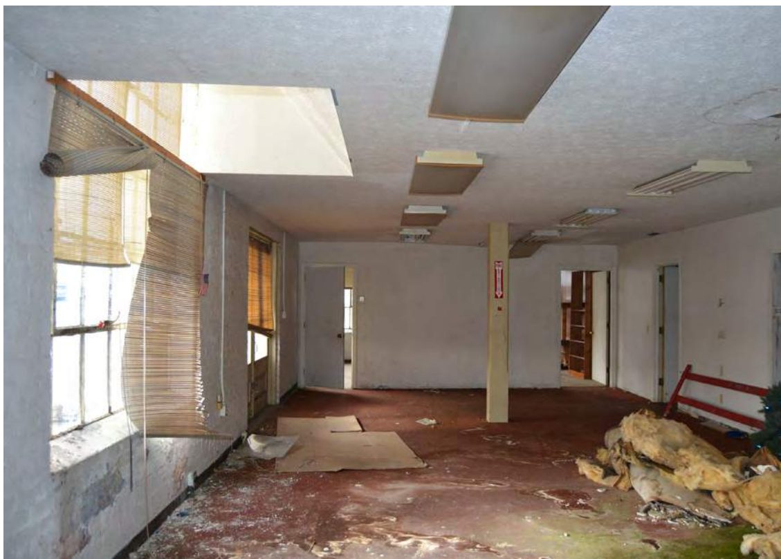
31. Grey Mill, 1915 Building, South End, Looking West
