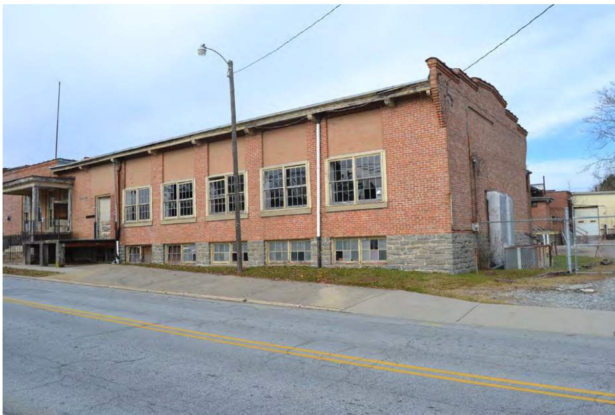
5. Grey Mill, 1919 Building, South Facade, Looking Northwest
