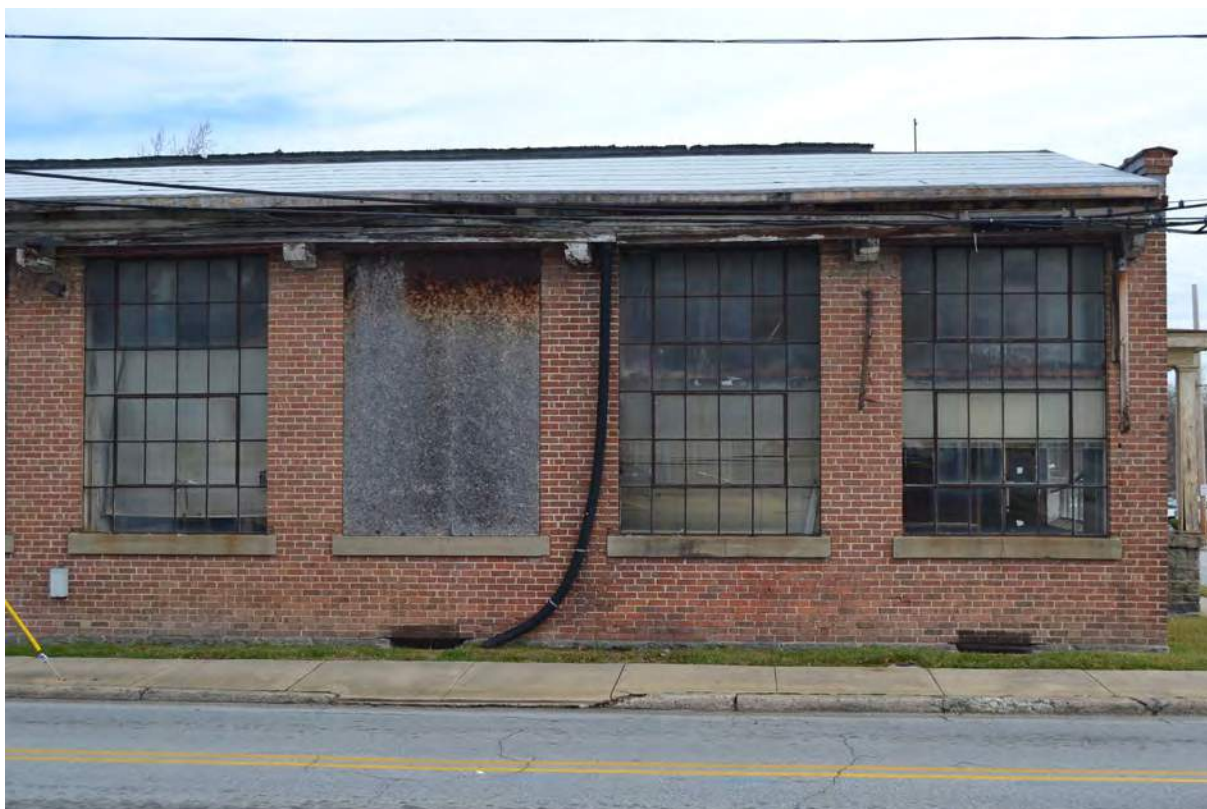
7. Grey Mill, 1915 Building, West Elevation, Window Detail
