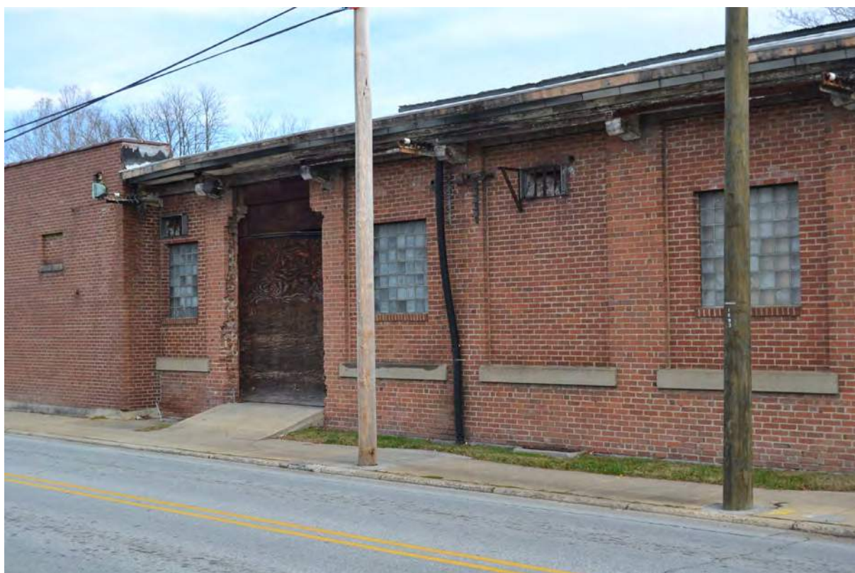
10. Grey Mill, 1915 Building and 1947 Addition, West Elevation, Looking Northeast
