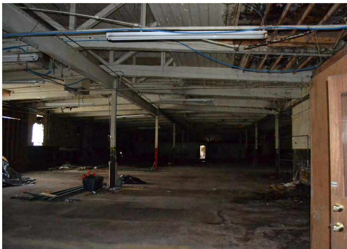
44. Grey Mill, 1947 Addition, Looking North
