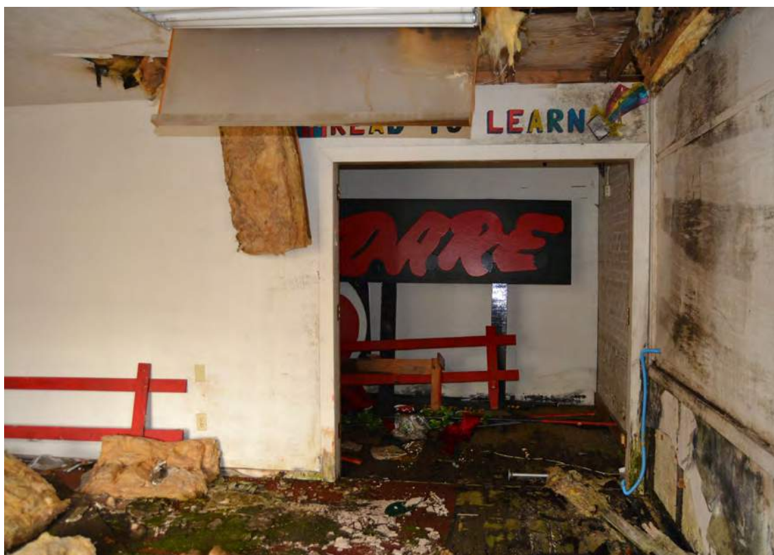
32. Grey Mill, 1915 Building, South End, Looking North
