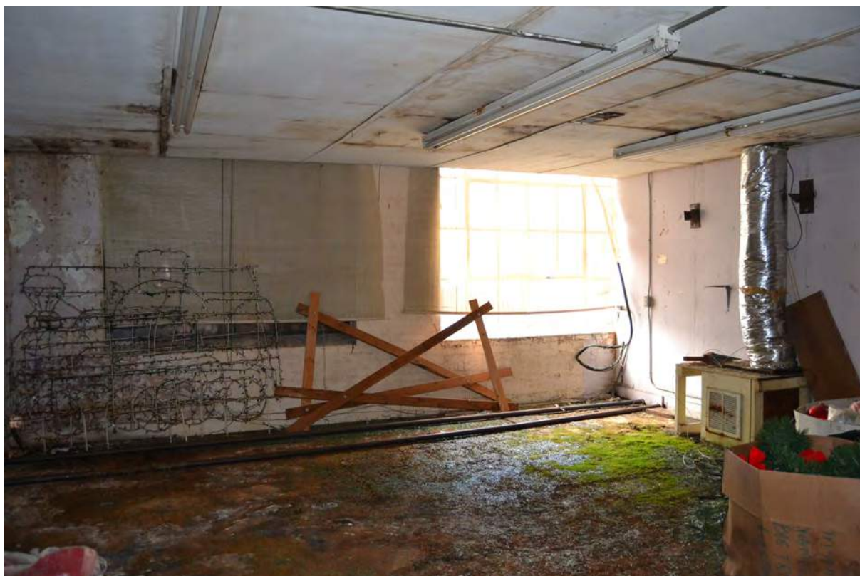
38. Grey Mill, 1915 Building, Looking West
