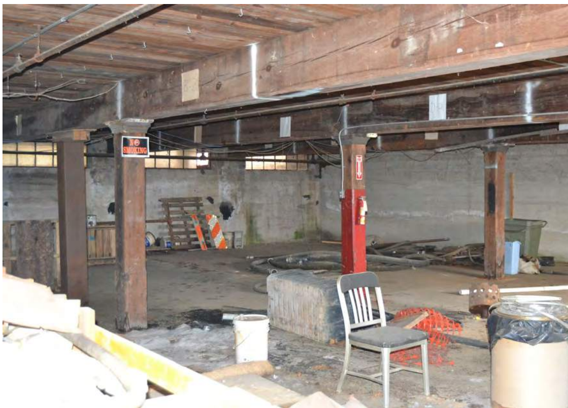
116. Grey Mill, Dye House Basement, Looking Northwest
