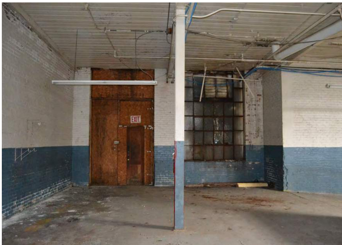
81. Grey Mill, 1926 Addition, Looking East
