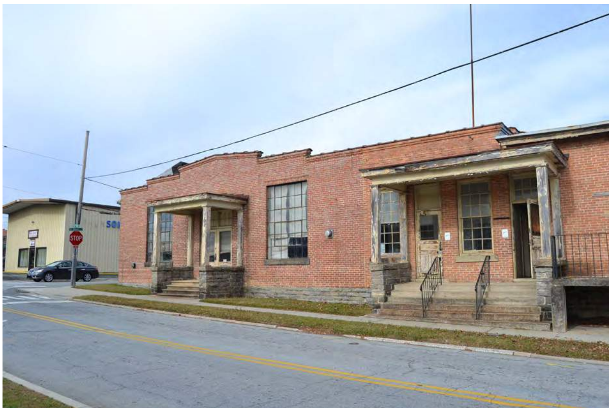
3. Grey Mill, 1915 Building, South Facade, Looking Northwest
