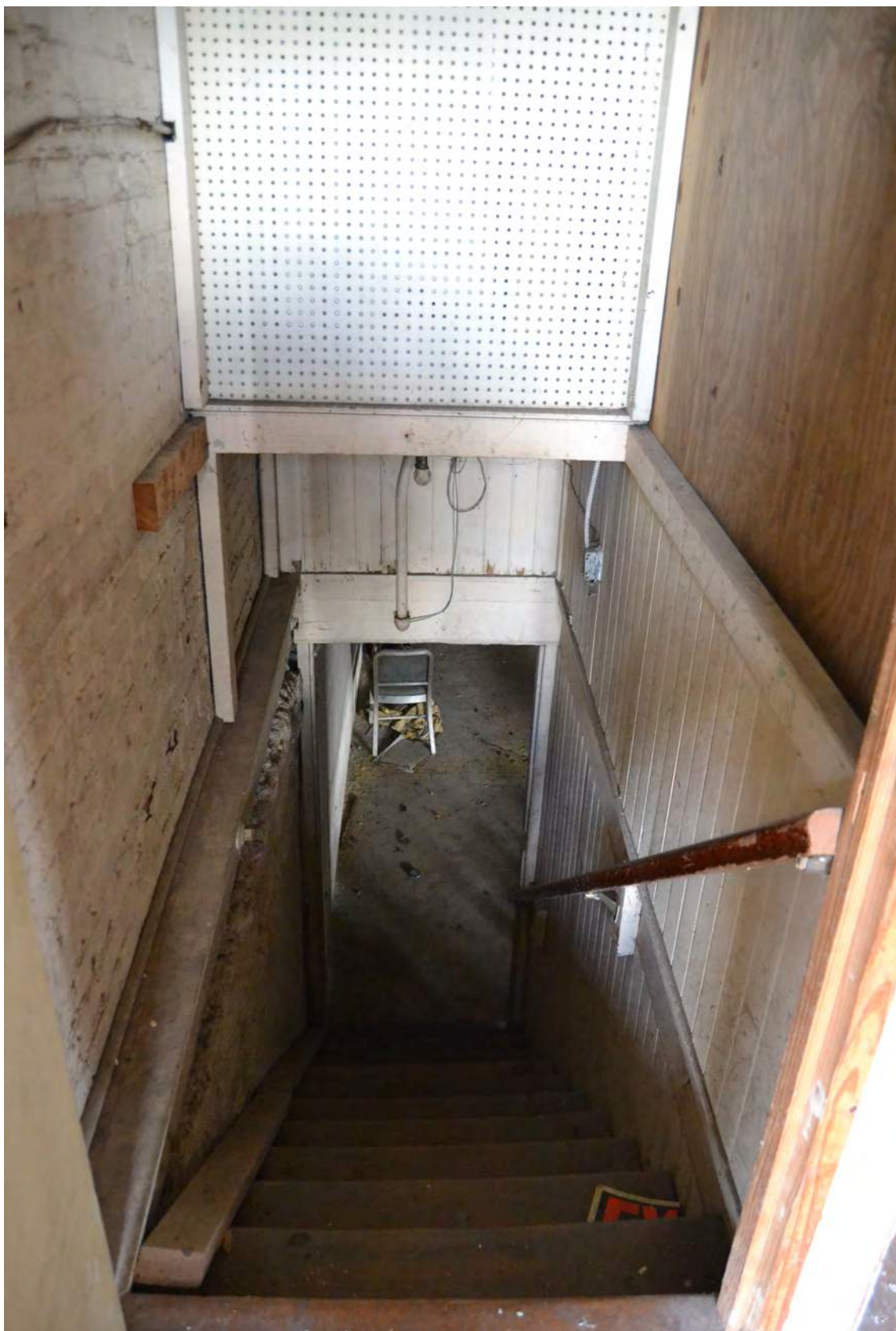
105. Grey Mill, Entrance to Basement, Looking North
