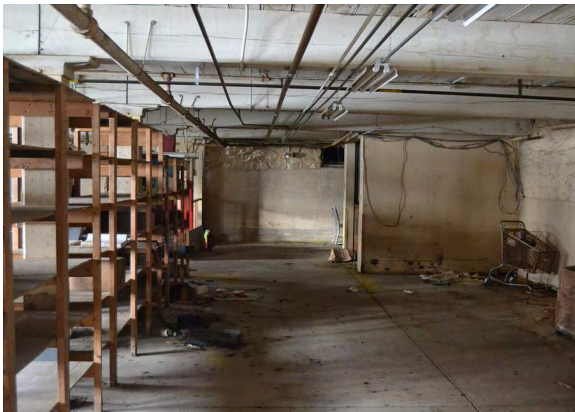
111. Grey Mill, Shipping and Storage Warehouse, Looking West
