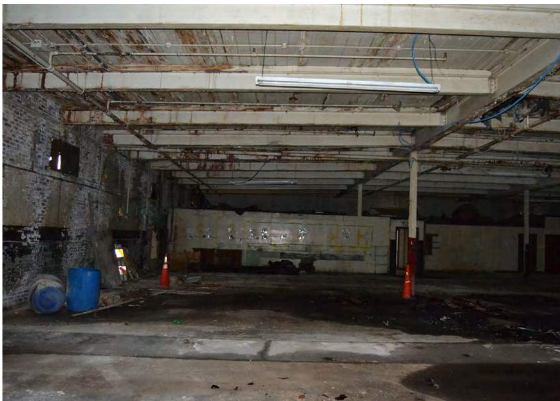
47. Grey Mill, 1947 Addition, Looking North
