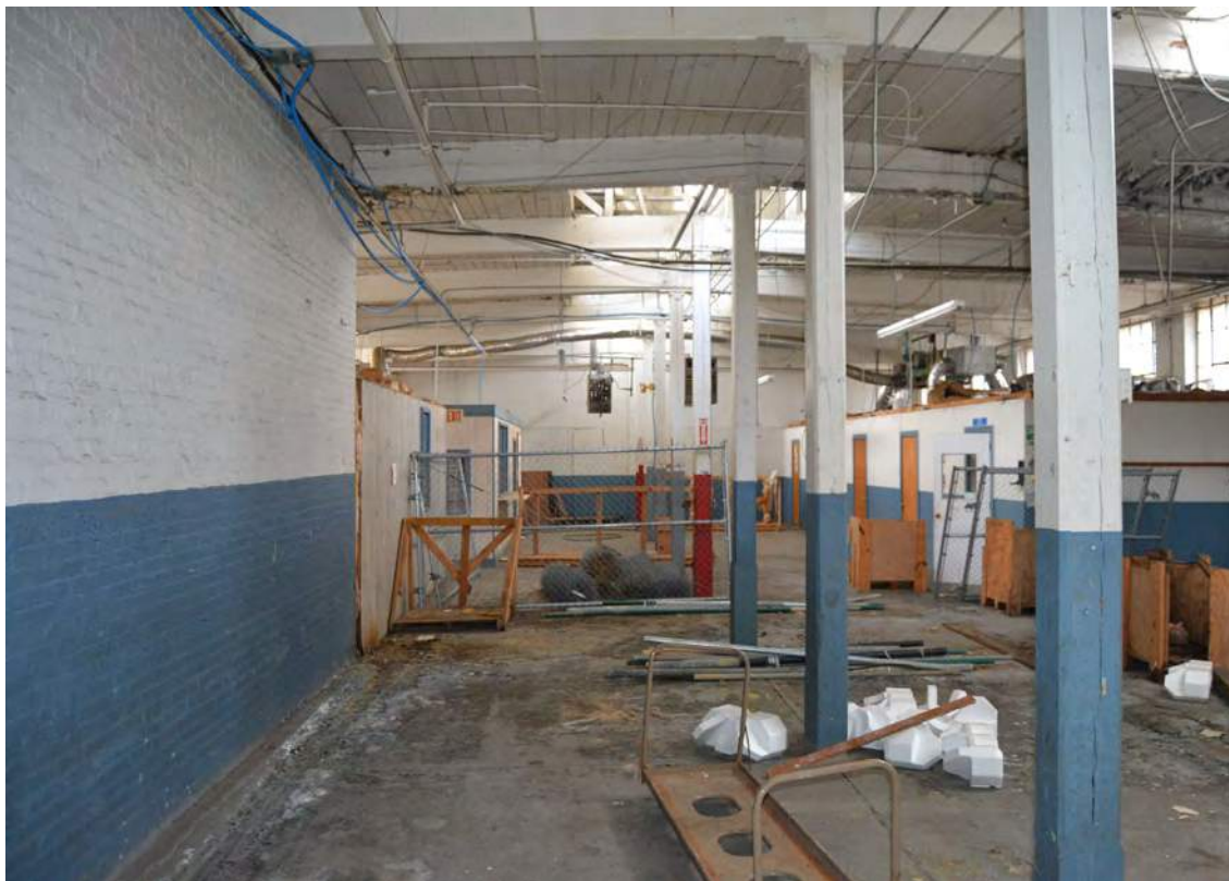
82. Grey Mill, 1926 Addition, Looking South
