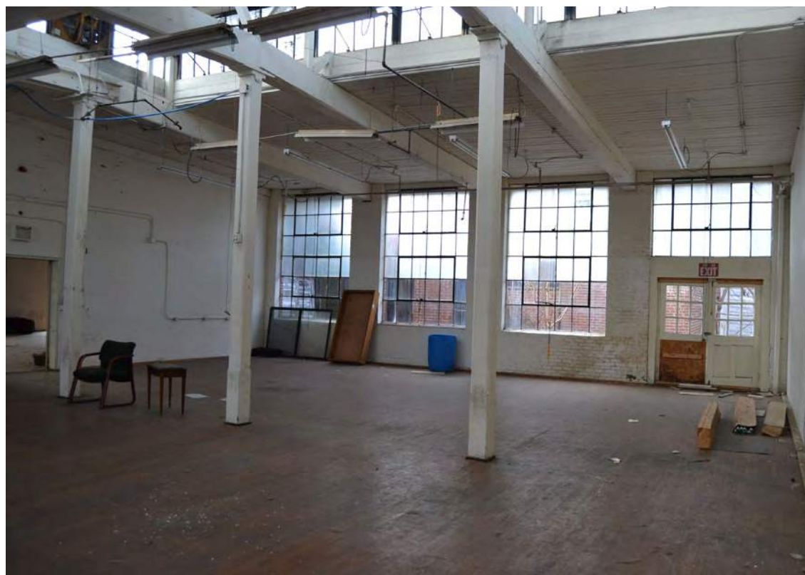
70. Grey Mill, 1926 Addition, Finishing Room, Looking Southwest
