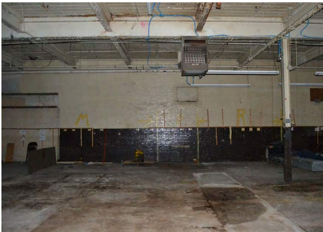
49. Grey Mill, 1947 Addition, Looking East
