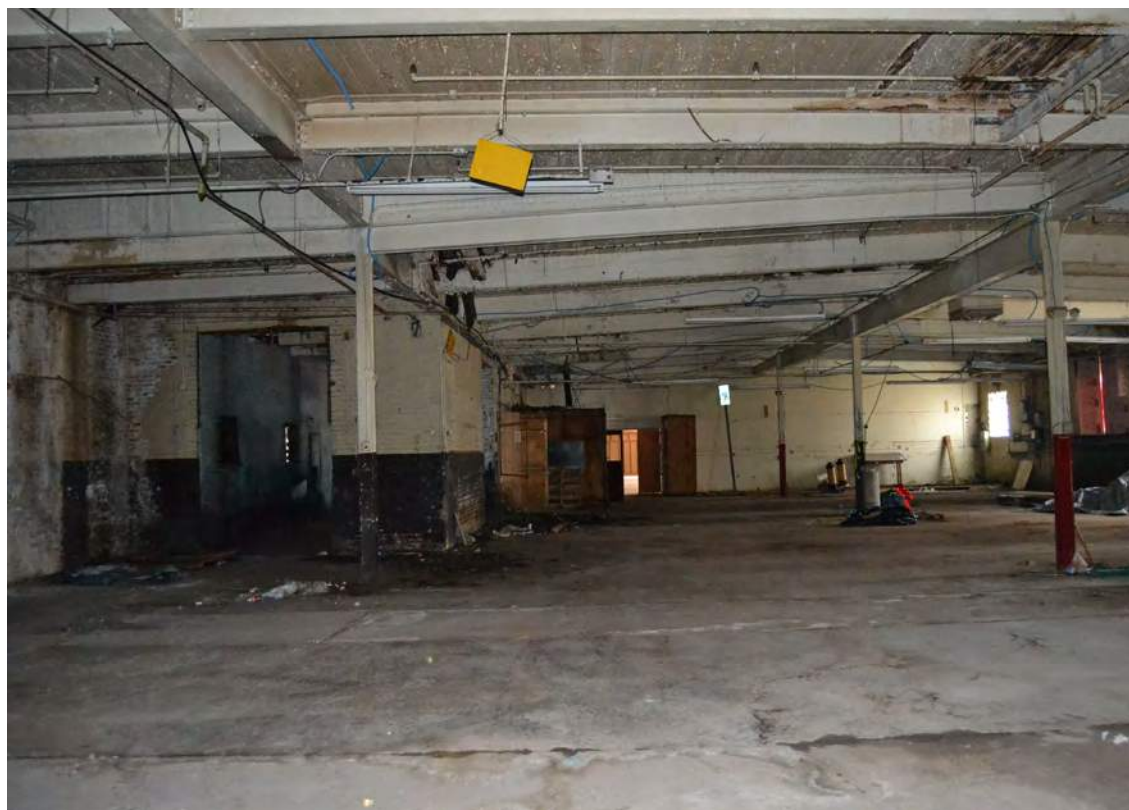
52. Grey Mill, 1947 Addition, Looking South
