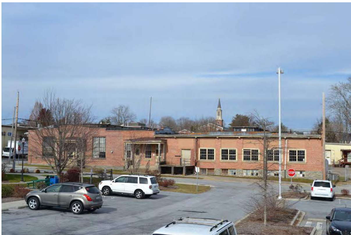
1. Grey Mill, South Facade, Looking North
