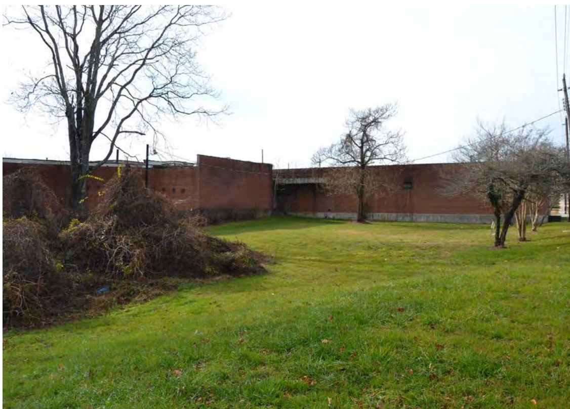
16. Grey Mill, 1947 Addition, North Elevation, Looking West
