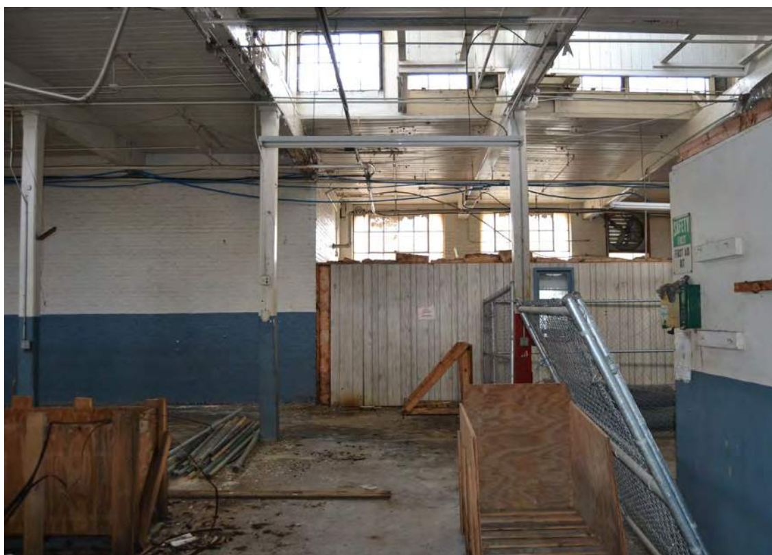
78. Grey Mill, 1926 Addition, Drying Room, Looking East
