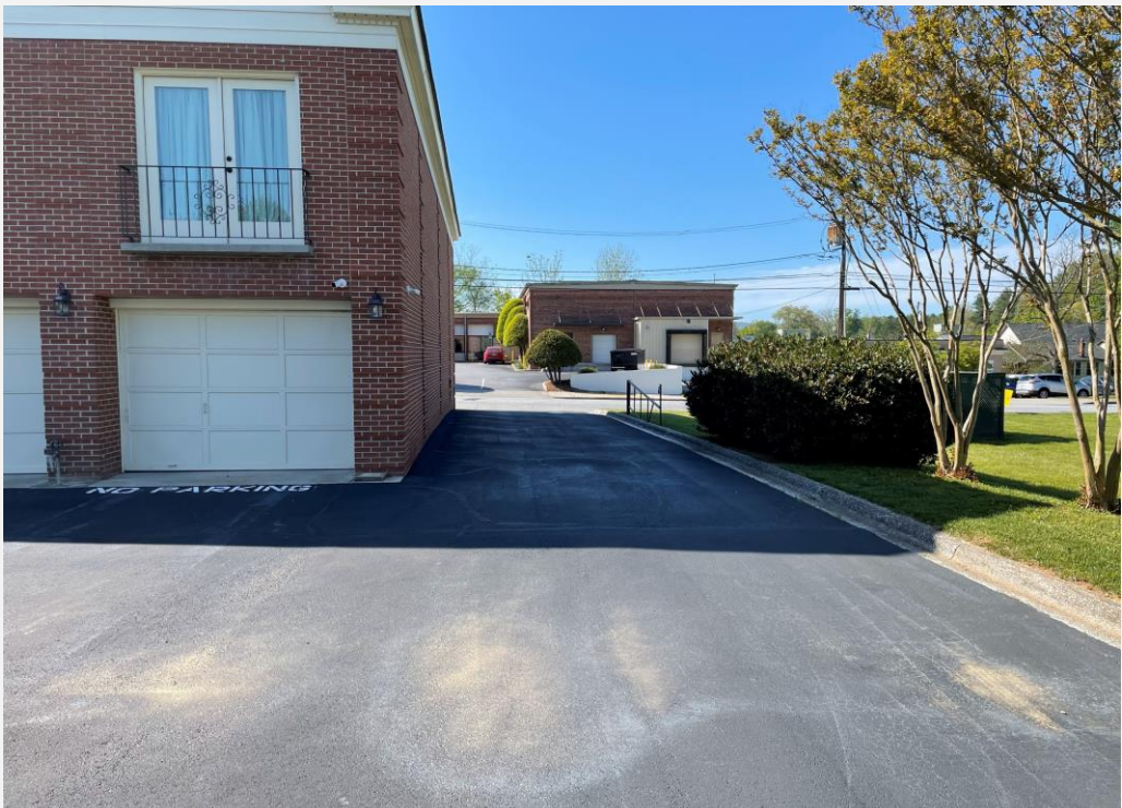
View of the existing rear access from W. Allen where the new parking lot will tie into.
