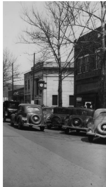
brick sills. Front
