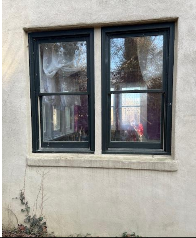
Exterior photo of windows proposed to be replaced with double doors.
