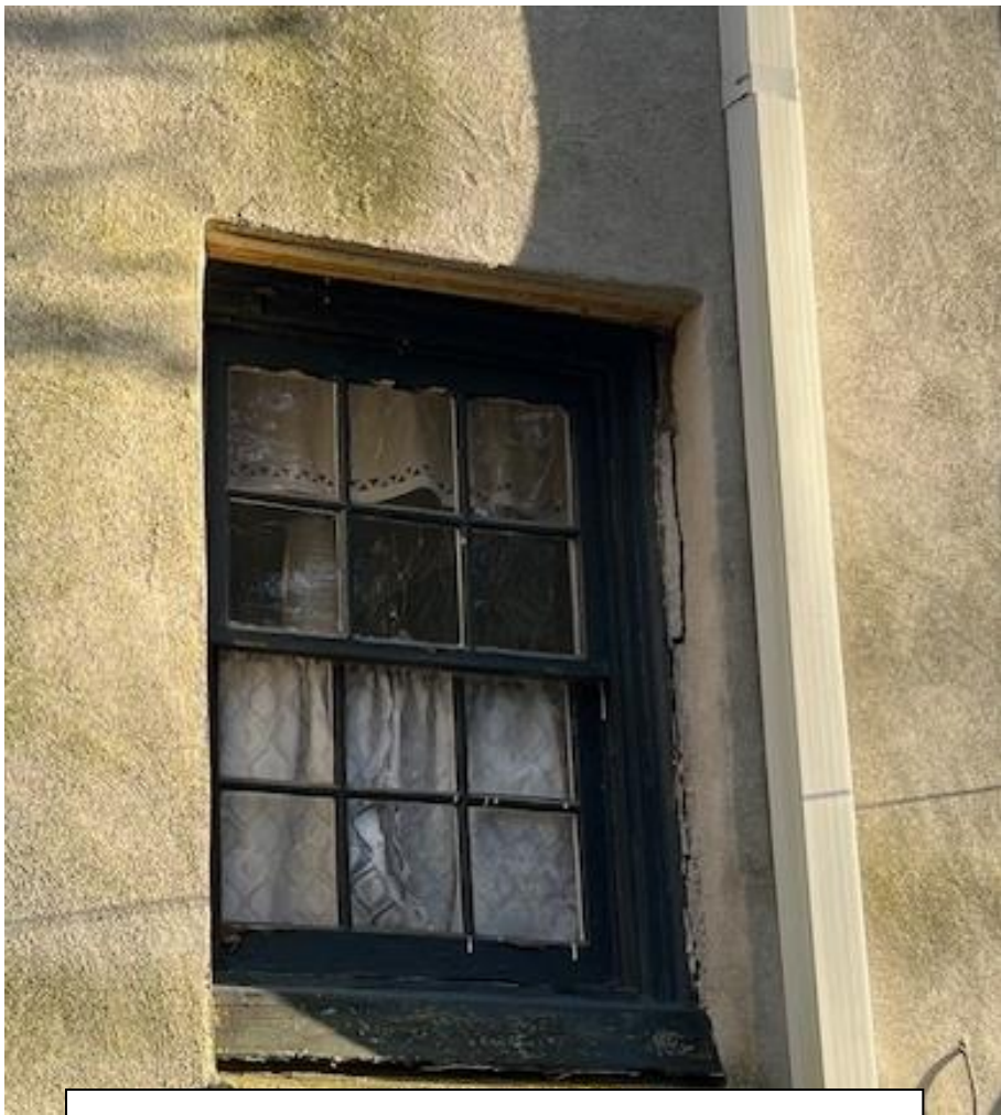
Exterior view of existing kitchen windows.
