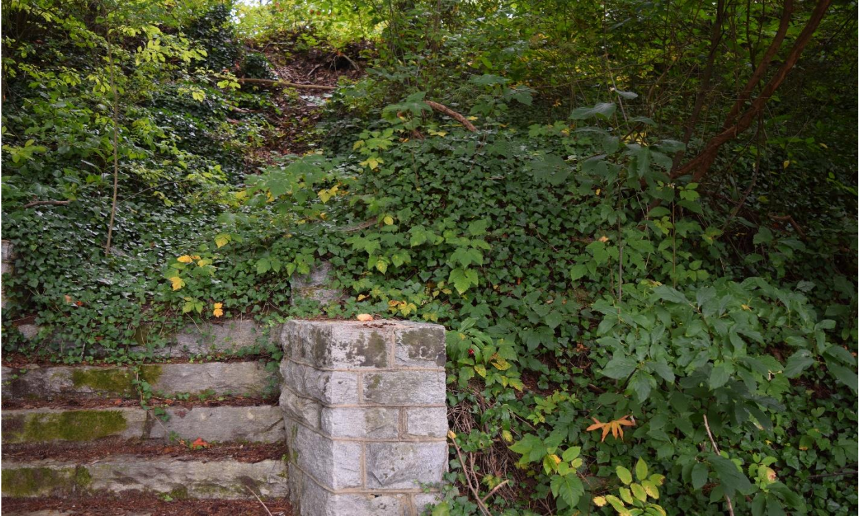
14. Staircase as rear of spring, view northwest
