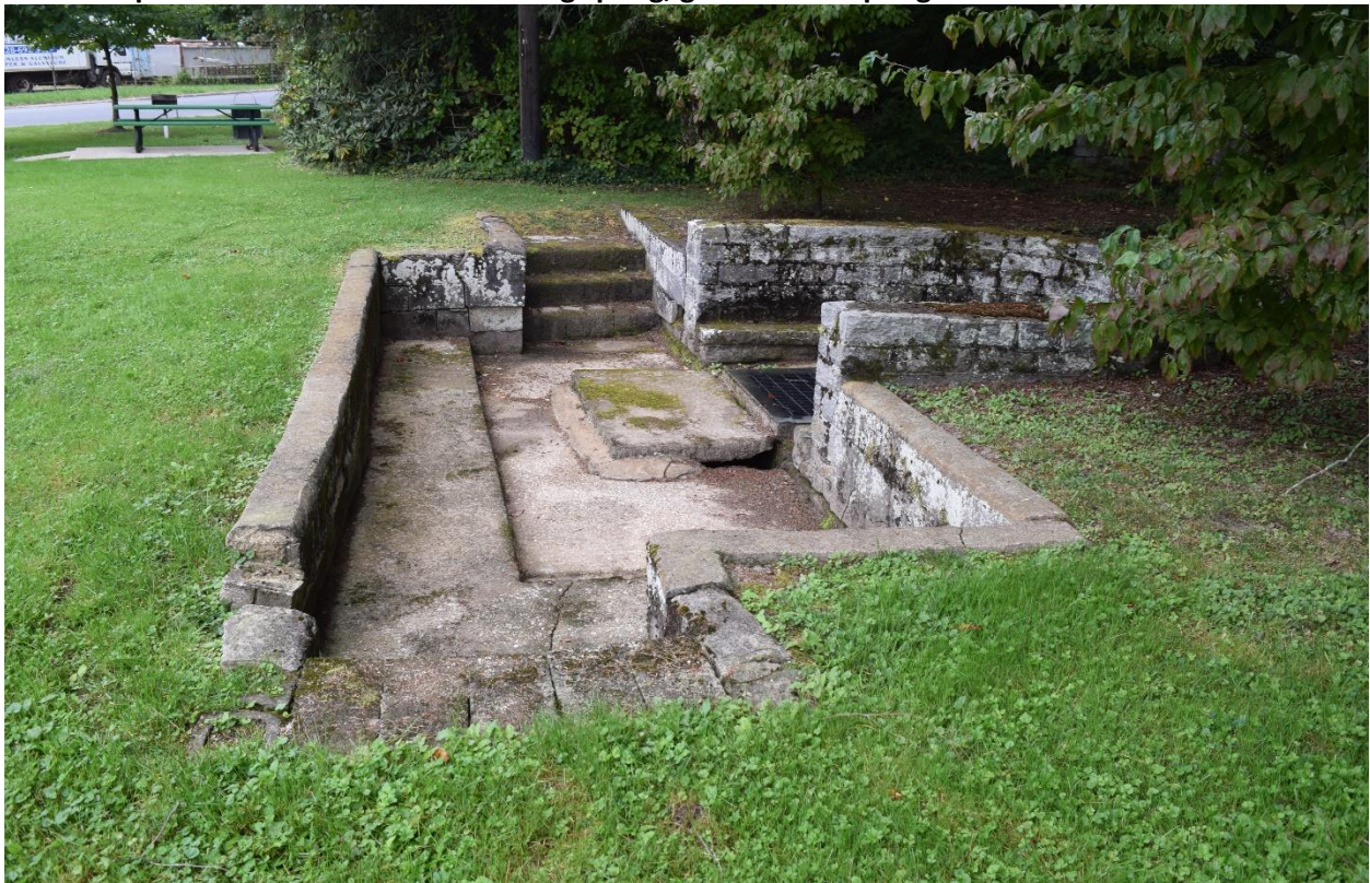
8. Lenox Spring stonework, view southeast
