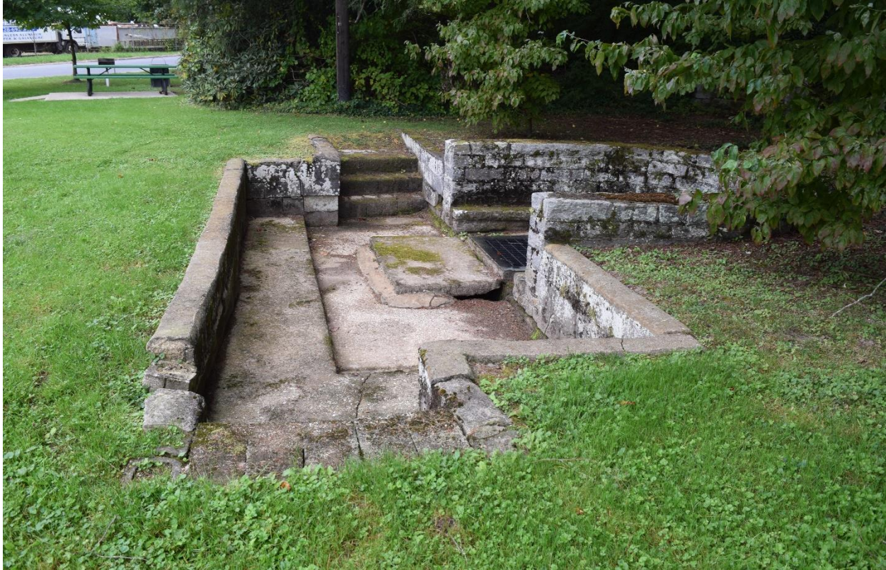
8. Lenox Spring stonework, view southeast
