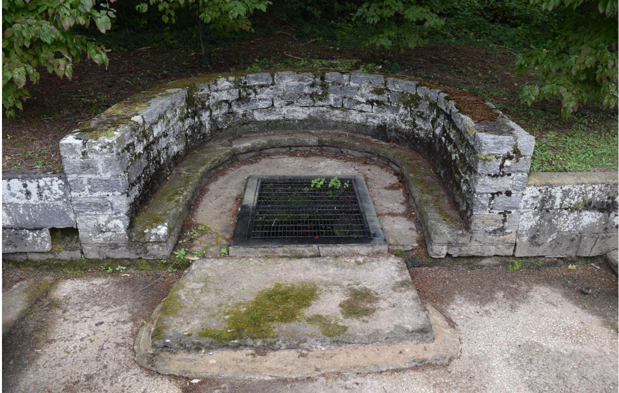
7. Close-up view of stonework surrounding spring, grate covers spring
