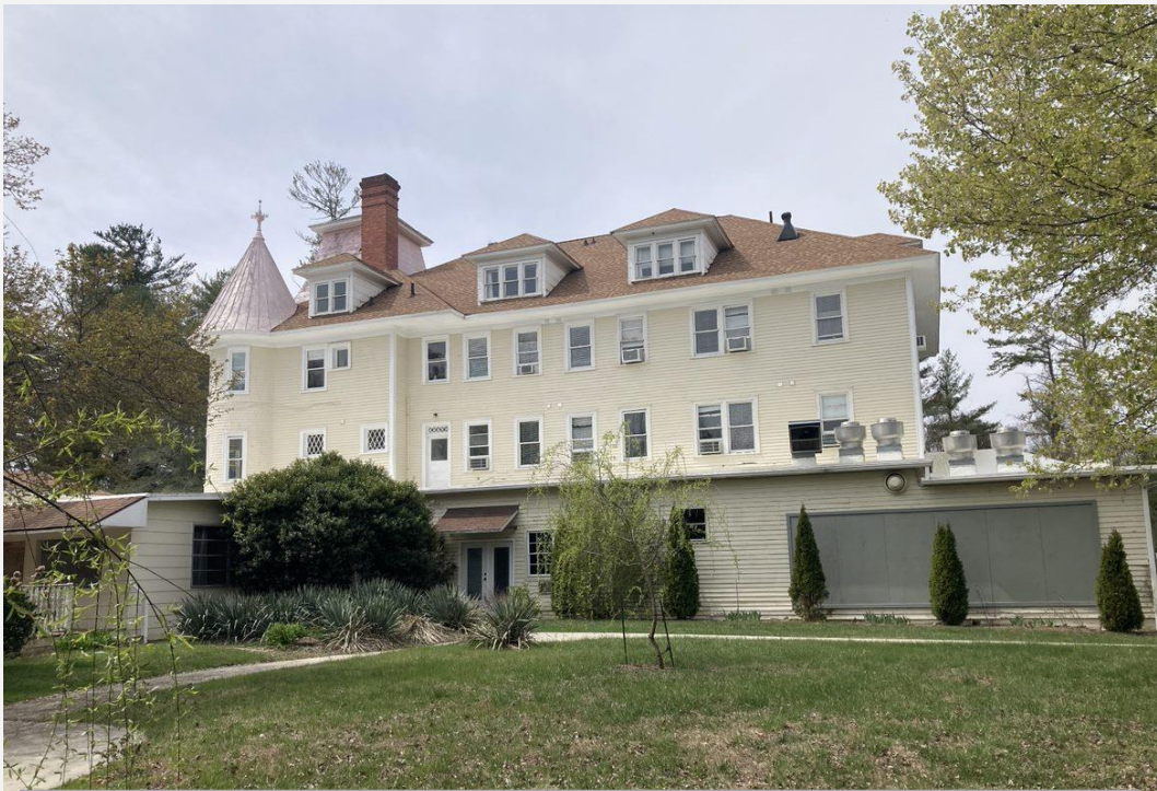
View of east side of principal structure from interior courtyard (facing west)
