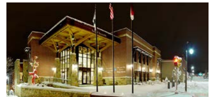
Waynesville Government Center Waynesville, North Carolina
