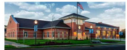
Wingate Government Center Wingate, North Carolina
