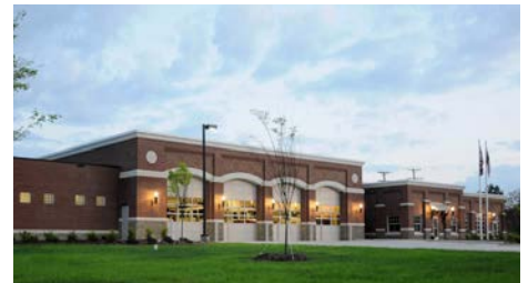
Concord Fire Station No. 9 Concord, North Carolina
