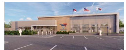
Cabarrus County EMS Headquarters Concord, North Carolina
