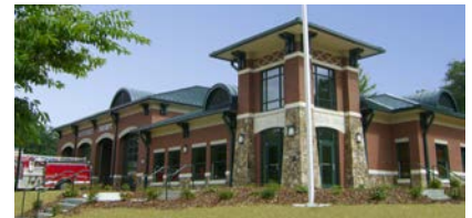
Waynesville Fire Station No. 1 Waynesville, North Carolina
