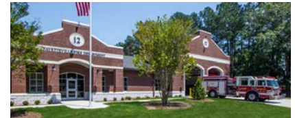
Fayetteville Fire Station No. 12 Fayetteville, North Carolina
