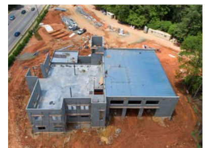
Cary Fire Station No. 9
