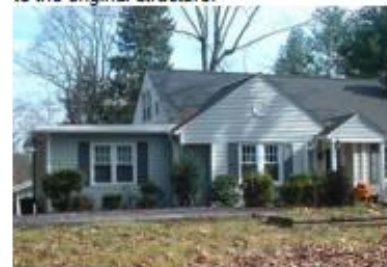
The addition on this home would have been more successful with a roofline that related to the original structure.
