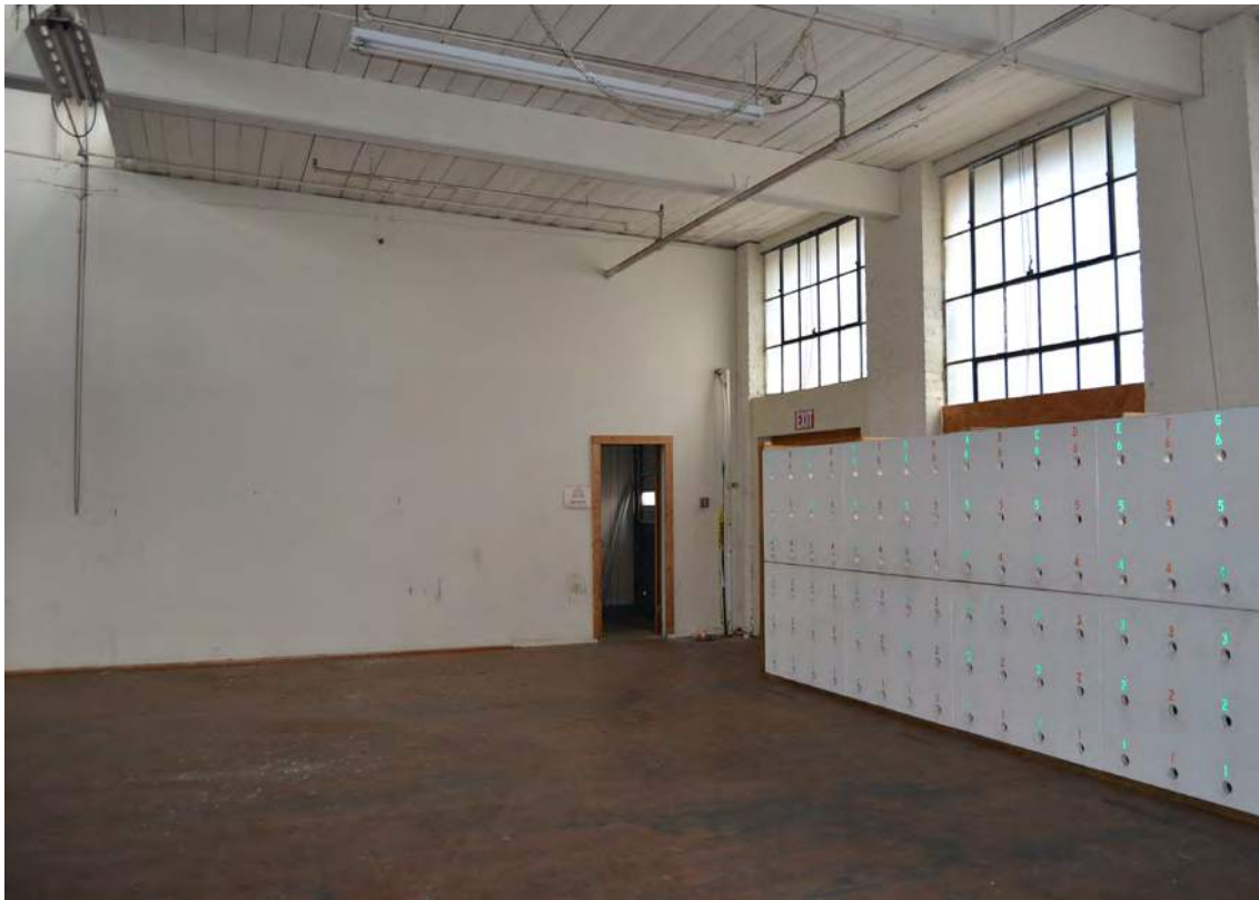
67. Grey Mill, 1926 Addition, Finishing Room, Looking Northeast
