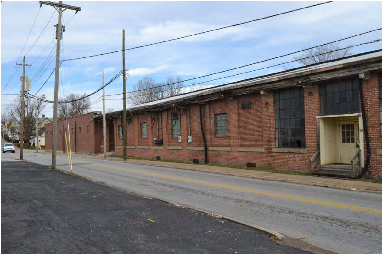
9. Grey Mill, 1915 Building, West Elevation, Looking Northeast
