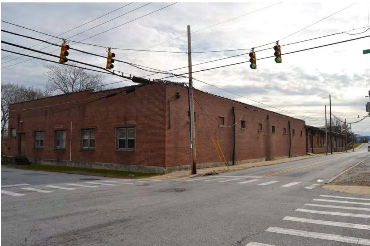
12. Grey Mill, 1947 Addition, Northwest Corner, Looking Southeast
