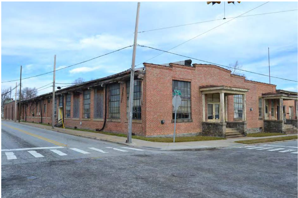
2. Grey Mill, 1915 Building, Southwest Corner, Looking Northeast
