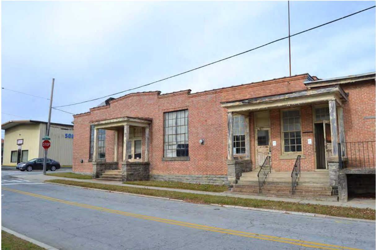
3. Grey Mill, 1915 Building, South Facade, Looking Northwest
