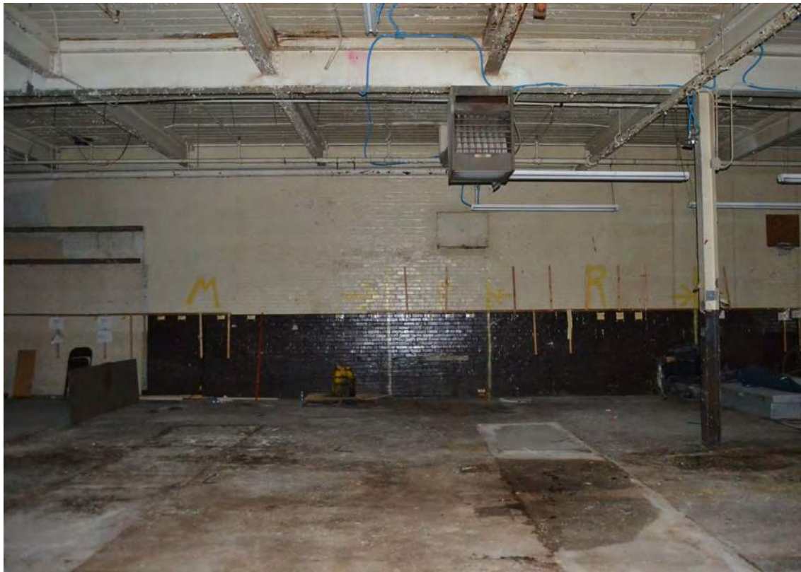
49. Grey Mill, 1947 Addition, Looking East
