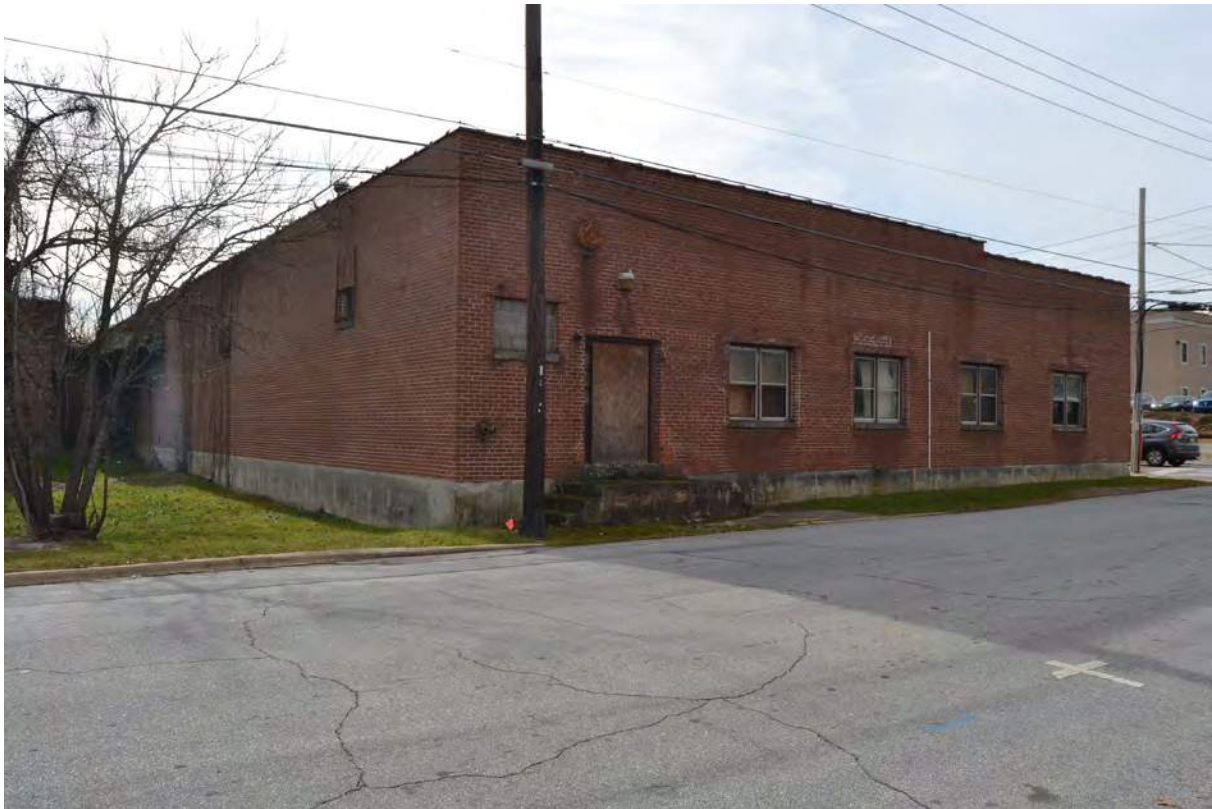
13. Grey Mill, 1947 Addition, North Elevation, Looking Southwest
