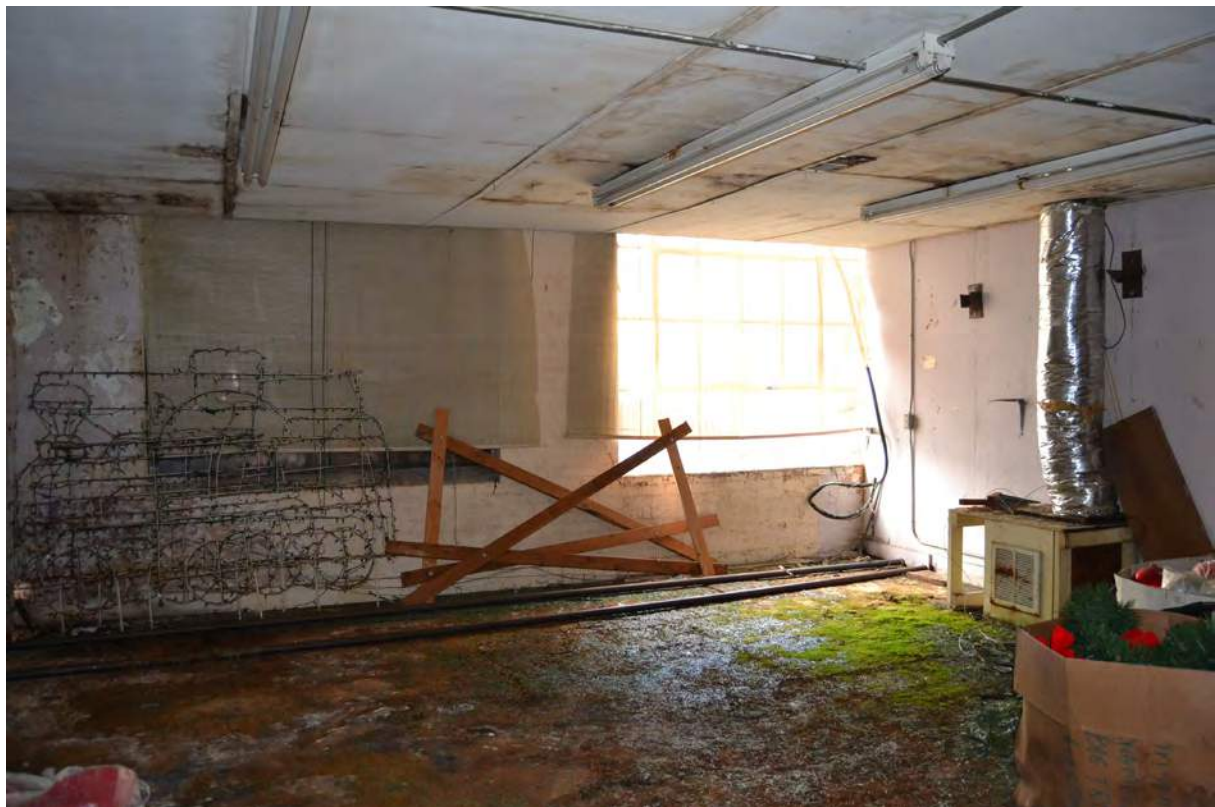
38. Grey Mill, 1915 Building, Looking West
