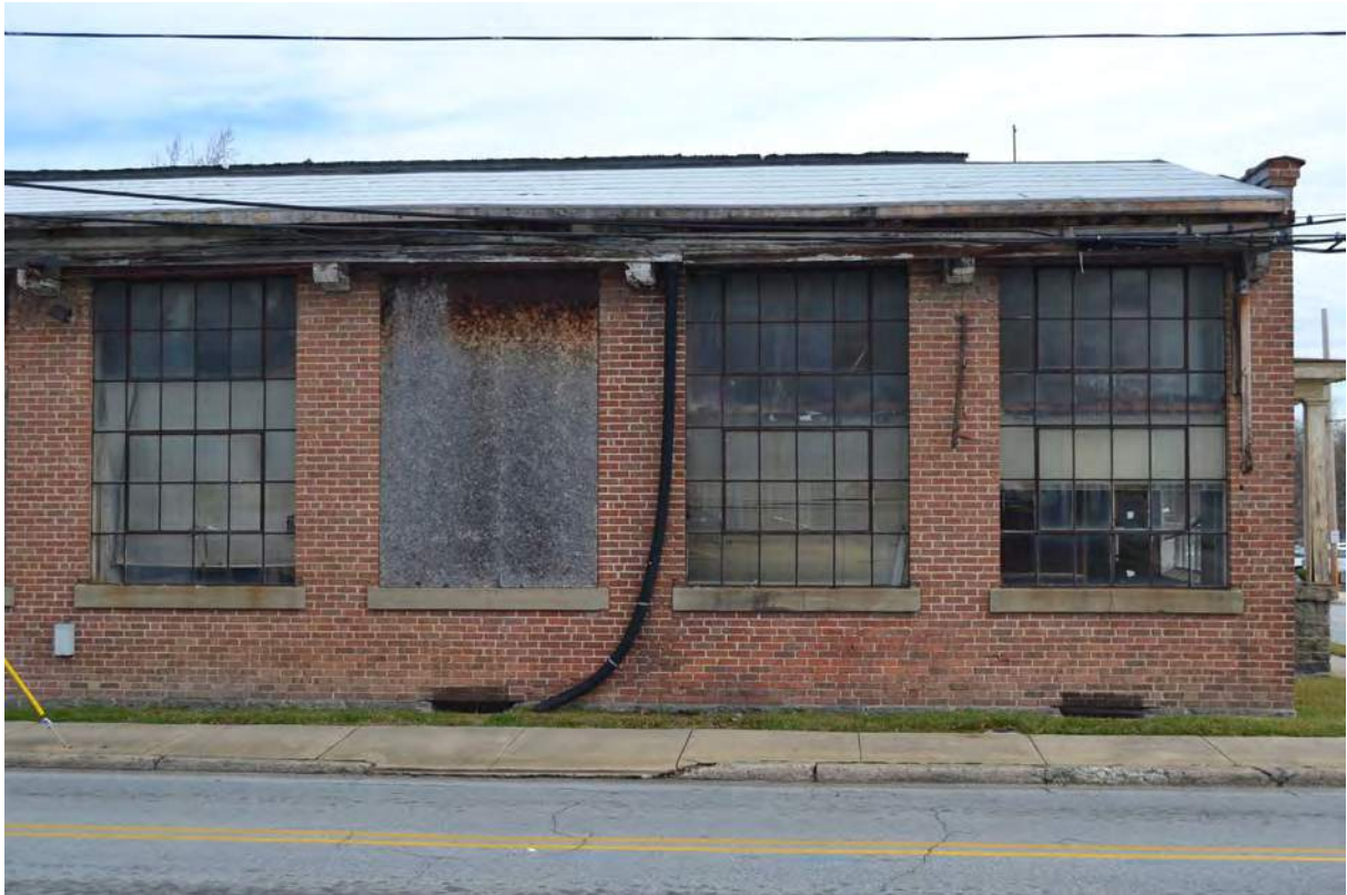
7. Grey Mill, 1915 Building, West Elevation, Window Detail
