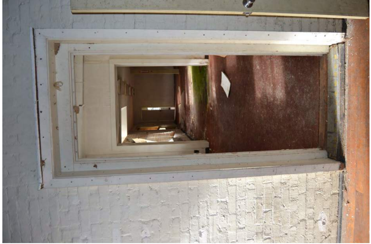
27. Grey Mill, 1919 Building to Office, Looking West
