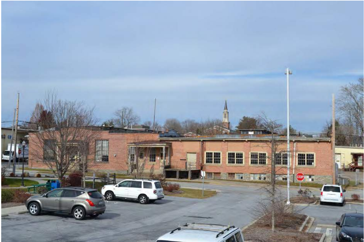
1. Grey Mill, South Facade, Looking North
