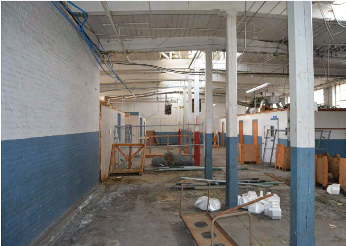
82. Grey Mill, 1926 Addition, Looking South
