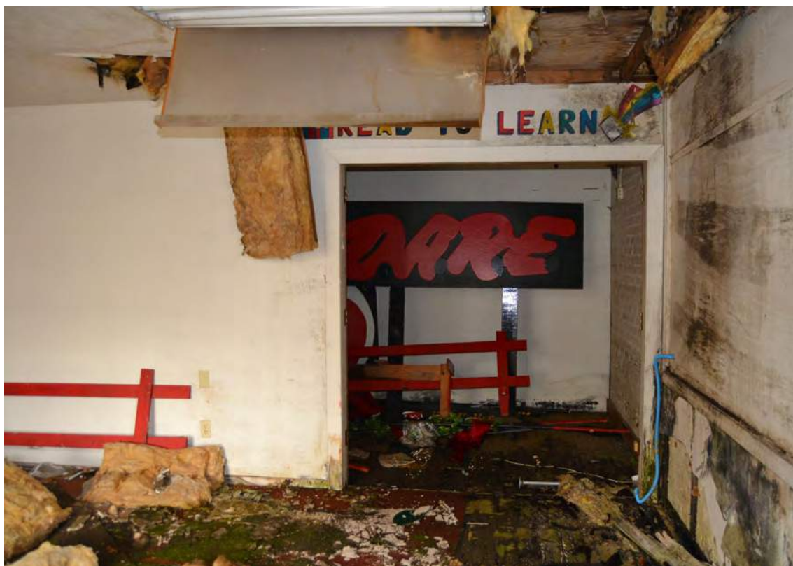
32. Grey Mill, 1915 Building, South End, Looking North
