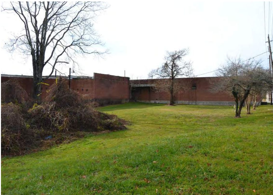
16. Grey Mill, 1947 Addition, North Elevation, Looking West
