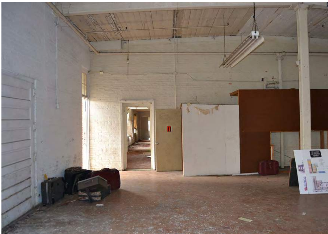
64. Grey Mill, 1919 Building, Looking West
