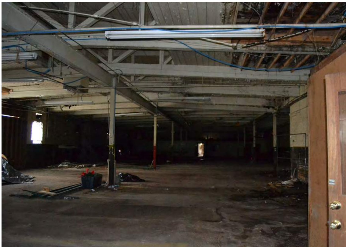
44. Grey Mill, 1947 Addition, Looking North
