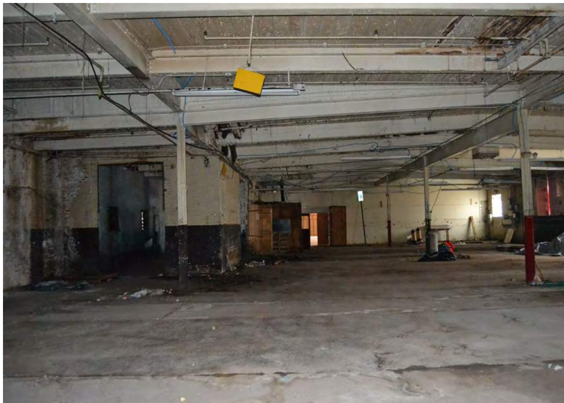
52. Grey Mill, 1947 Addition, Looking South
