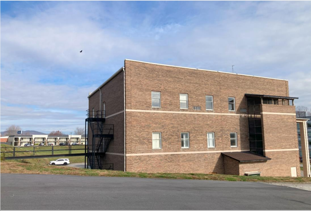
View of subject property from southern boundary facing north
