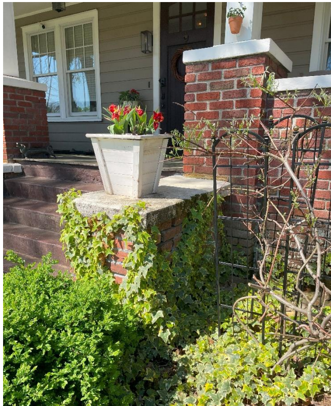
Right wing wall. Mortar has significantly eroded from in between the bricks.
