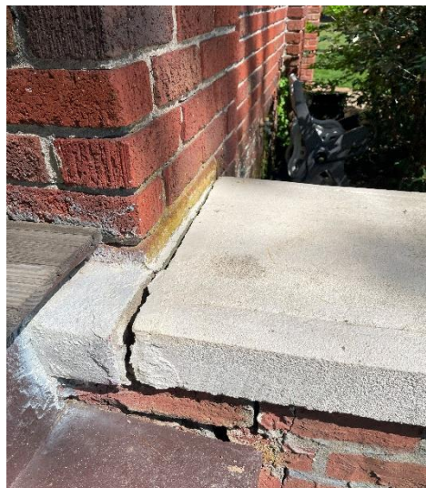
Caps on right wing wall cracked and separated from porch masonry.
