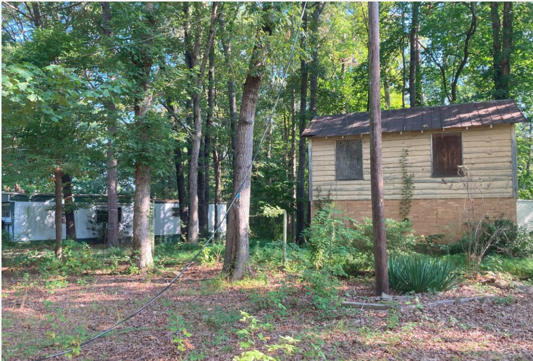
View of existing structures on the site
