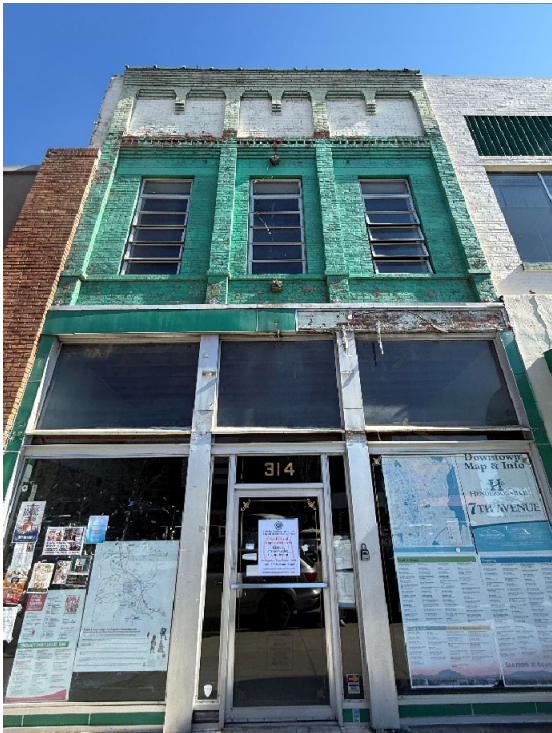
Close up photo of storefront facade
