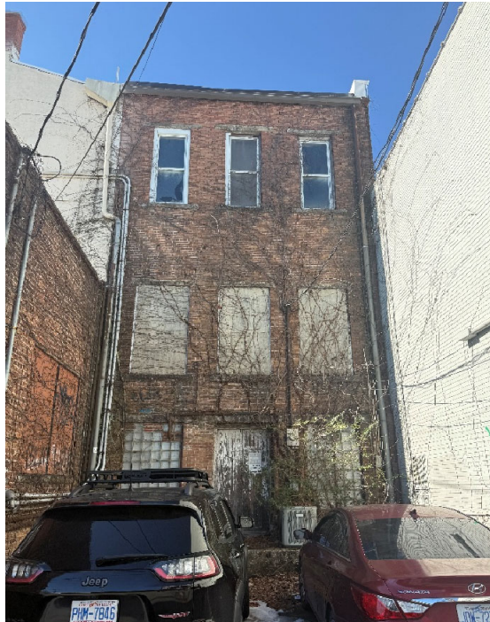
Current rear façade
