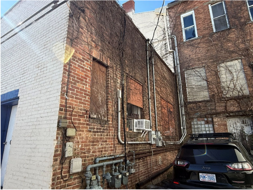
Neighboring building stairwell addition will border
