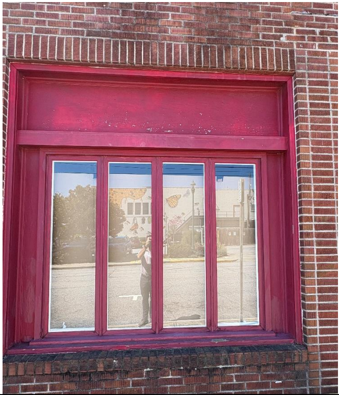
Easternmost infilled windows. Proposal will remove entire window and trim unit and replace with aluminum windows.
