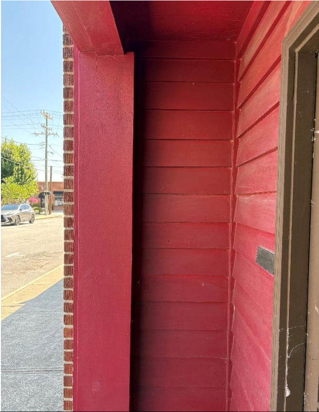
Entryway side wall.
