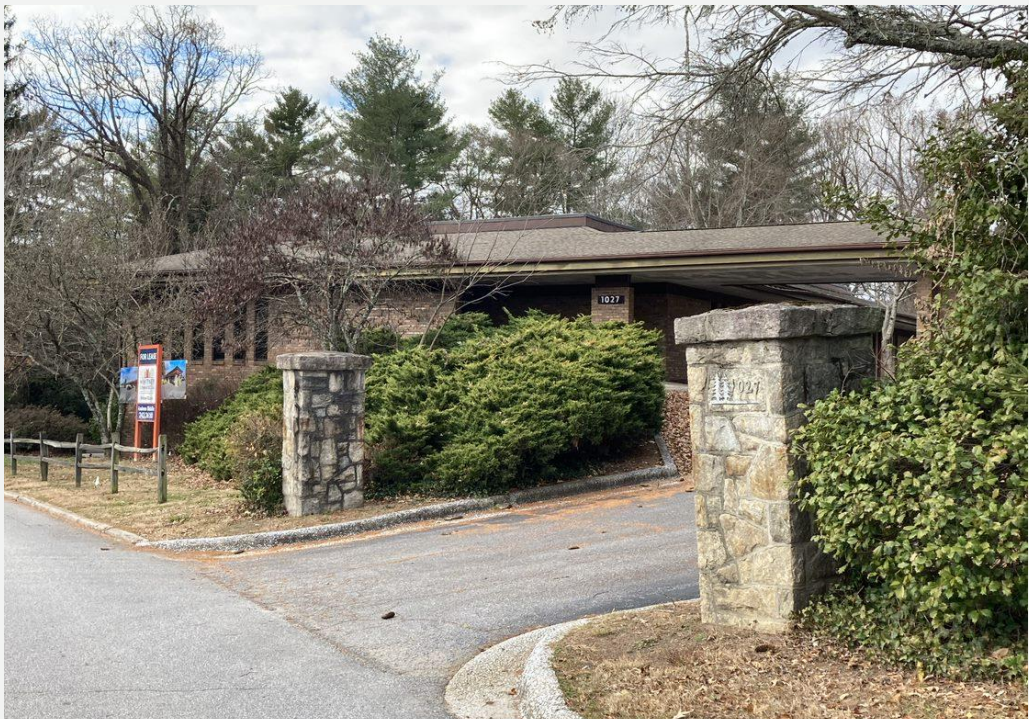
View of 1 of 2 access points to the subject property from Fleming St
