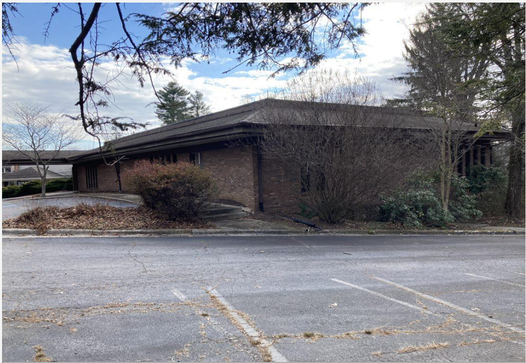
View of rear (west facing) side of the existing building
